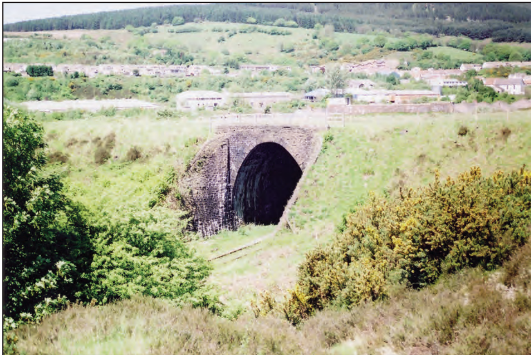
Plate 12 Bridge crossing Llynfi Valley Railway
