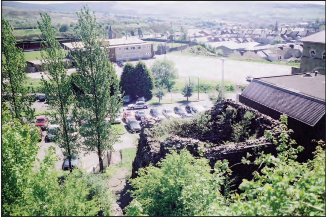
Plate 1 South-western part of the site, with blast furnace in foreground
