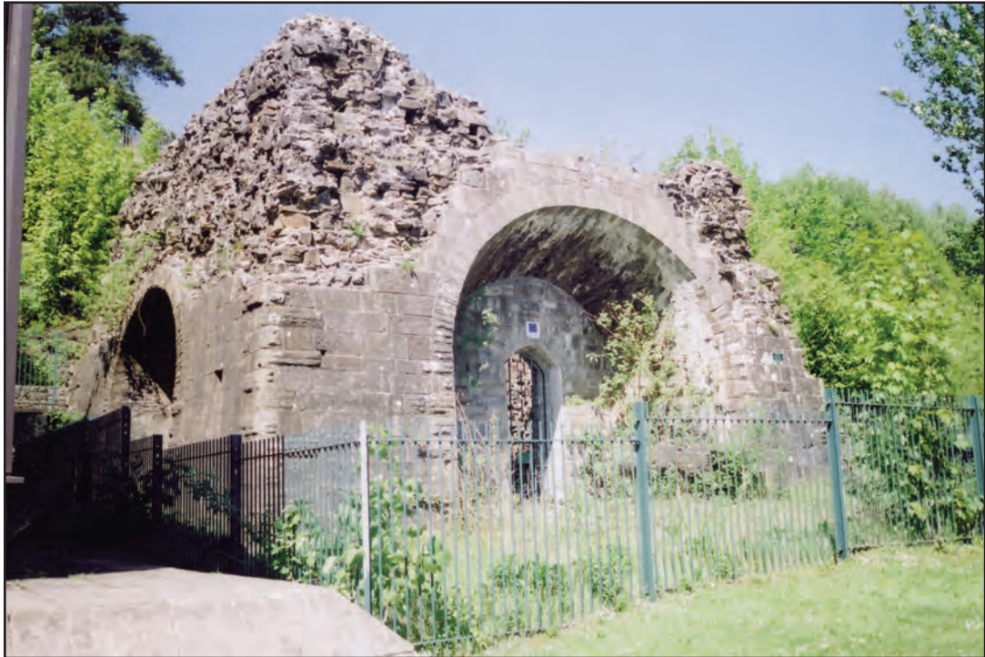
Plate 6 Former No.1 blast furnace
