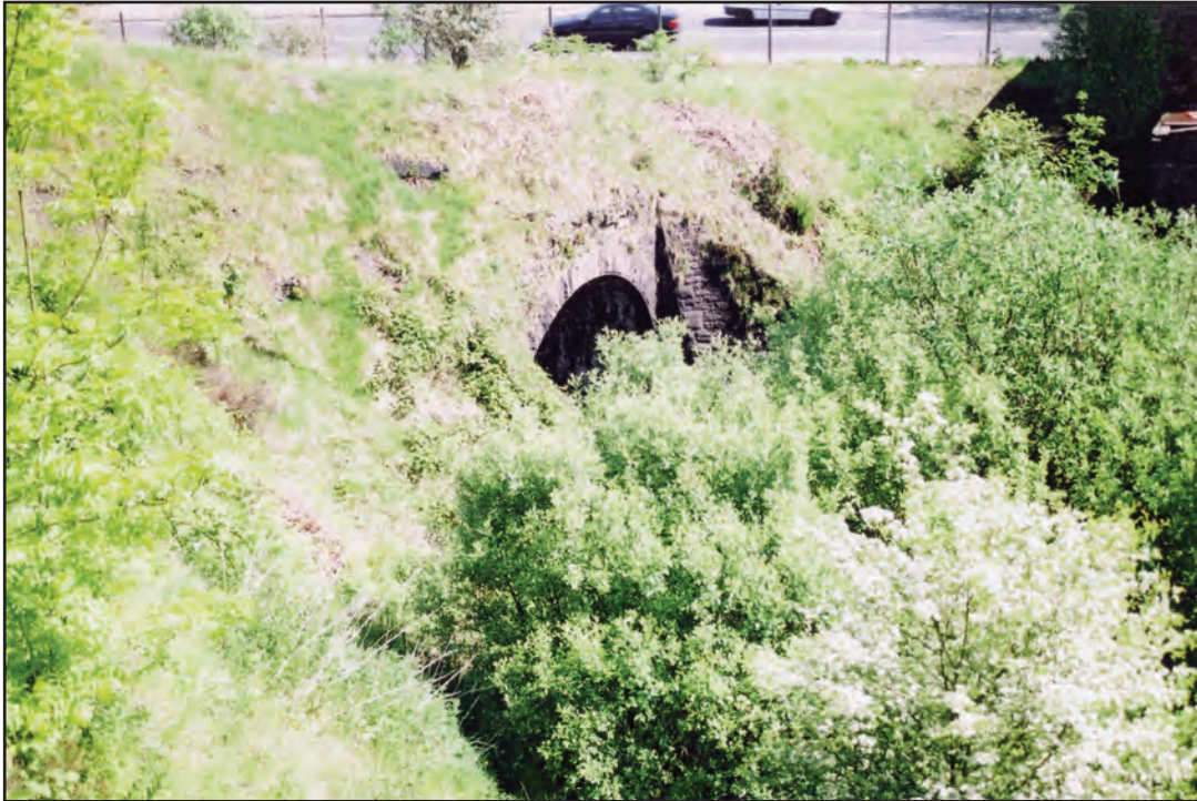
Plate 8 Southern end of Llynfi River culvert
