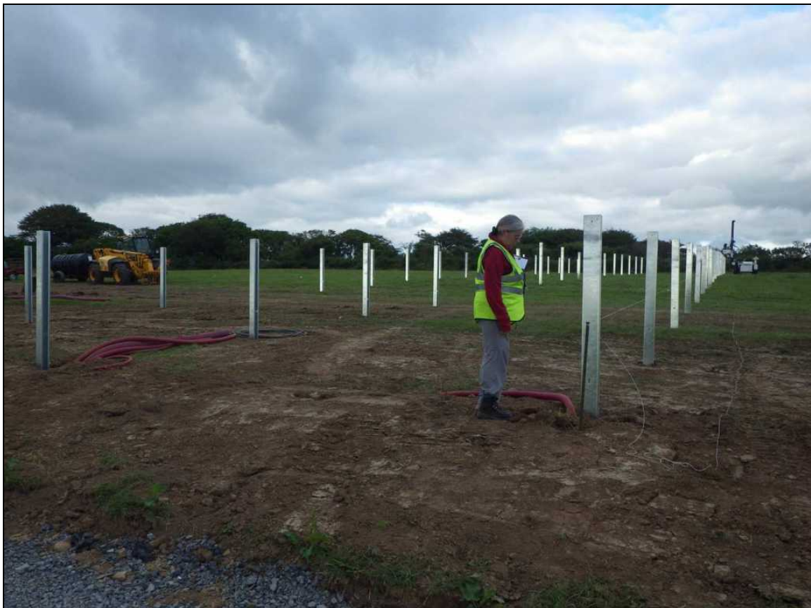
Plate 14: PFL2014_114, supporting posts erected ready to receive the panels.
