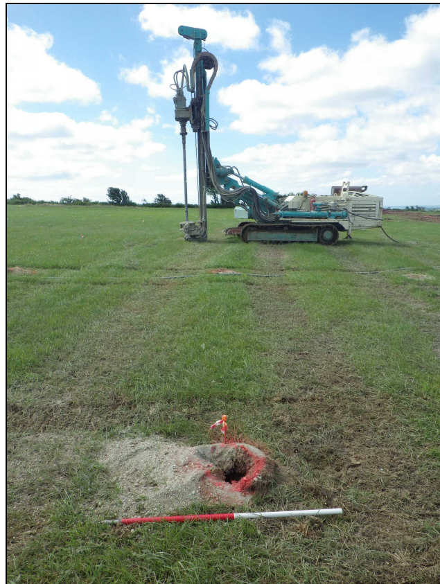
Plate 12: PFL2014_112, boring holes for the supporting posts for the solar panels
