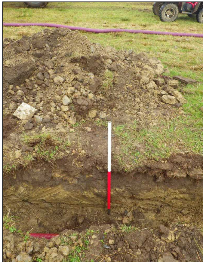
Plate 8: PFL2014_108, section of the main cable trench at SN5351808715, looking east.
