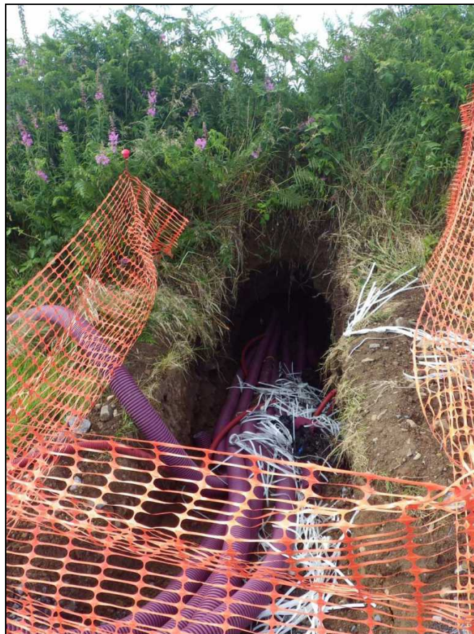
Plate 6: PFL2014_106, cable trench moled beneath boundary bank at SN5349308779, looking north.
