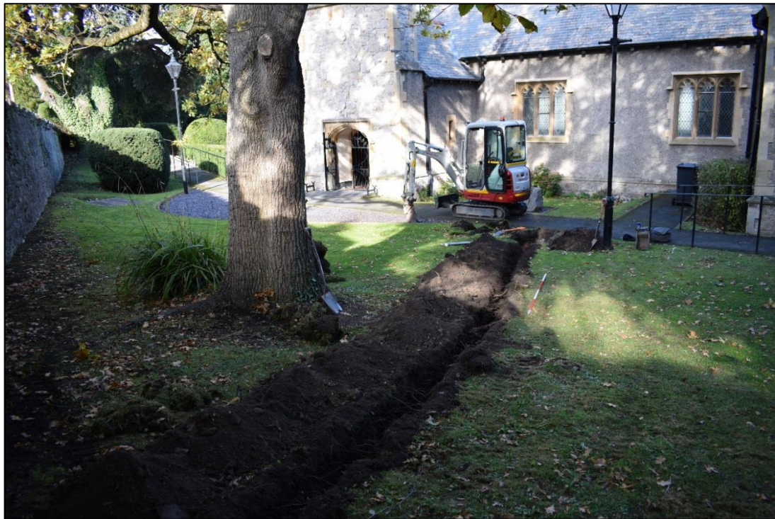
Fig. 3: The southern section of the pipe trench. Photo CPAT 4560-0005
