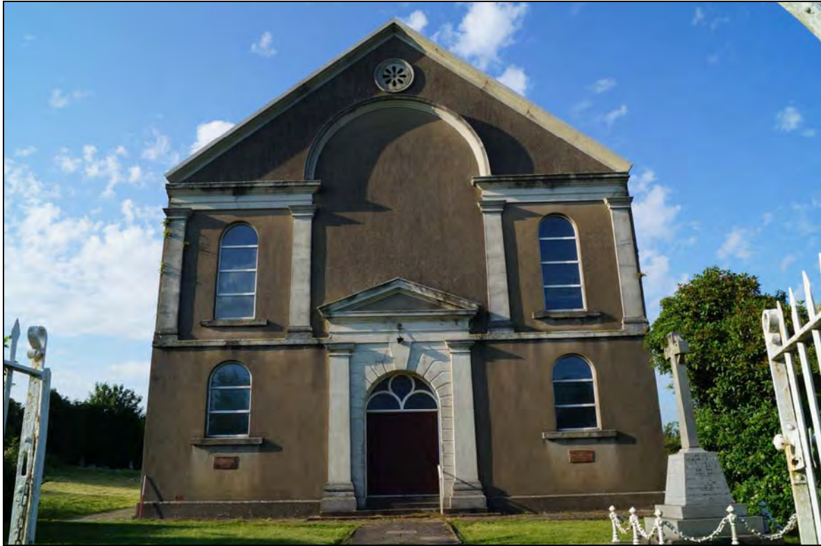
Plate 29: BTC2017_029, external view of the south elevation, looking north-northeast from the gateway.
