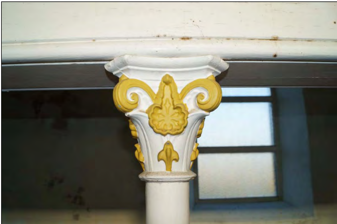
Plate 81: BTC2017_081, a close up of the decorative capital of one of the cast-iron columns supporting the gallery, looking east-southeast.
