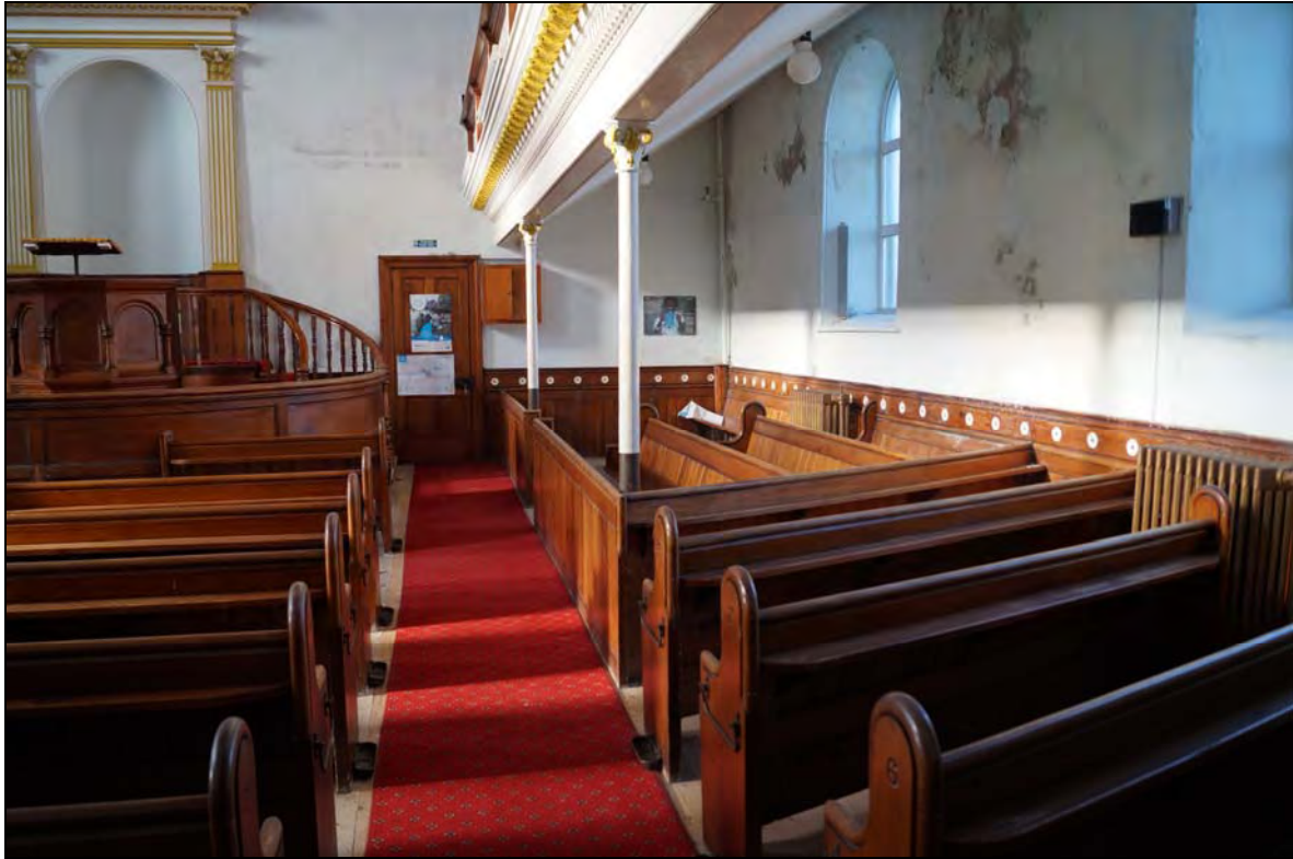
Plate 47: BTC2017_047, internal view of the chapel along the eastern aisle with the pews along the eastern wall to the right, below the gallery, supported on cast iron pillars, looking north-northeast.
