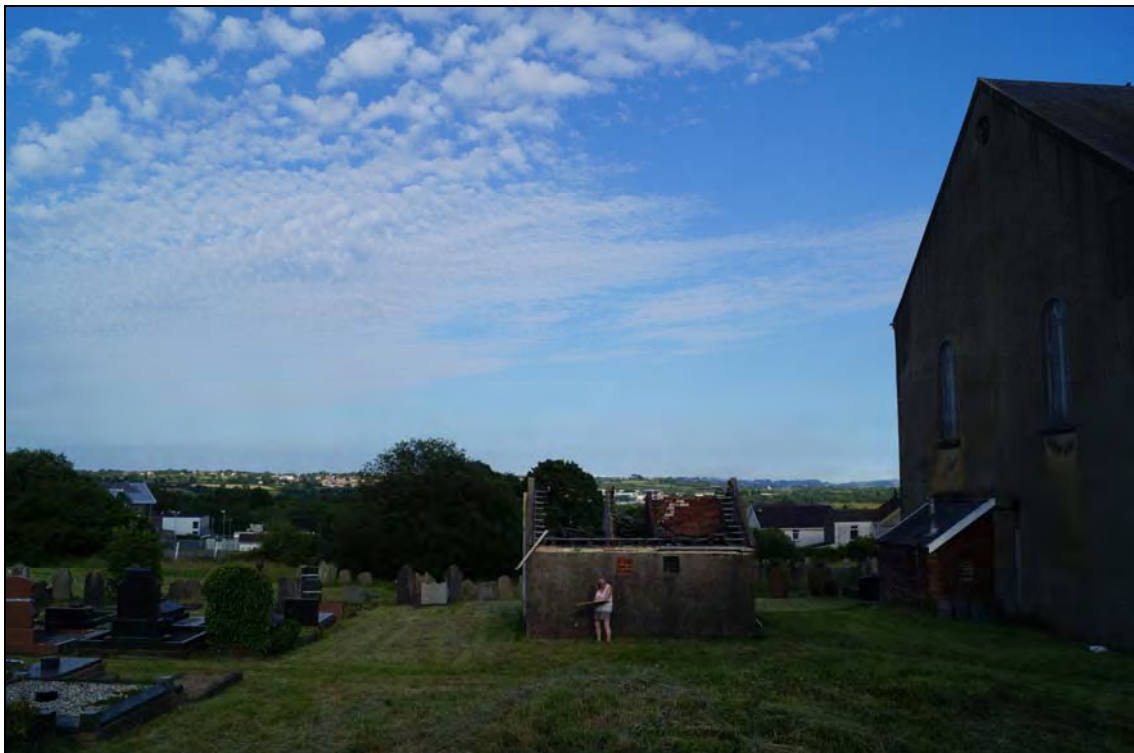
Plate 16: BTC2017_016, External view of the outbuilding to the north of the chapel, looking east-southeast.
