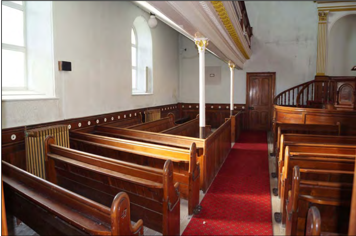
Plate 45: BTC2017_045, internal view of the chapel along the western aisle with the pews along the western wall to the left, below the gallery, supported on cast iron pillars, looking north-northeast.
