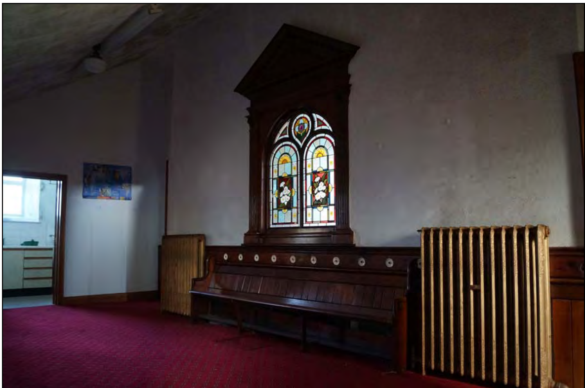
Plate 69: BTC2017_069, the inner lobby and the stained-glass window of the entrance lobby. A pew removed from the chapel when it was truncated to create the inner lobby is placed below the window, with decorative radiators either side. Looking southeast.
