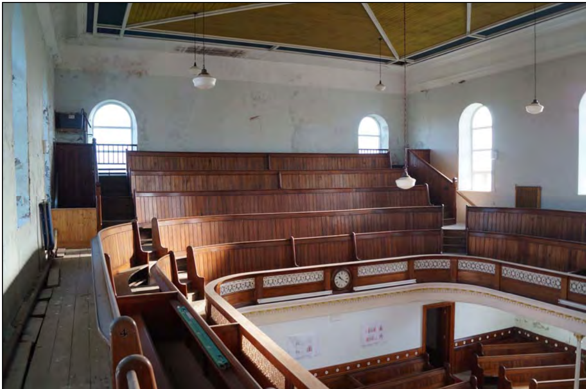
Plate 52: BTC2017_052, internal view of the chapel from the gallery, looking southwest towards the seats at rear of the gallery.
