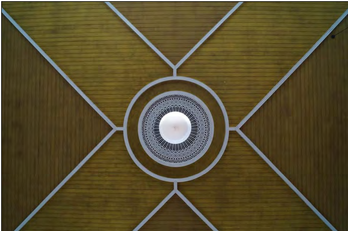
Plate 87: BTC2017_087, a view of the centre of the chapel ceiling, looking upwards from the ground floor.
