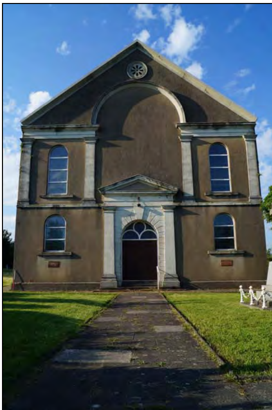
Plate 28: BTC2017_028, external view of the south elevation, looking north-northeast along the path.
