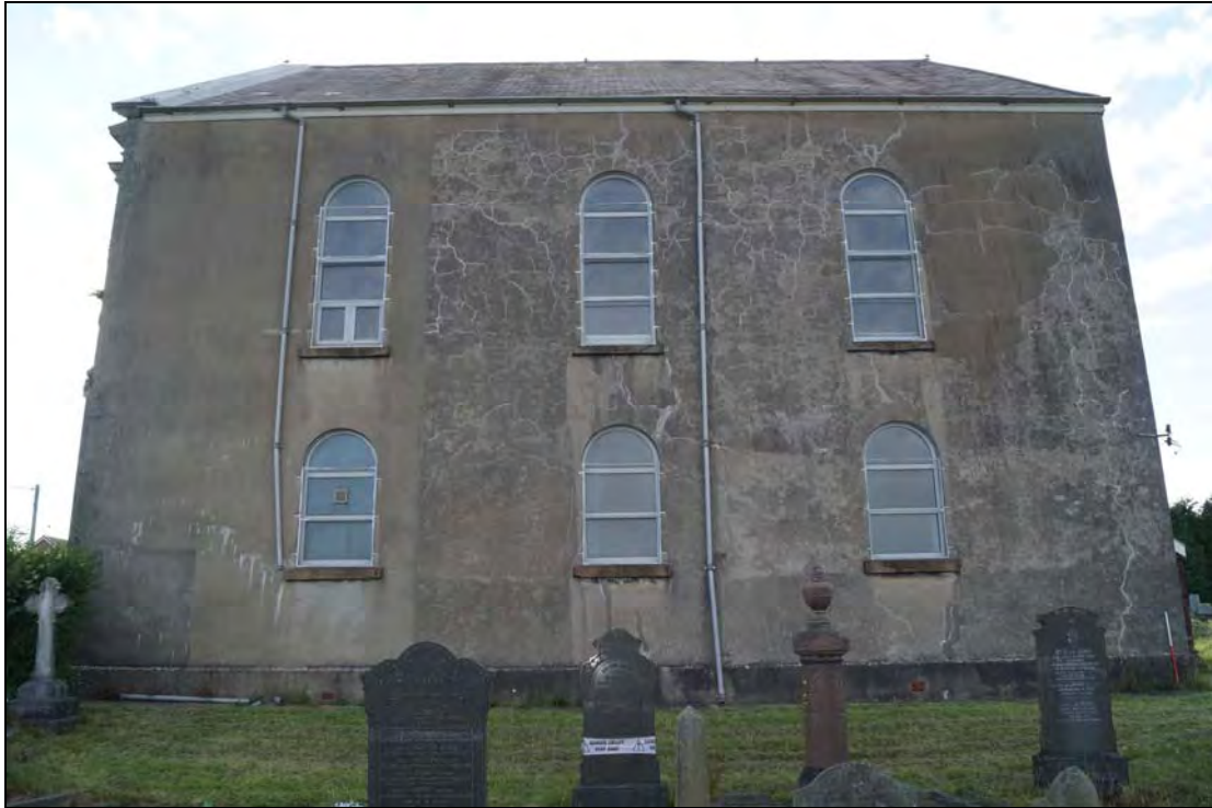
Plate 3: BTC2017_003, external view of east elevation of chapel, looking west-northwest.
