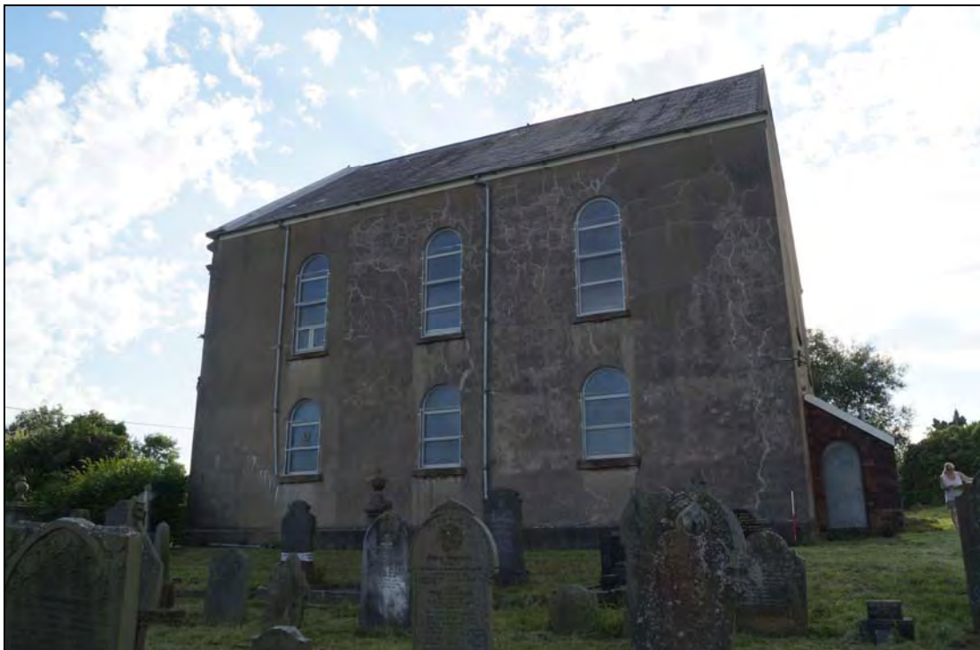
Plate 4: BTC2017_004, external view of east elevation of chapel, looking west.
