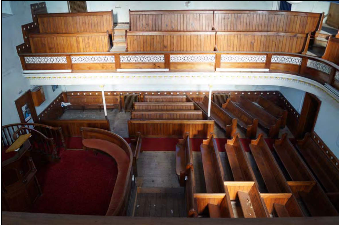
Plate 58: BTC2017_058, a view of the eastern side of the ground floor from the western gallery, with the eastern gallery above, looking east-southeast.
