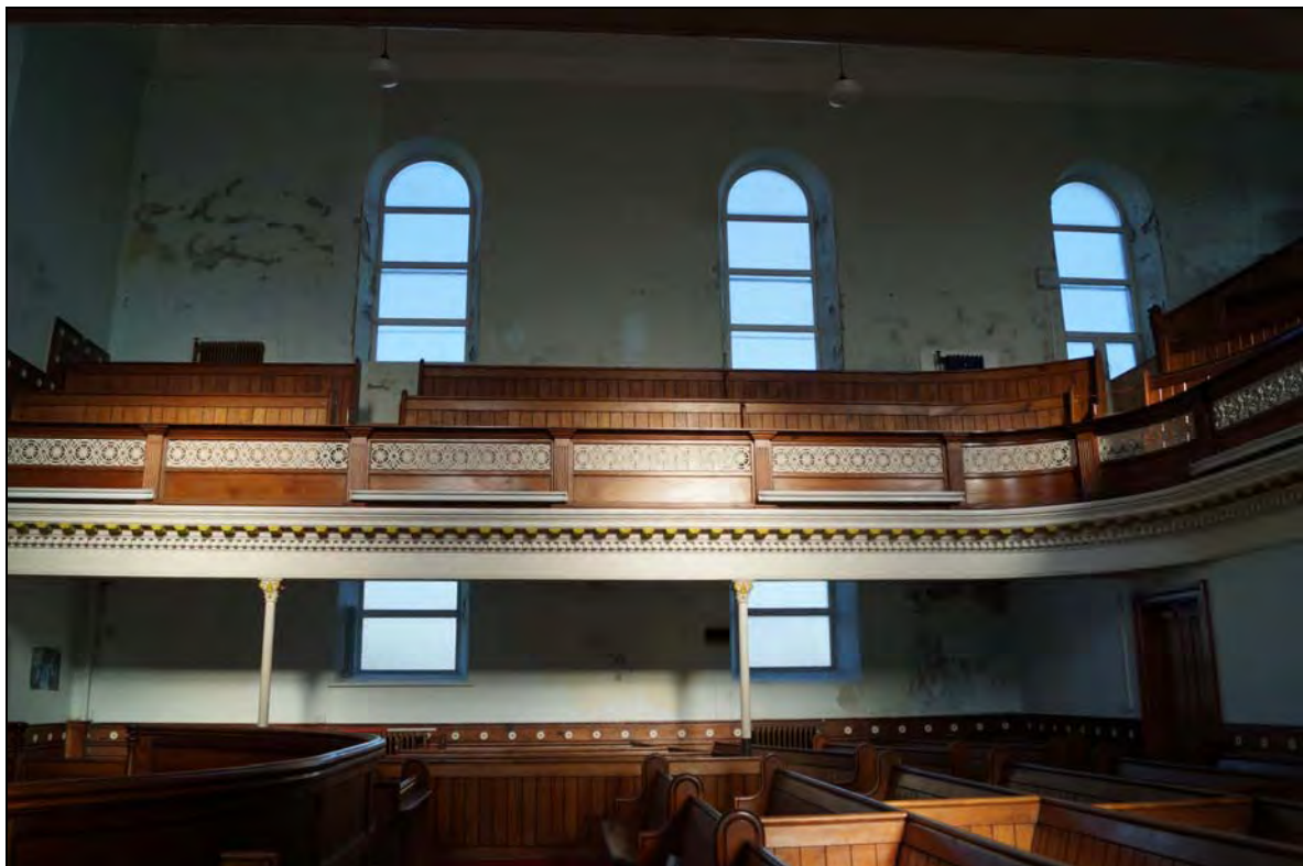
Plate 42: BTC2017_042, internal view of the chapel looking east-southeast across the ground floor with the ornate gallery above, supported on cast iron pillars.
