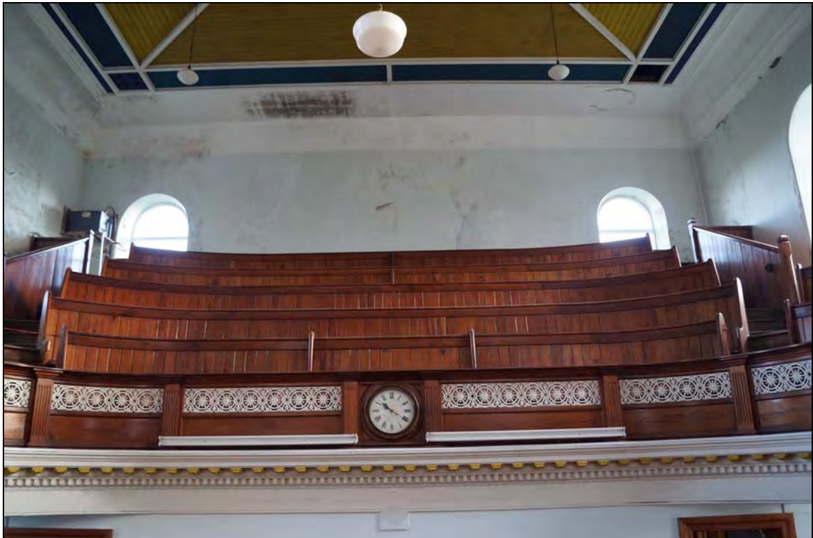
Plate 93: BTC2017_093, a view of the southern gallery, which faces the pulpit, showing the clock, looking south-southwest.
