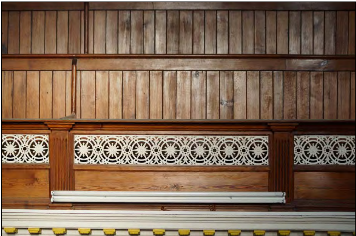
Plate 55: BTC2017_055, gallery seats and the decorative cast-iron tracery of the eastern side of the gallery, looking east-southeast.
