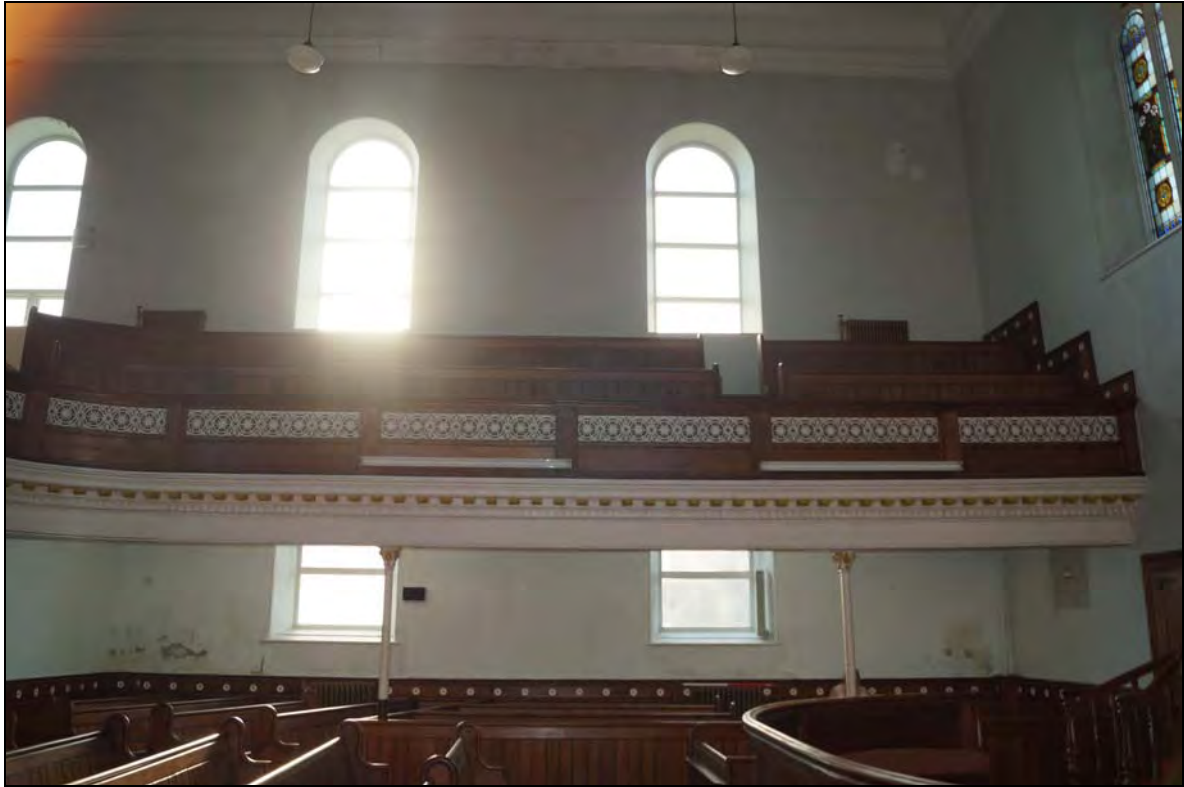
Plate 43: BTC2017_043, internal view of the chapel looking west-northwest across the ground floor with the ornate gallery above, supported on cast iron pillars.
