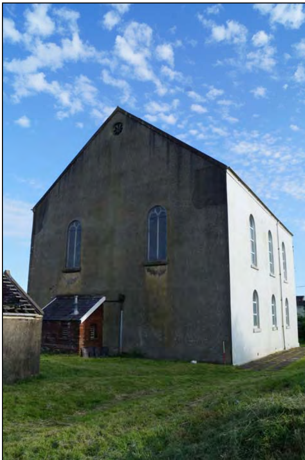
Plate 12: BTC2017_012, External view of north elevation of chapel, looking south.
