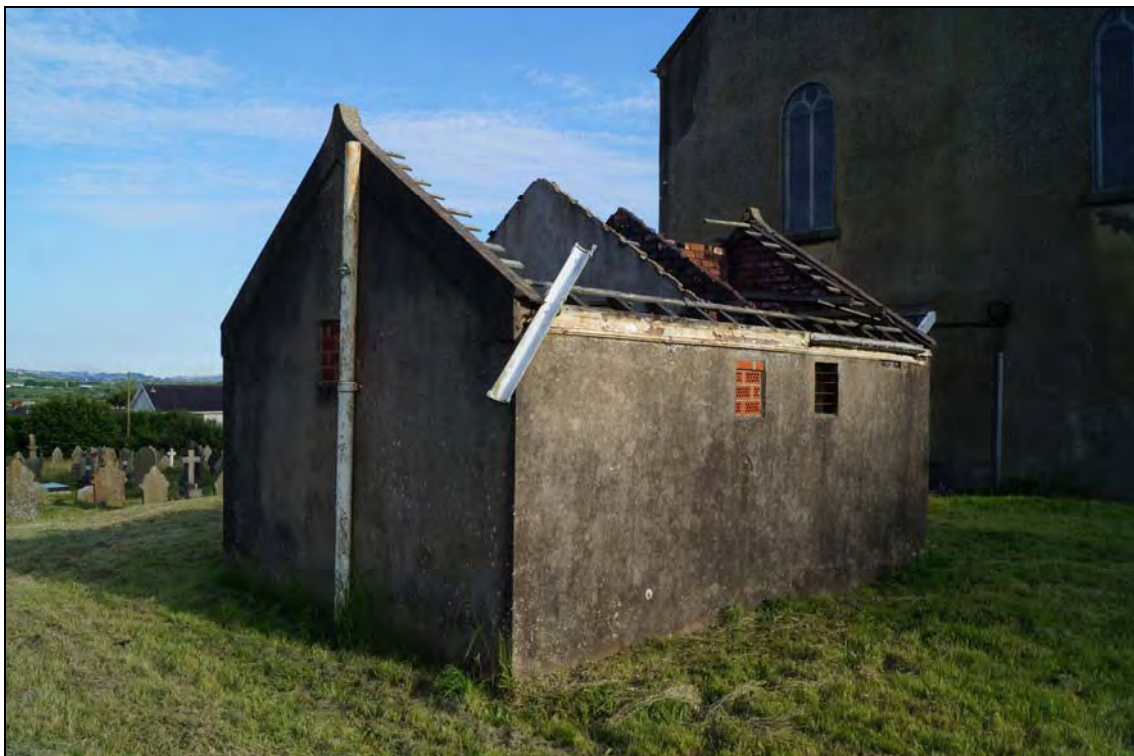
Plate 10: BTC2017_010, external view of outbuilding to north of chapel, looking east-northeast.
