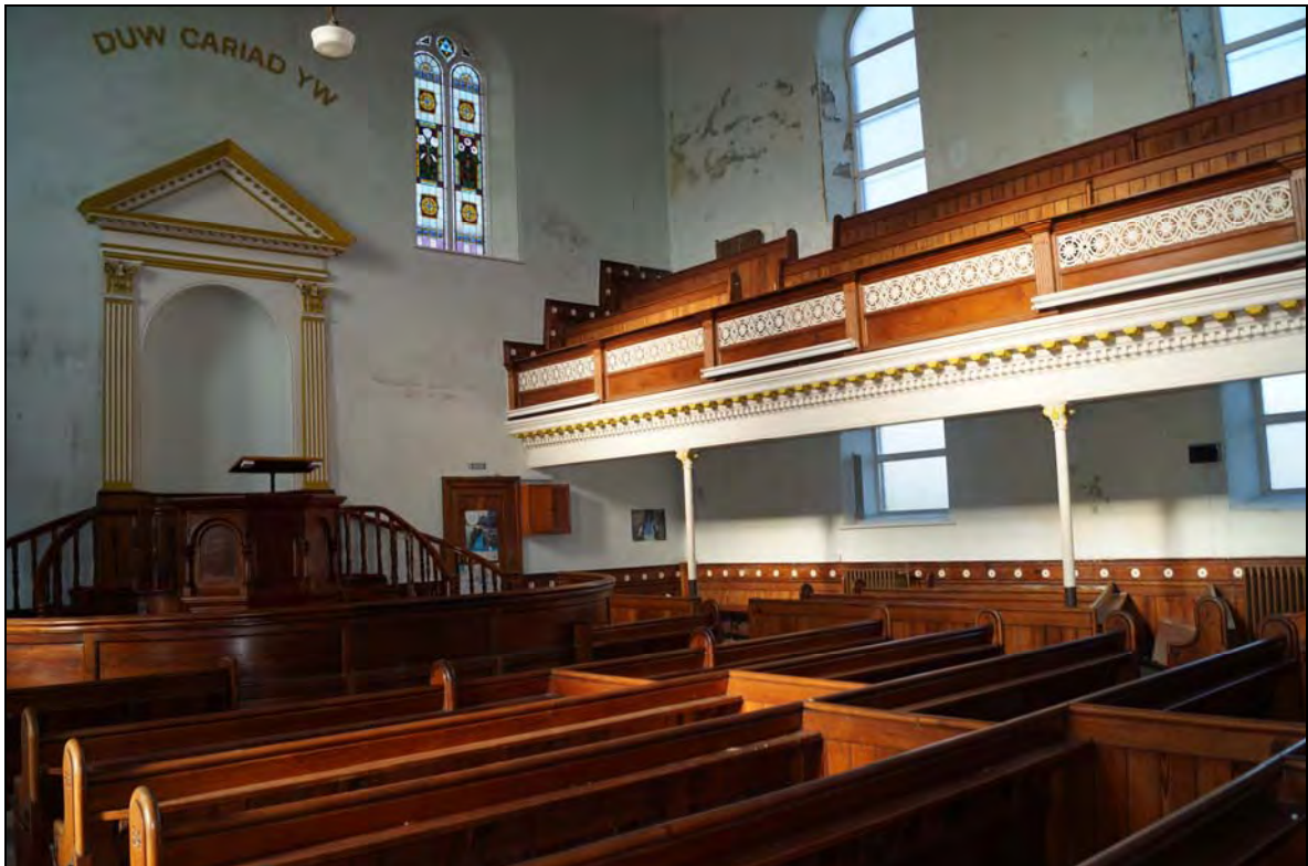
Plate 44: BTC2017_044, internal view of the chapel looking northeast across the ground floor with the ornate gallery above, supported on cast iron pillars.
