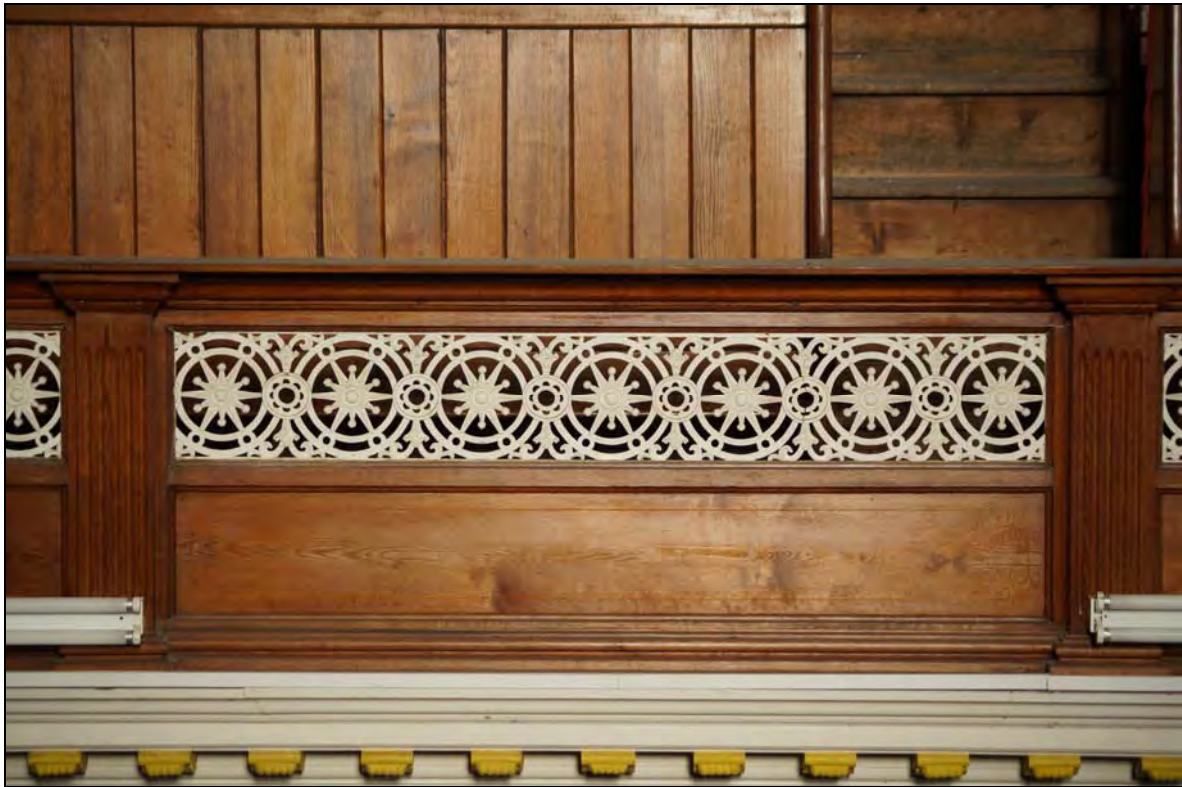
Plate 56: BTC2017_056, a closer view of the decorative cast-iron tracery fronting the eastern side of the gallery, looking east-southeast.
