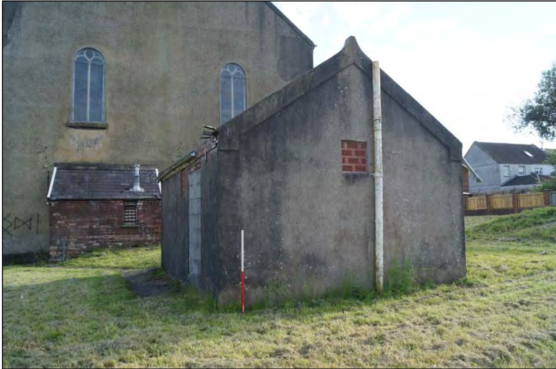
Plate 11: BTC2017_011, external view of outbuilding to north of chapel, looking south-southwest.
