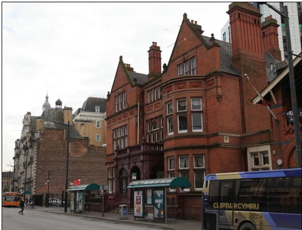
Figure 7 Former County Club. Source: Lichfields, January 2019.
