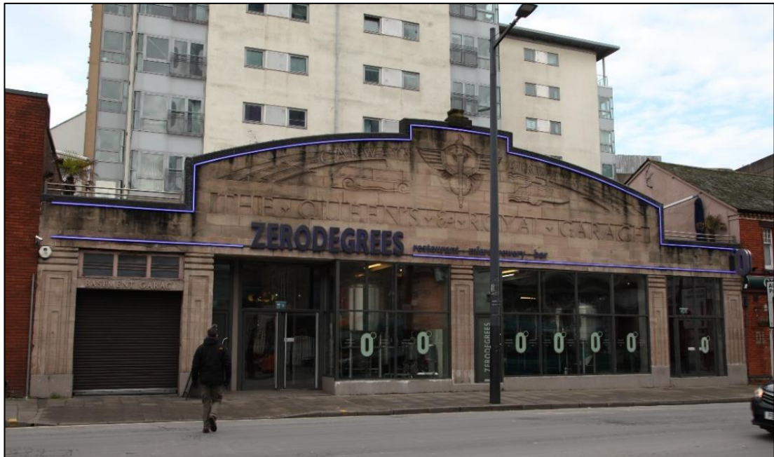
Figure 9 The Queens & Royal Garage. Source: Lichfields, January 2019.
