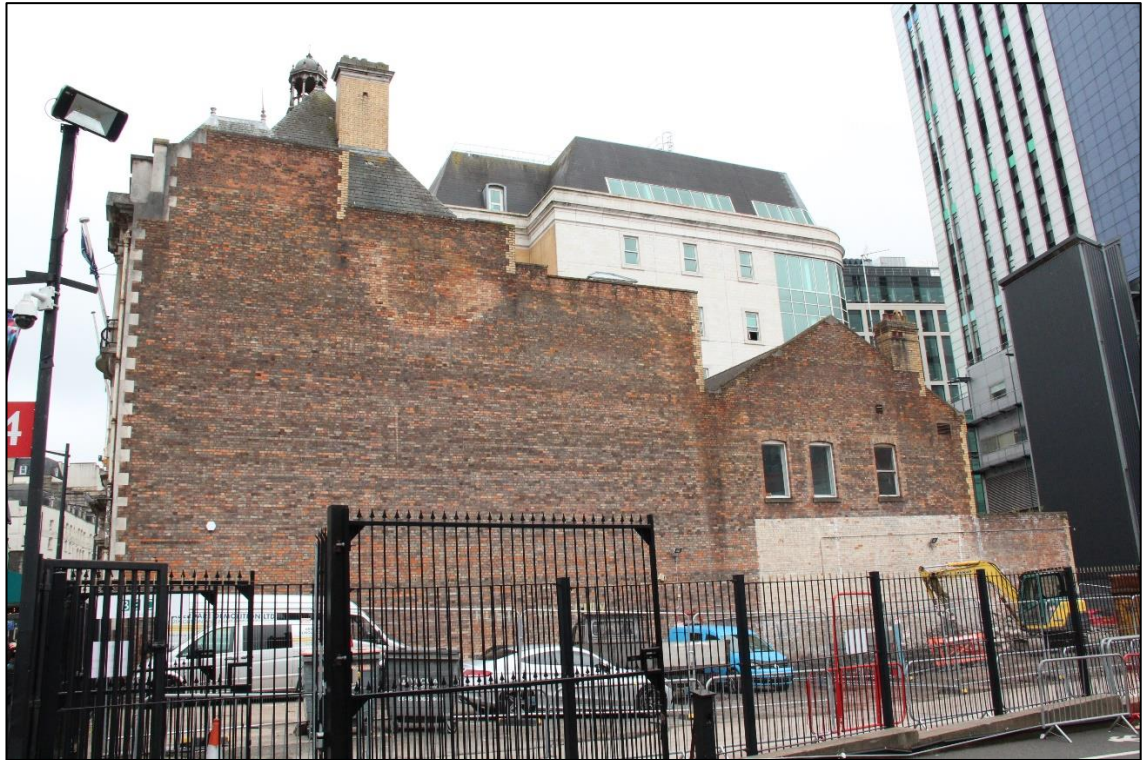
Figure 2 View of the side elevation of the former County Court and Inland Revenue Offices. Source: Lichfields, Sept 2019.
