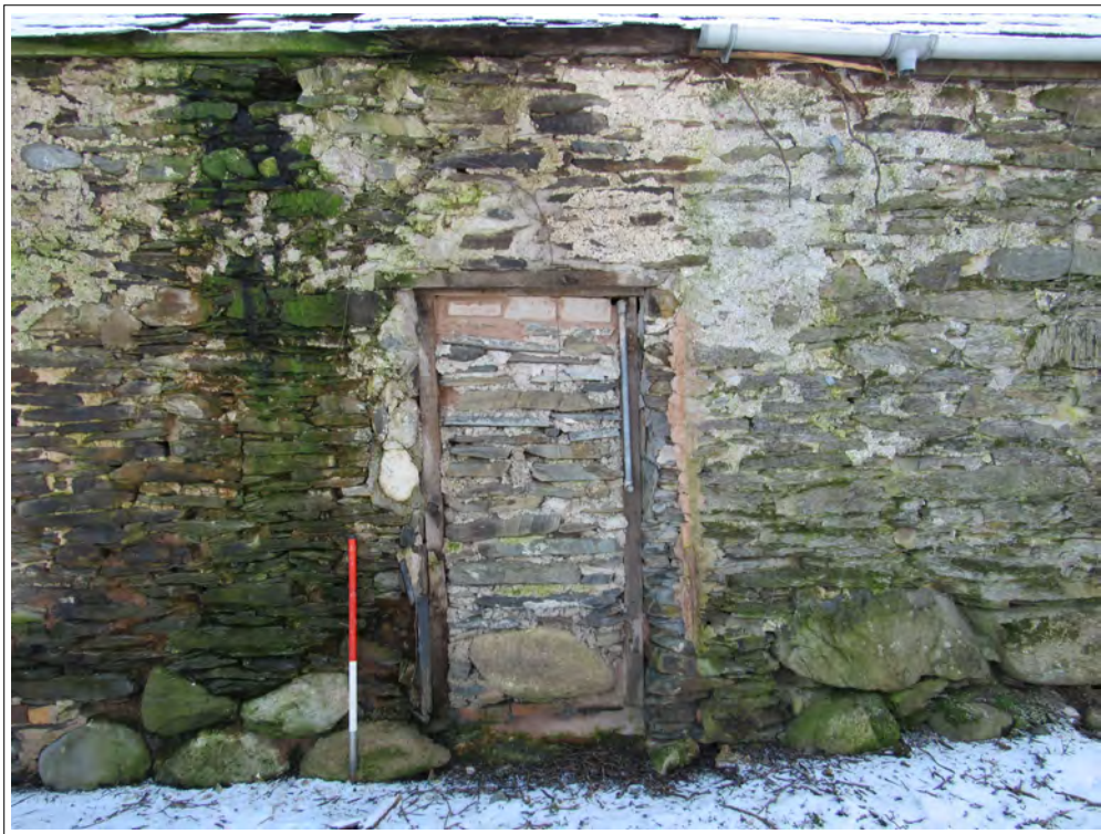
Plate 22. The barn north-west elevation blocked doorway, view south-east. 1m scale
