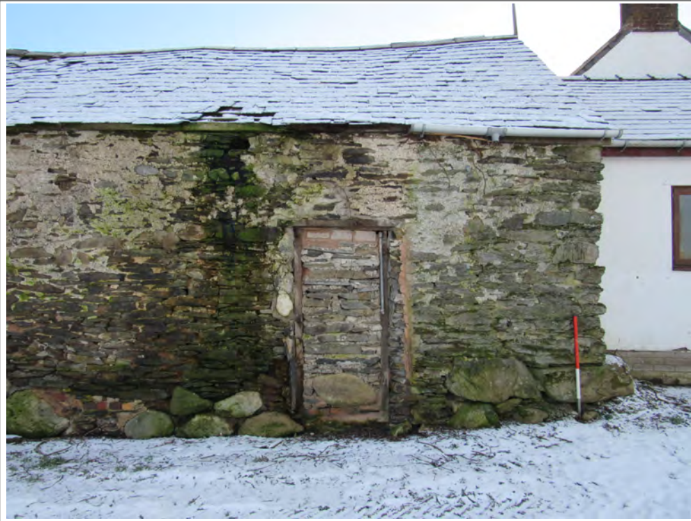
Plate 19. The barn north-west elevation blocked doorway, view south-east. 1m scale
