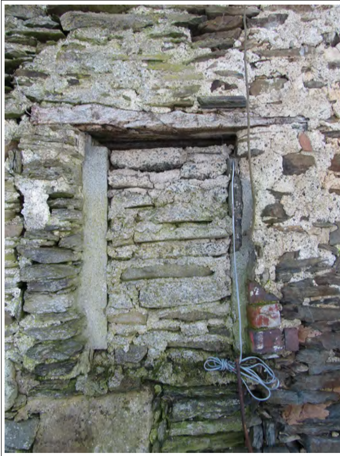
Plate 21. The barn north-west elevation blocked window, view south-east. 1m scale
