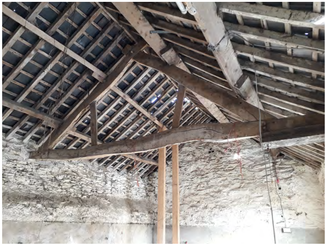
Plate 31. Barn interior with mortise and tenon jointed and pegged roof truss, view north-east.
