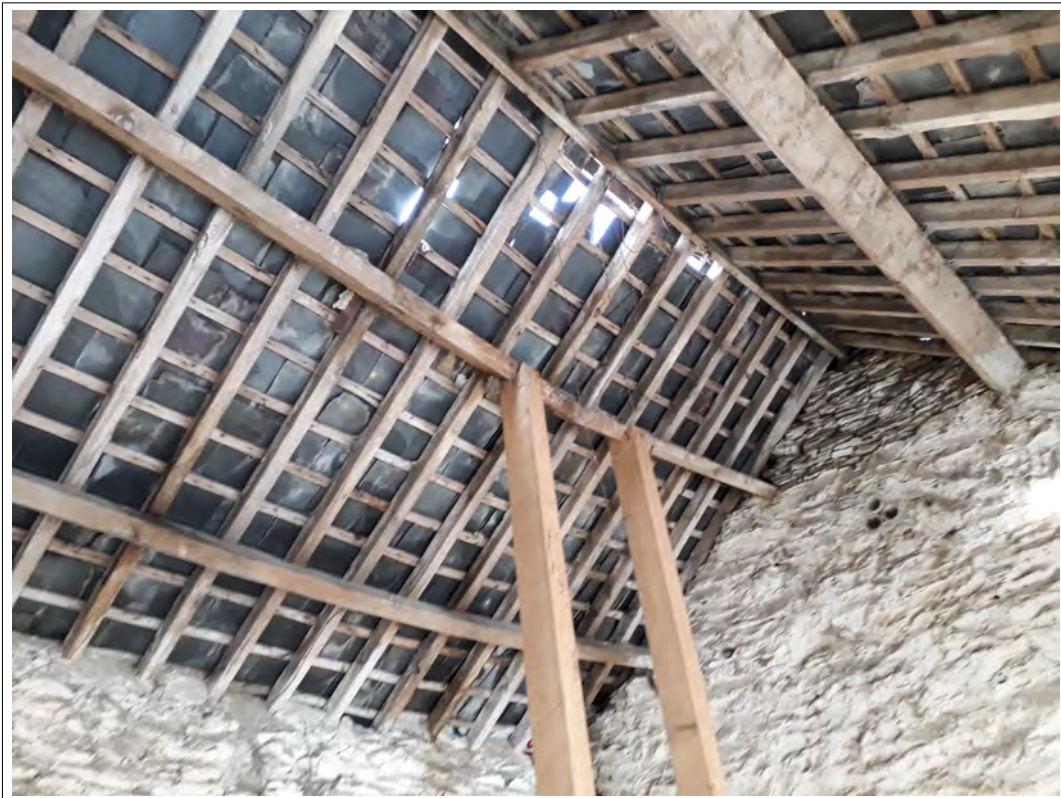
Plate 34. Barn interior purlin damage with modern supports, view north-east.
