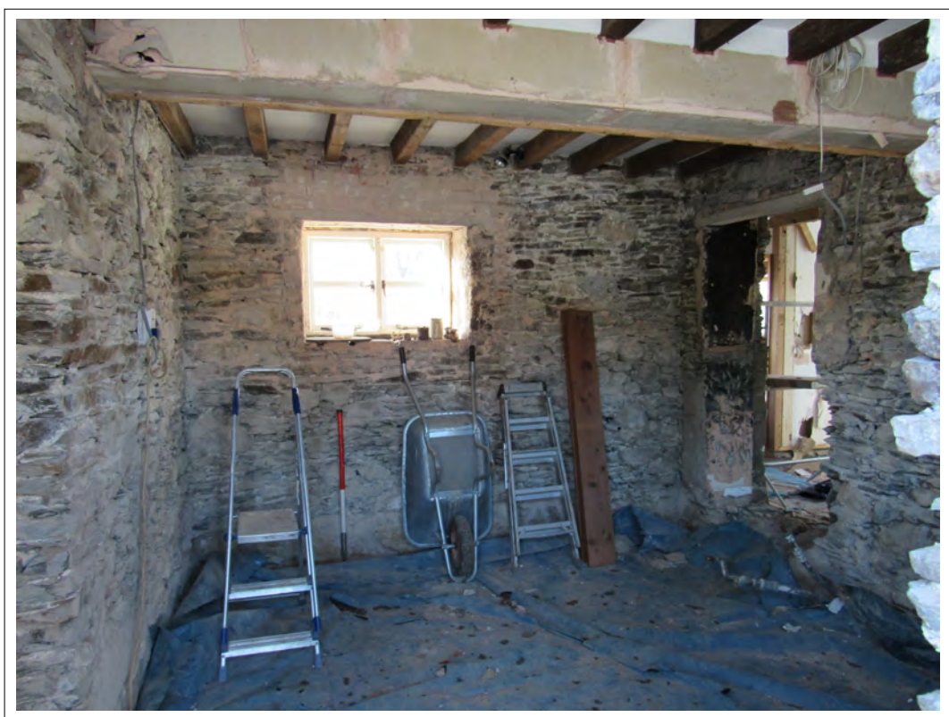
Plate 42. Kitchen in original house with inserted doorway to modern extension, view south-west. 1m scale.
