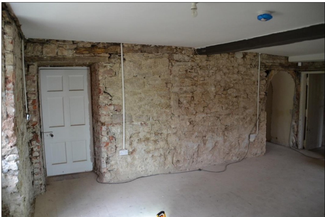
Fig. 10 Exposed south-west wall in Room G14. Photo CPAT 4404-0006
