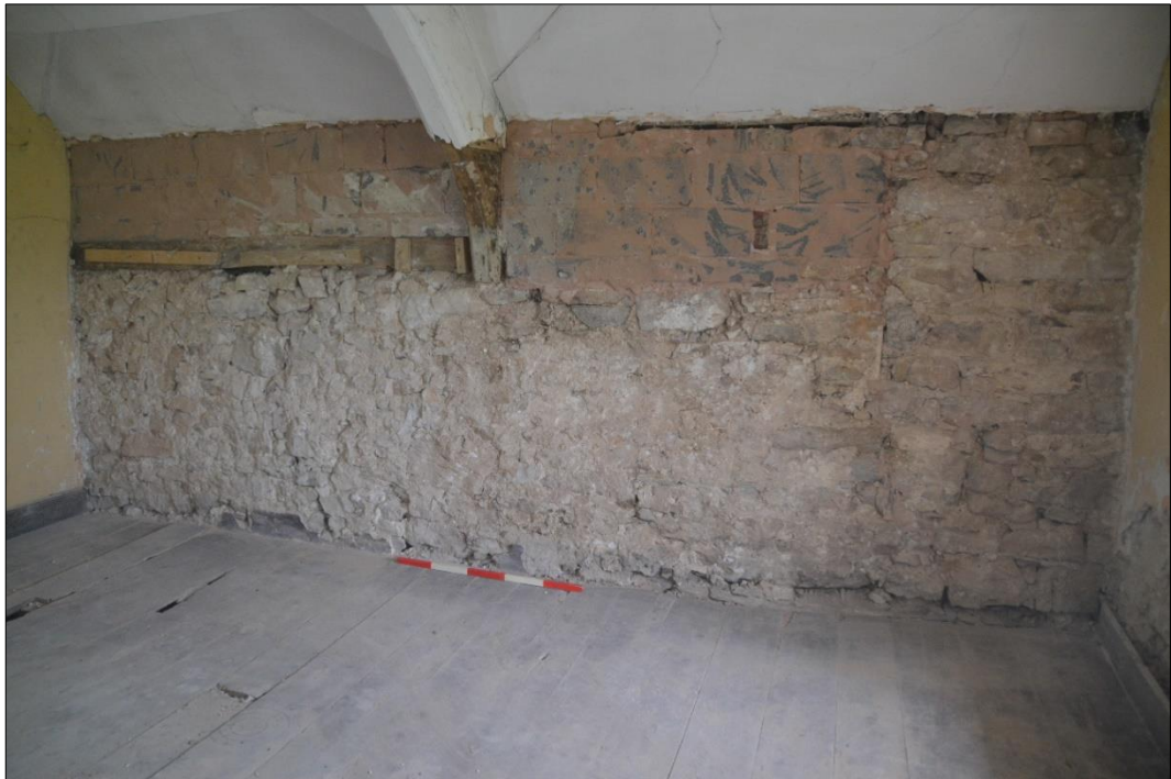
Fig. 11 Exposed walling in Room S06. Photo CPAT 4404-0011
