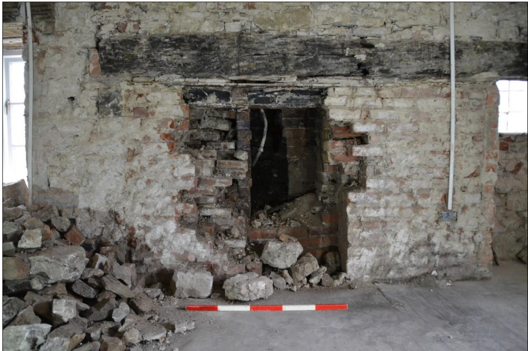
Fig 9 The original fireplace opening in Room G14. Photo CPAT 4404-0002
