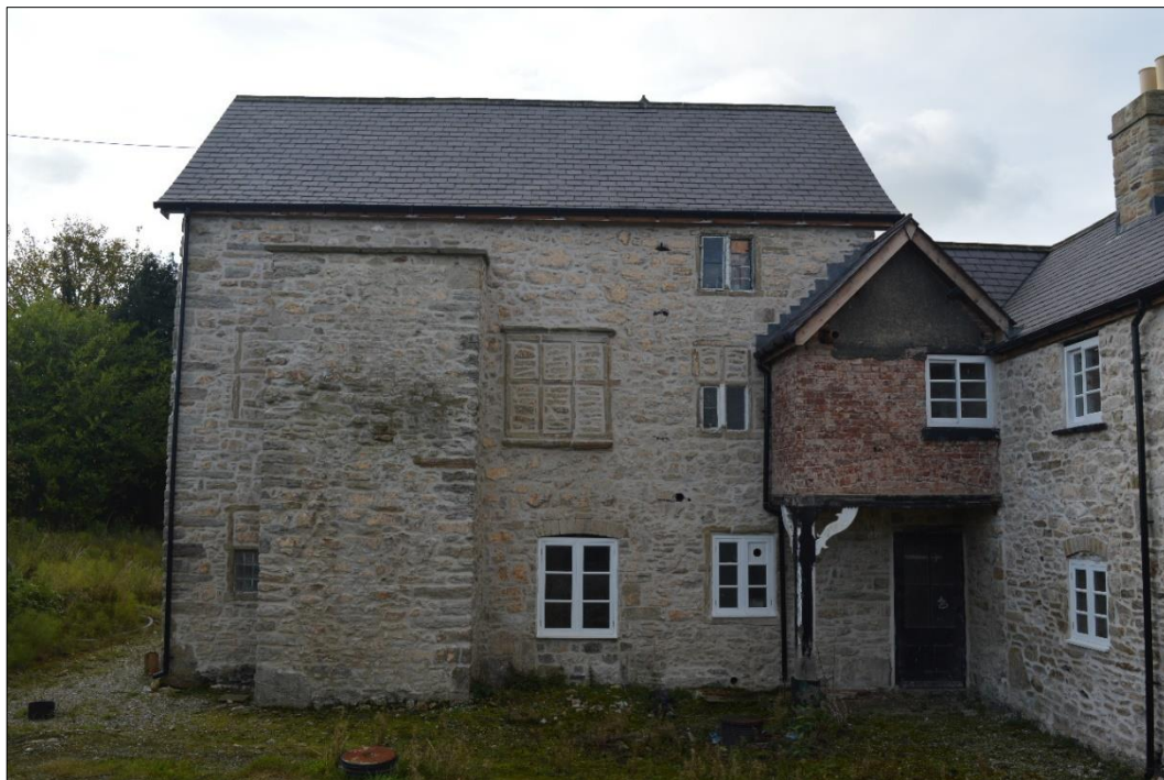
Fig. 3 The south-west elevation of the 16 th -century range. Photo CPAT 4246-0001
