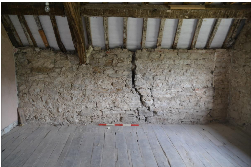
Fig. 12 Exposed walling in Room S03 showing substantial displacement of masonry, with a blocked window to the right of the crack. Photo CPAT 4404-0024
