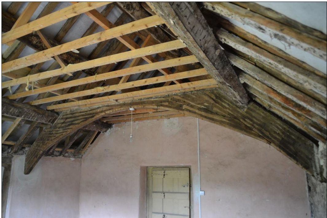
Fig. 14 Original roof truss in Room S03. Photo CPAT 4404-0034
