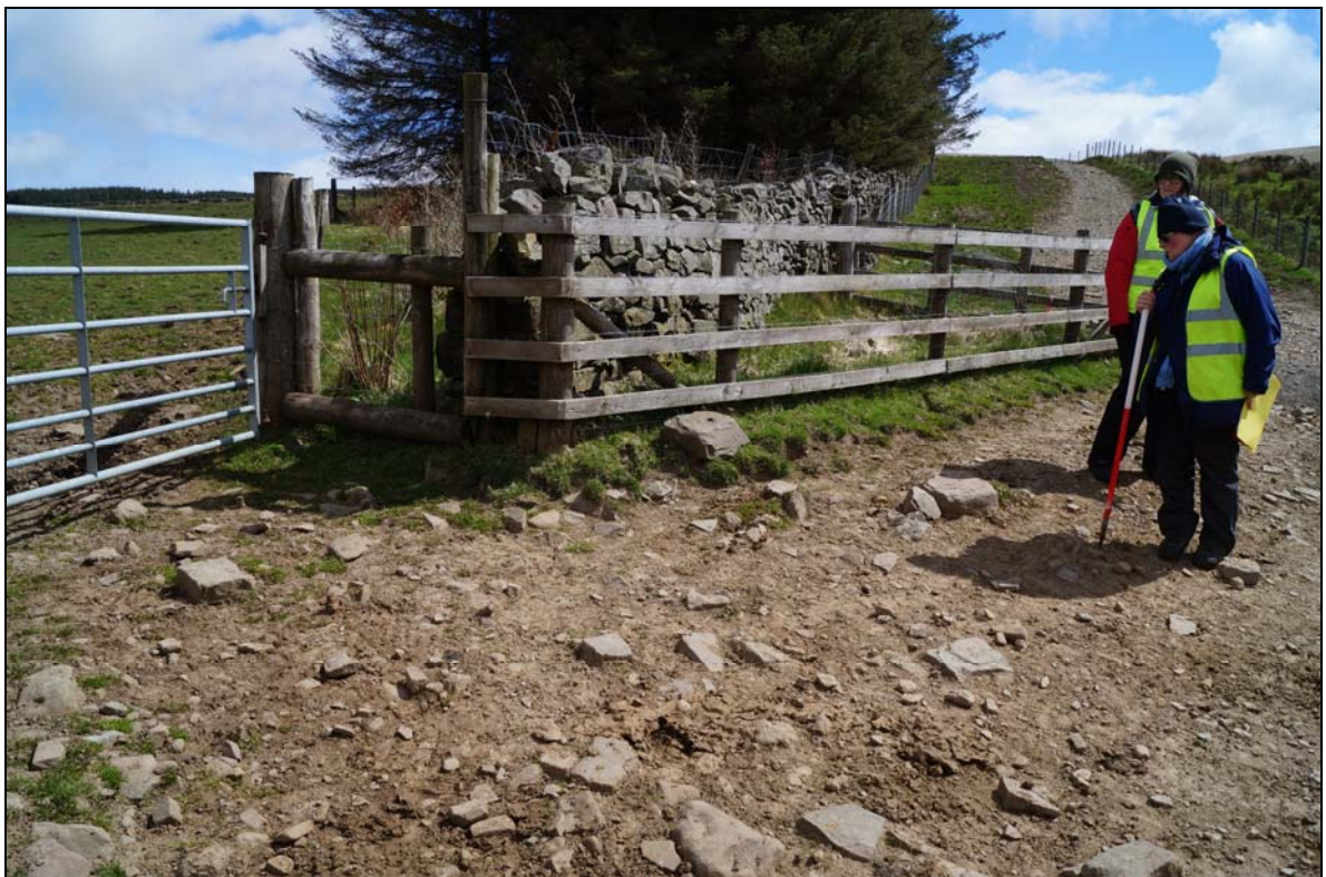
Plate 18: CNX2016_114, Detail of iron pegs/bolts, possible remains of tramroad CNX2016_007, looking east.
