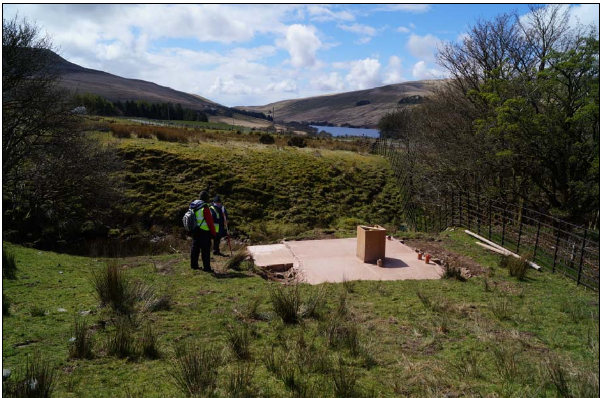
Plate 22: CNX2016_122, Micro hydro turbine housing, CNX2016_011, where water will be returned to the Nant Cnewr Fach stream.
