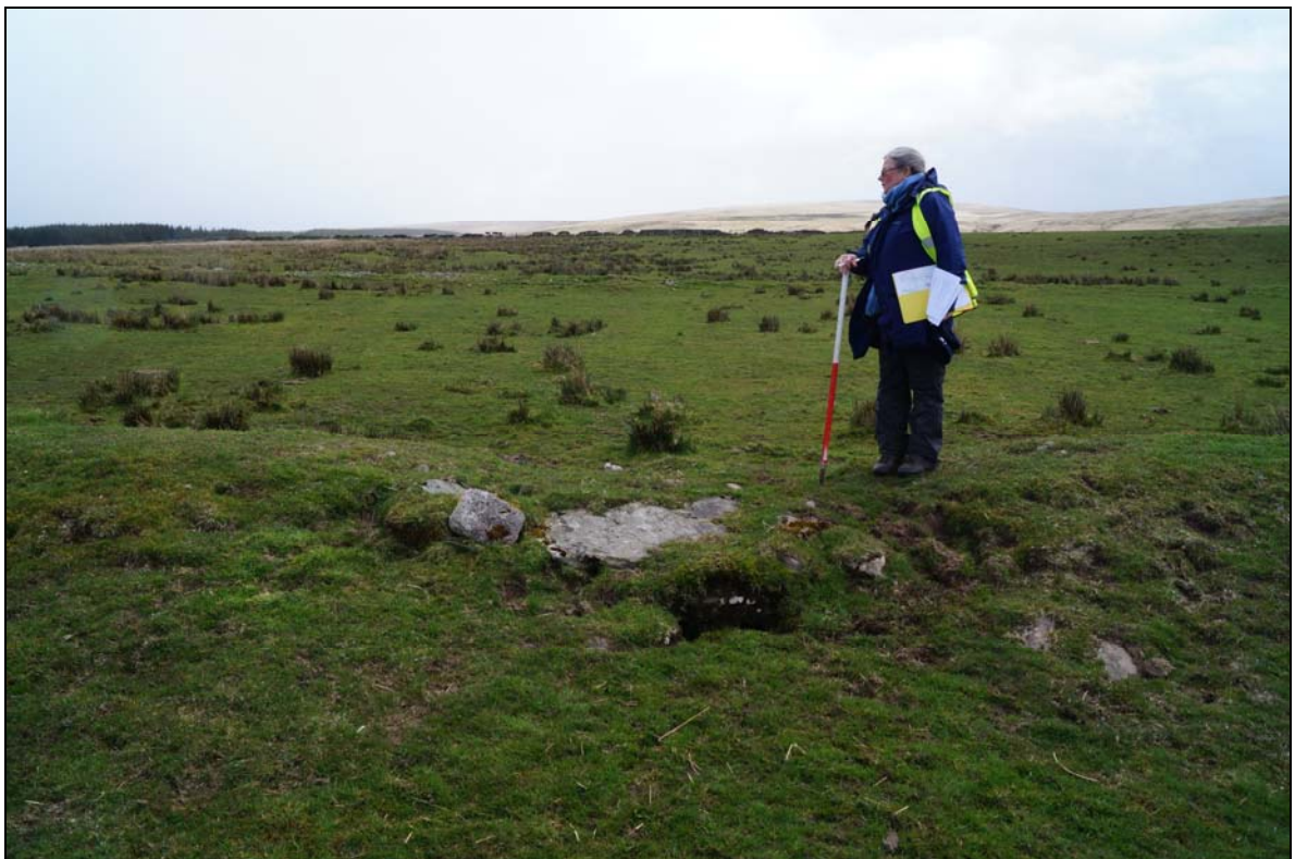
Plate 16: CNX2016_116, Culvert, CNX2016_008, through tramroad, CNX2016_007, looking southeast.
