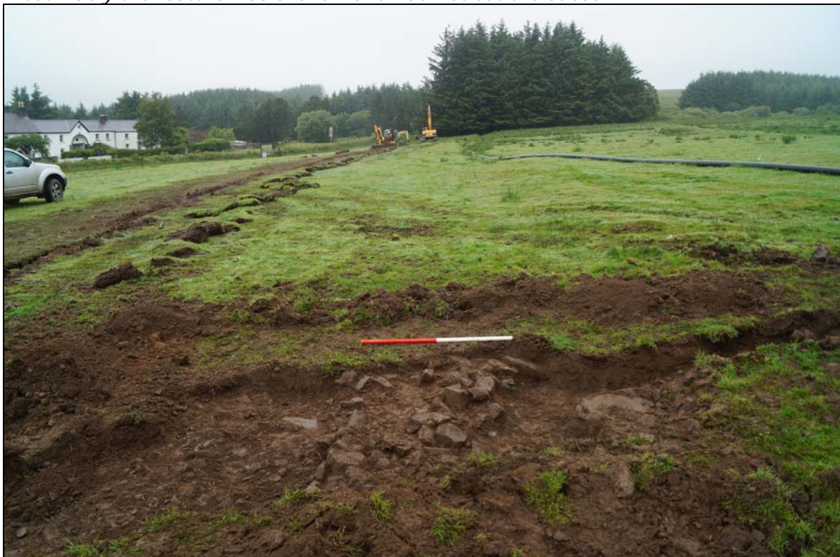
Plate 4: CNX2016_126. Looking north across the hand excavated area of the water pipeline trench, showing the remains of the tramway, context, CNX2016_202.
