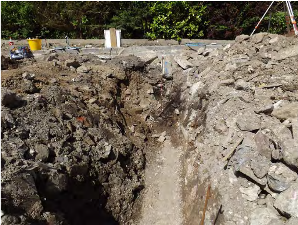
Plate 4: Concrete slab (107) in slot 1 (northern), shot facing west.
