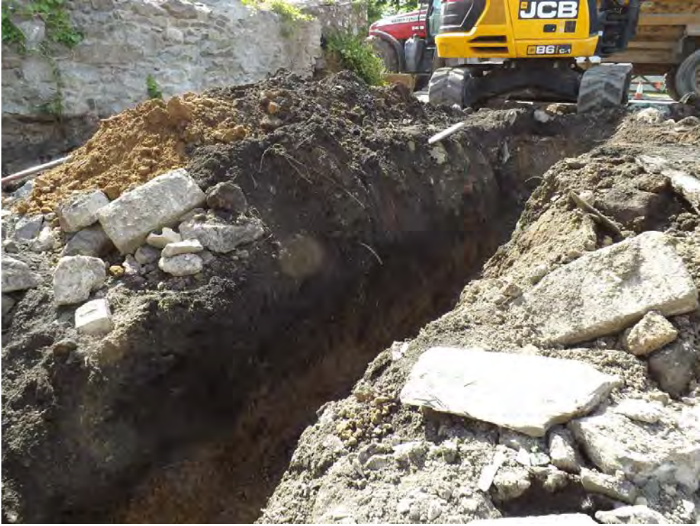
Plate 7: Oblique view of slot 3 (middle), (108) and (109), shot facing southeast.
