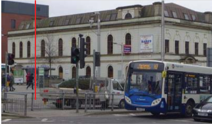
Figure 2.10: Northern Elevation of the Former Custom House (original building to the right and rebuilt extension to the left)
