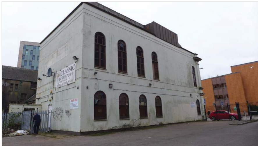
Figure 2.12: Eastern Elevation of the Listed Building
