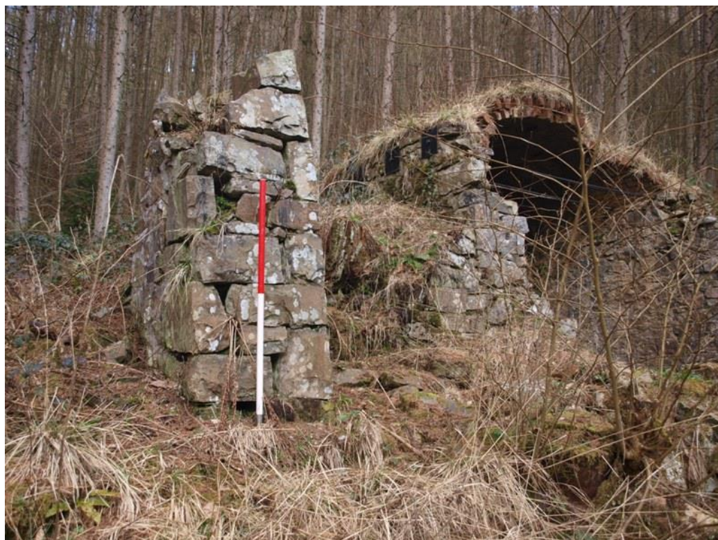
Fig. 10. Elevated Leat (W 4 ). Detail of one of the stone supporting pillars, adjacent to the Expense Magazine (B12)..
