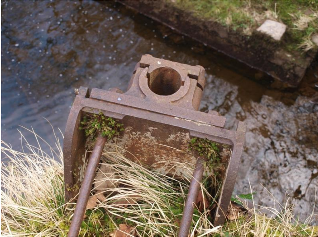
Fig. 18. Detail of iron fixtures on the Main Weir (W11).
