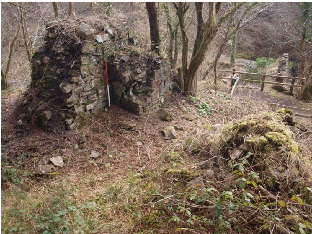
Fig. 13. Structure at the junction of the Elevated Leat (W 4 ), the Lower Leat (W 12 ) and the 'Clean Gangway' (W 7 ). View looking south, with the Waterwheel (W 8 ) in the background, beyond the line of the Main Tramway (T 1 ).
