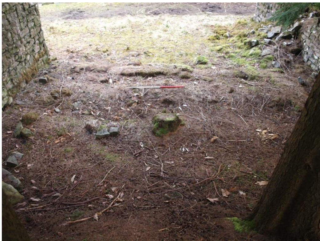
Fig. 25. Pellet House (B3). View from the embankment to the west, showing the sleeper walls and foundations. Magazine (B1) is to the left, Magazine (B3) is to the right.
