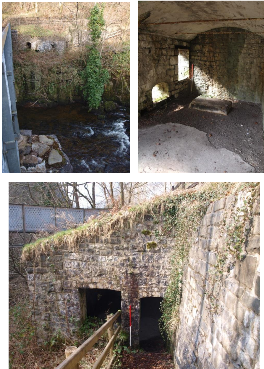
Fig. 19. 6hp Turbine and Pump House (W14). Top left: view from across the river, looking along the modern footbridge built on the abutments of the Lower Aqueduct (W13). Top right: interior view, showing the arched roof, concrete floor, machine base and aperture for a bearing block. Bottom: exterior view looking south-west, with the footbridge behind.
