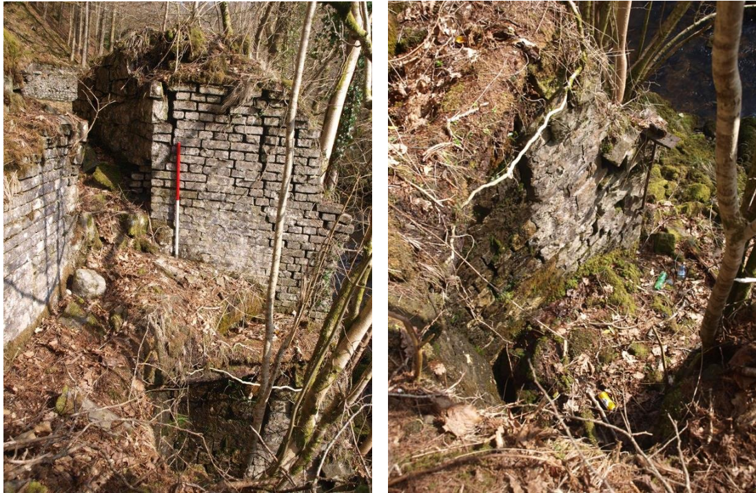
Fig. 12. The 12-15hp Turbine House (W6). Left: View of the superstructure at the level of the Main Tramway, looking north. Right: view down into the turbine housing.
