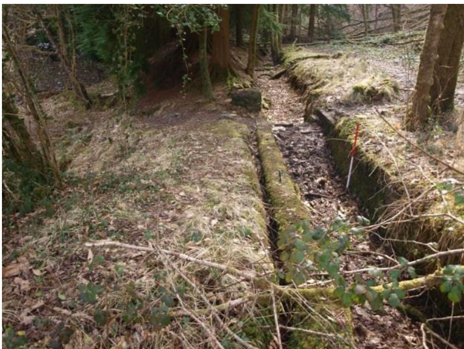
Fig. 7. Upper Leat (W3), north end. Looking south from the interface with the former aqueduct, showing showing the brick and concrete former sluice emplacement (foreground) and the stone-lined main channel running towards the Boiler House (B7).
