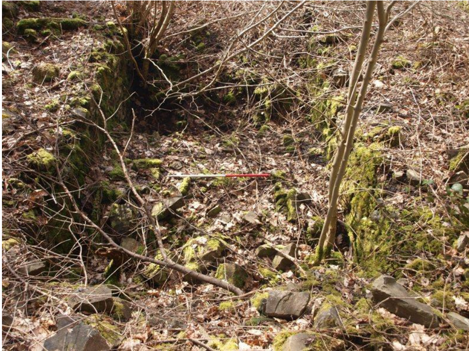
Fig. 36. Corning House (B15). The possible power transmission pit in the centre of the building; view looking south from the northern end of the building.
