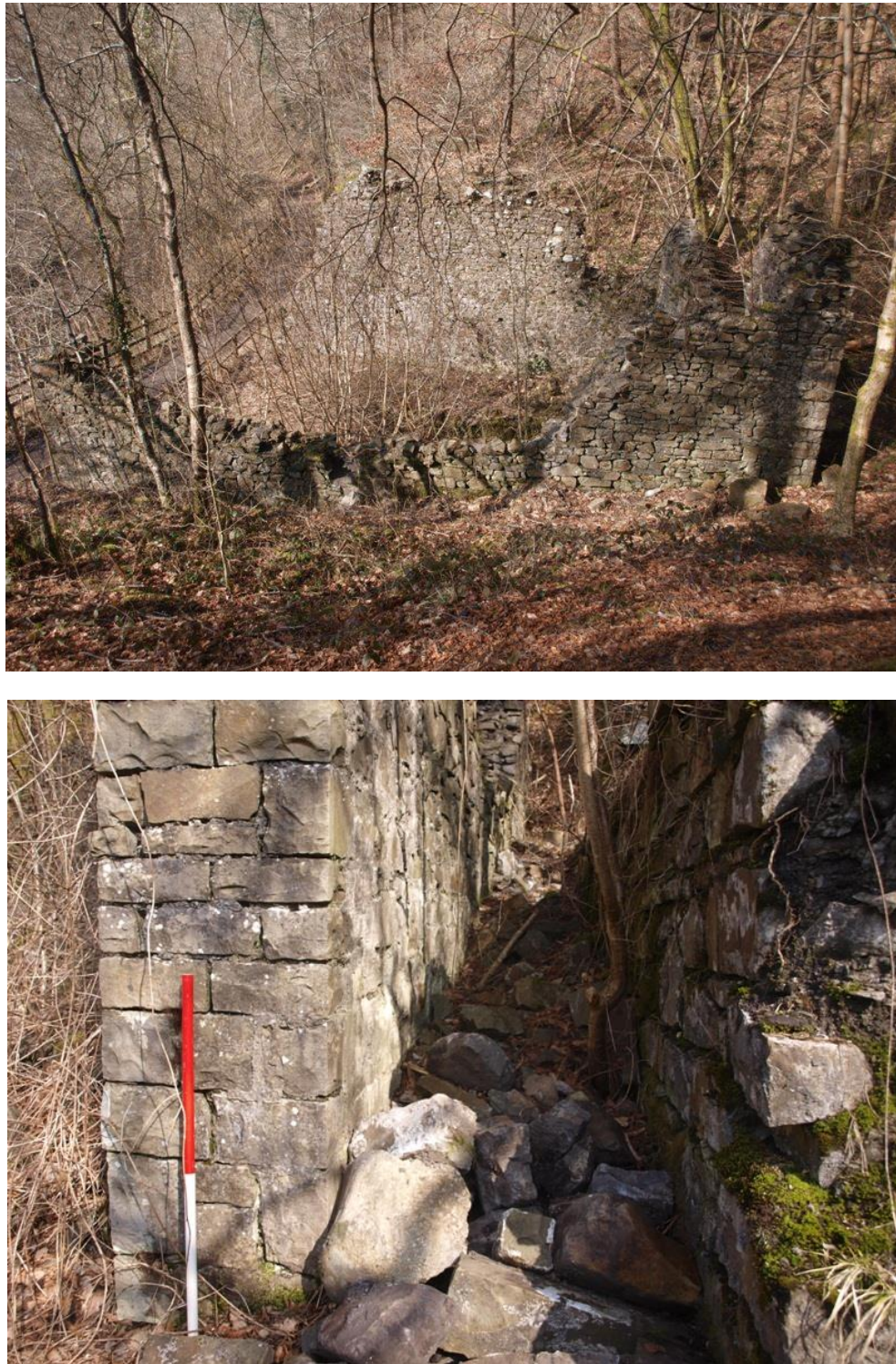
Fig. 35. Corning House (B15). Top: general view looking east from the line of the 'Clean Gangway' (W7), with the tramway and river to the left. Bottom: detail of the south-eastern corner of the building, showing the well-finished end to the east wall on the left, and the retaining wall on the right.
