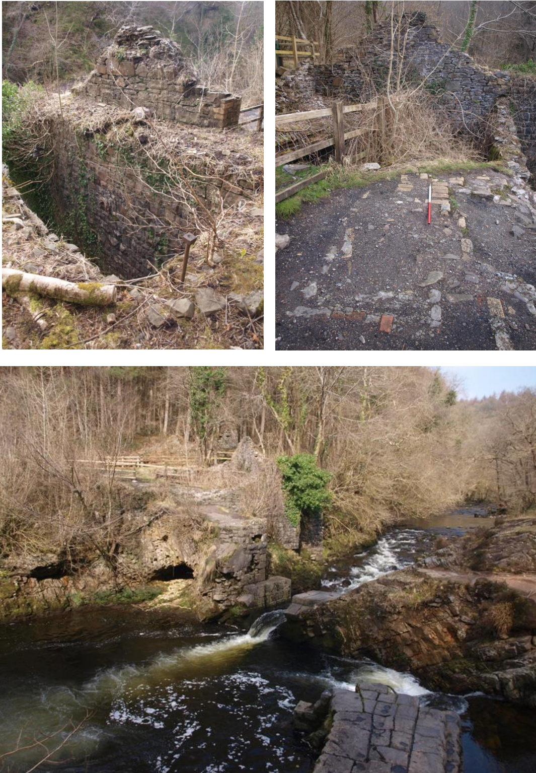
Fig. 15. Waterwheel (W8) and 18hp Turbine and Pump House (W9). Top left: the top of the Wheelpit with the gable wall of the Pump House. Top right: the interior of the Pump House. Bottom: Both structures viewed from the east side of the river, showing the relationship between them and the Main Weir (W11).
