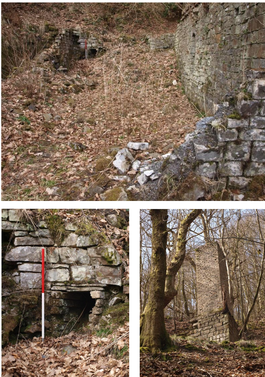
Fig. 29. Boiler House (B6), Flue (B7) and Chimney (B8). Top: the interior of the Boiler House looking west. Bottom left: detail of the entrance to the flue in the western wall of the Boiler House. Bottom right: the Chimney.
