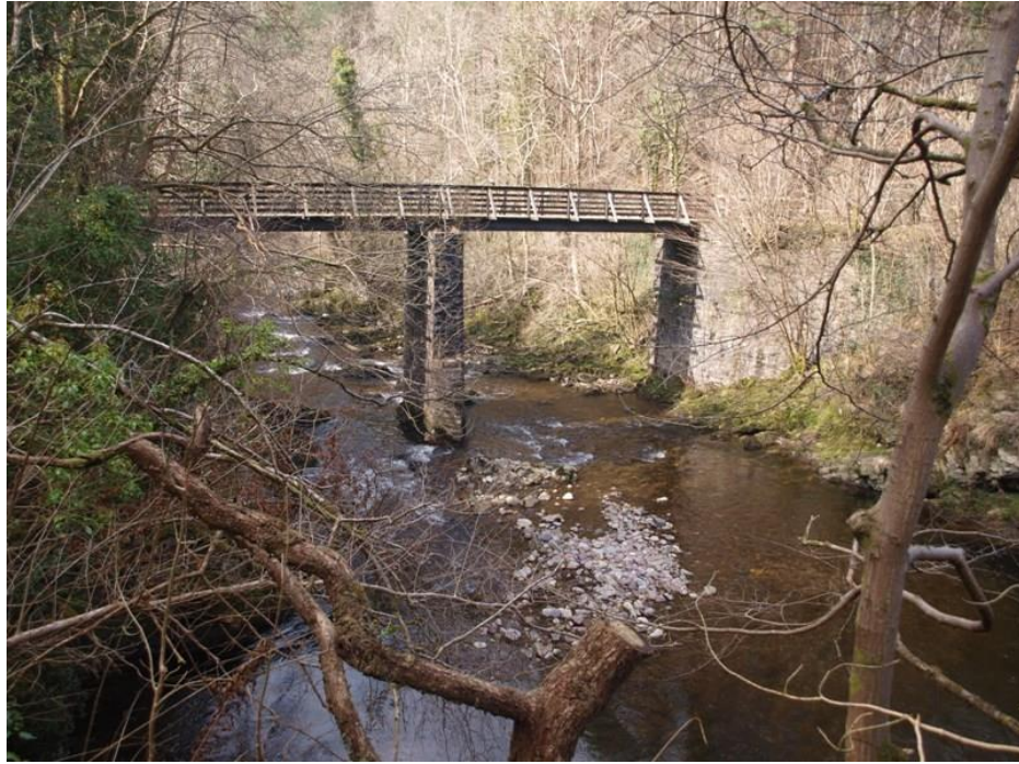
Fig. 21. Lower Tramway Bridge (T6). View from the east showing the upstream side of the bridge.
