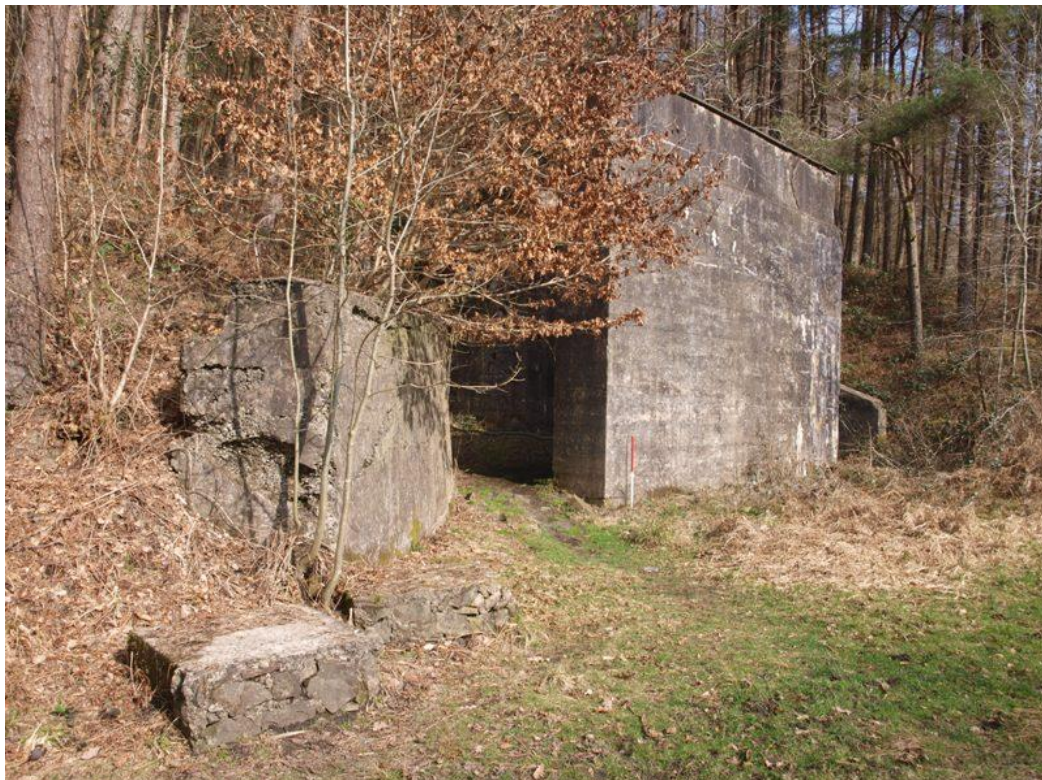
Fig. 34. New Corning House (B14). View looking north from the former junction of the Main Tramway (T1) with the Lower Tramway Branch (T7).
