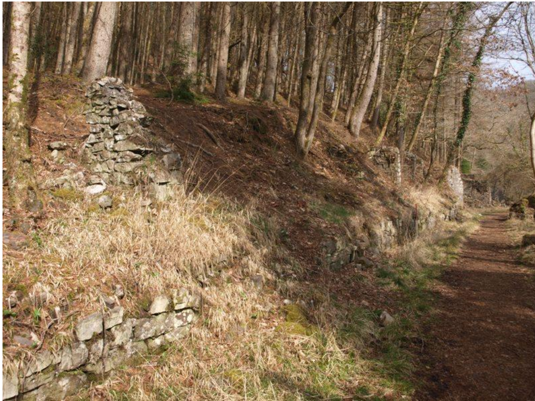
Fig. 11. Stone pillars of the Elevated Leat (W4) alongside the Main Tramway (T1).
