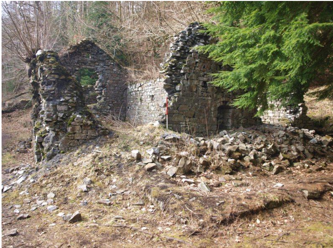
Fig. 28. Stove House (B5). View looking south, with the tramway and river to the left of the photograph. The building platform to the north – not marked on the Nobel Plan – is evident in the foreground.
