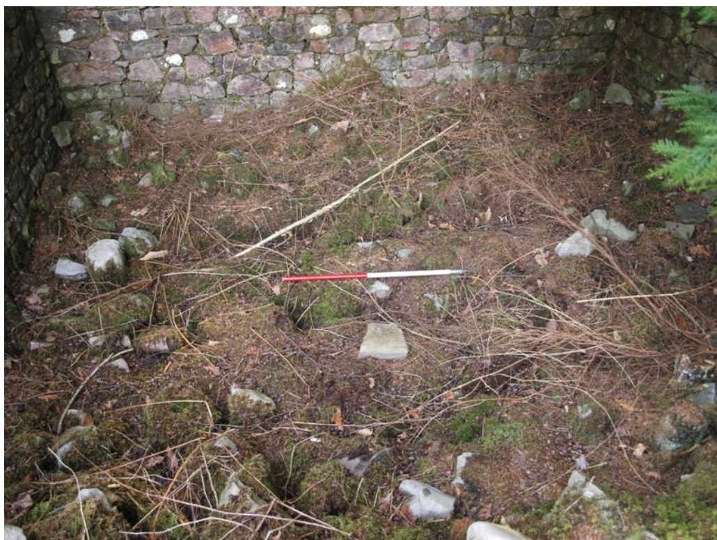
Fig. 26. Magazine (M3). Interior view showing sleeper walls and rubble.
