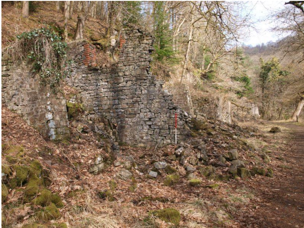
Fig. 20. The Stable (T5). View looking north along the Main Tramway (T1), showing the northern wall of the stable with brick surround to the support for the Elevated Leat (W4).
