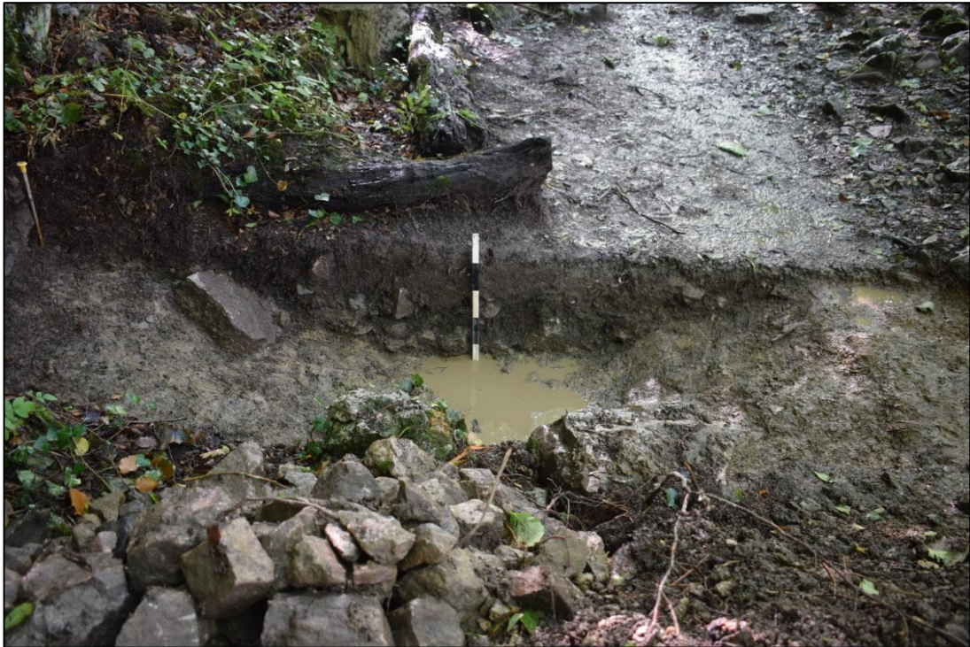
Fig. 6: The waterlogged trench clearly demonstrating that the waterproof lining of the leat was still functioning, from the north. Photo CPAT 4398-0020
