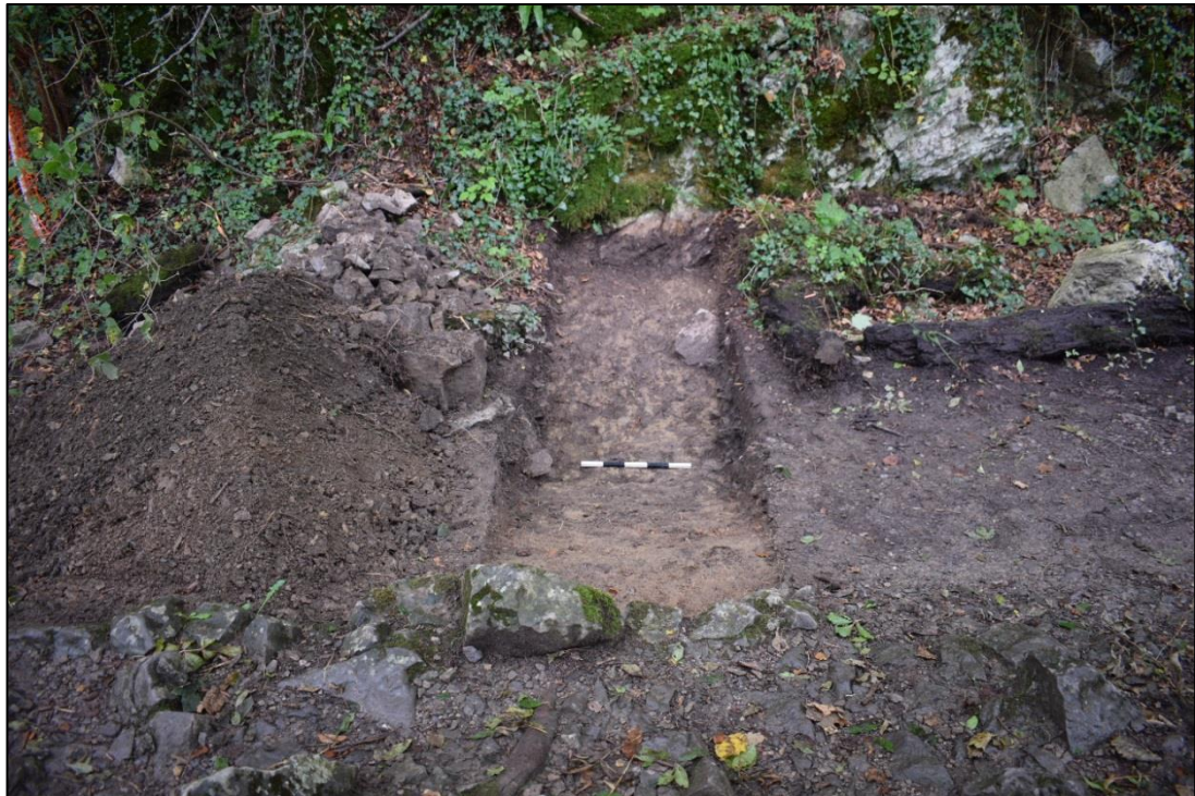
Fig. 4: The watercourse as excavated with the retaining wall in the foreground and the rock-cut scarp in the background, from the west. Photo CPAT 4398-0010
