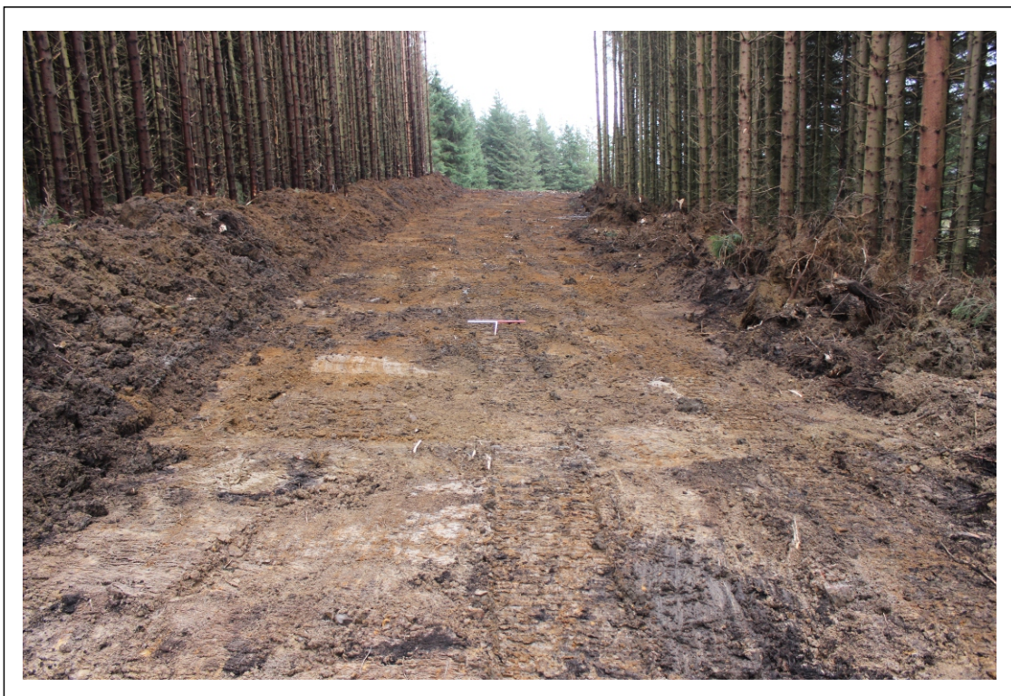
Plate 6: View east showing roadway topsoil strip and natural clay (001) through managed forest area
