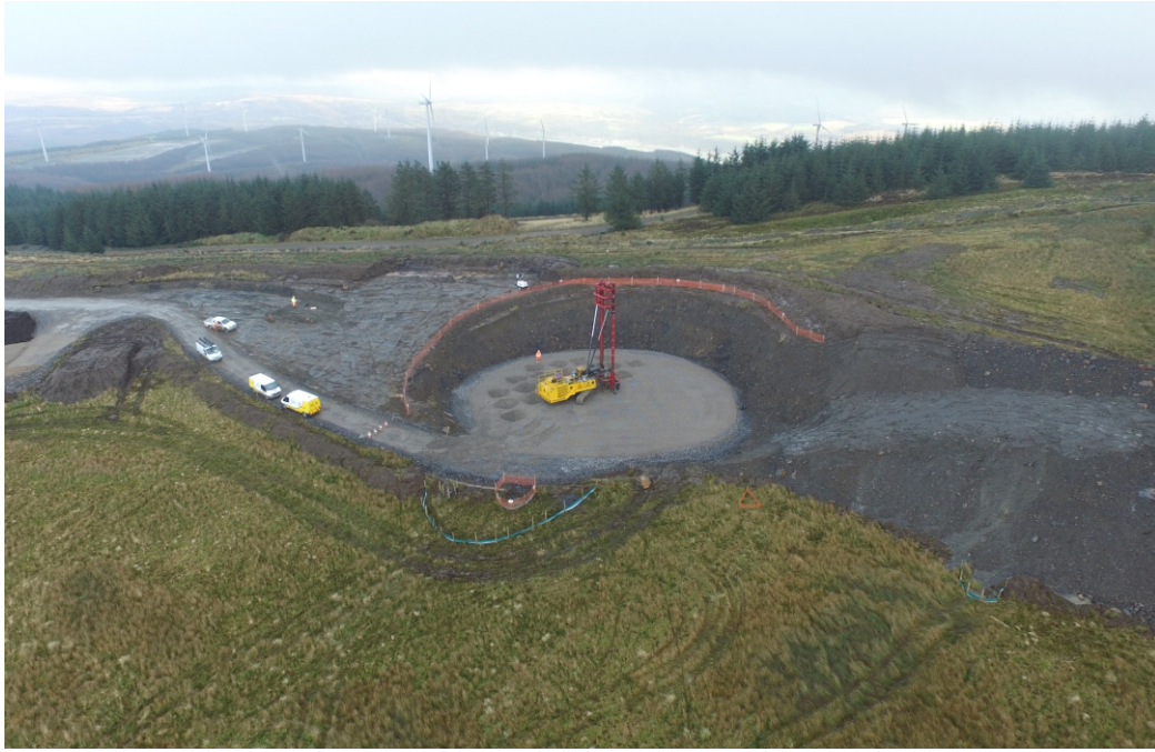
Plate 1: View of turbine foundation excavation showing (003) dark brown grey quarry tip, looking south
