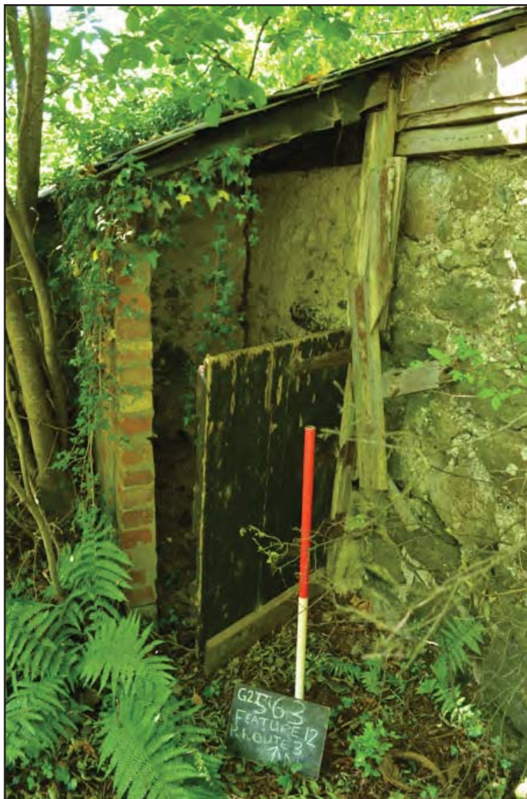
Plate 30 - Primary Reference Number: 56143. Entrance to lean to structure of Feature 12; scale: 1x1m (archive reference: G2563_077).
