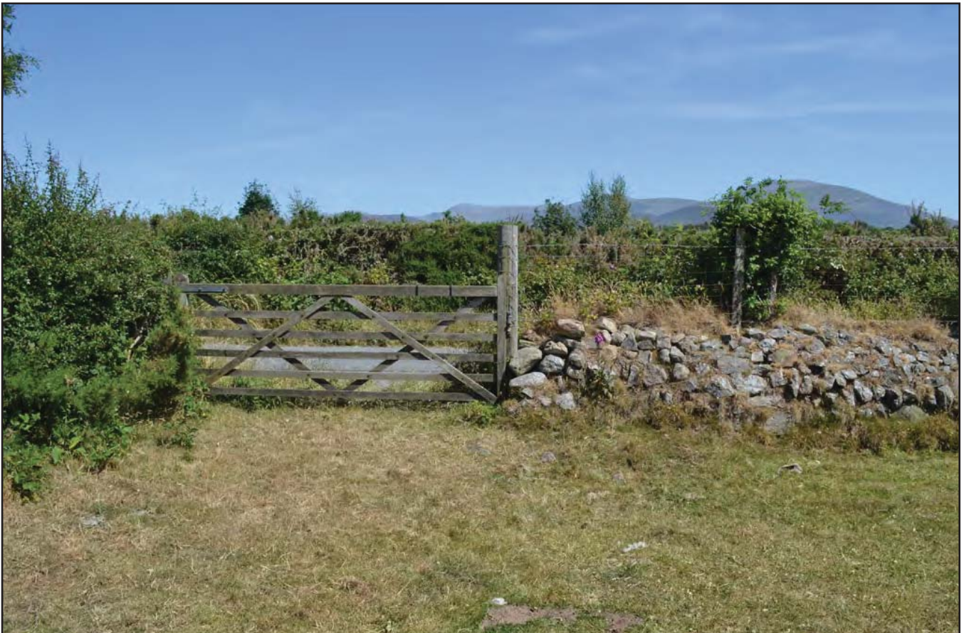
Plate 6 - Close up view of field entrance and clawdd wall field boundary on eastern side of field (archive reference: G2563_014).
