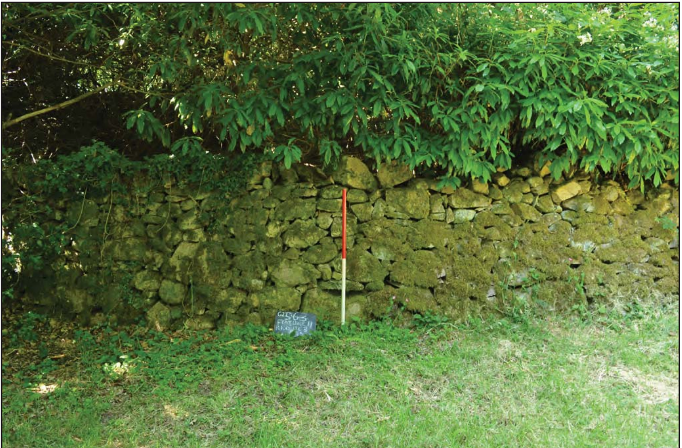
Plate 28 - Primary Reference Number: 71218. Southwest face of Feature 11, proposed pipe route 3; scale: 1x1m (archive reference: G2563_073).
