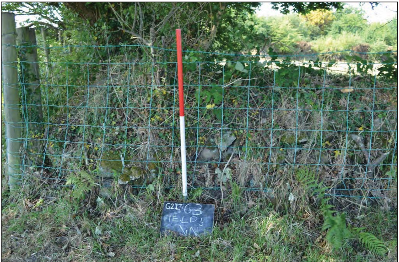
Plate 16 - Primary Reference Number: 71211. Close-up of north face of Feature 4, Field 5; scale: 1x1m (archive reference: G2563_037).
