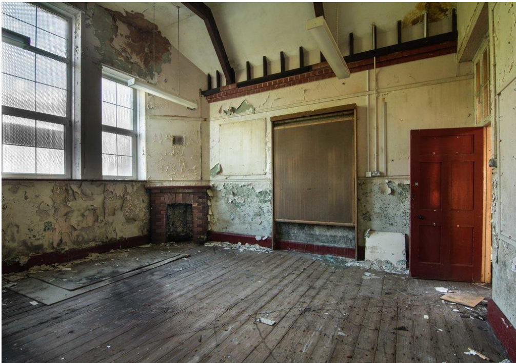
Figure 16 - classroom (showing survival of historic ceilings, doors and fireplaces)
