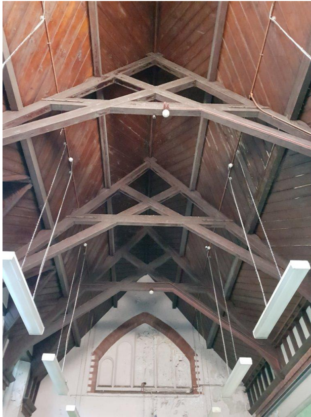
Figure 13 - open roof of original hall
