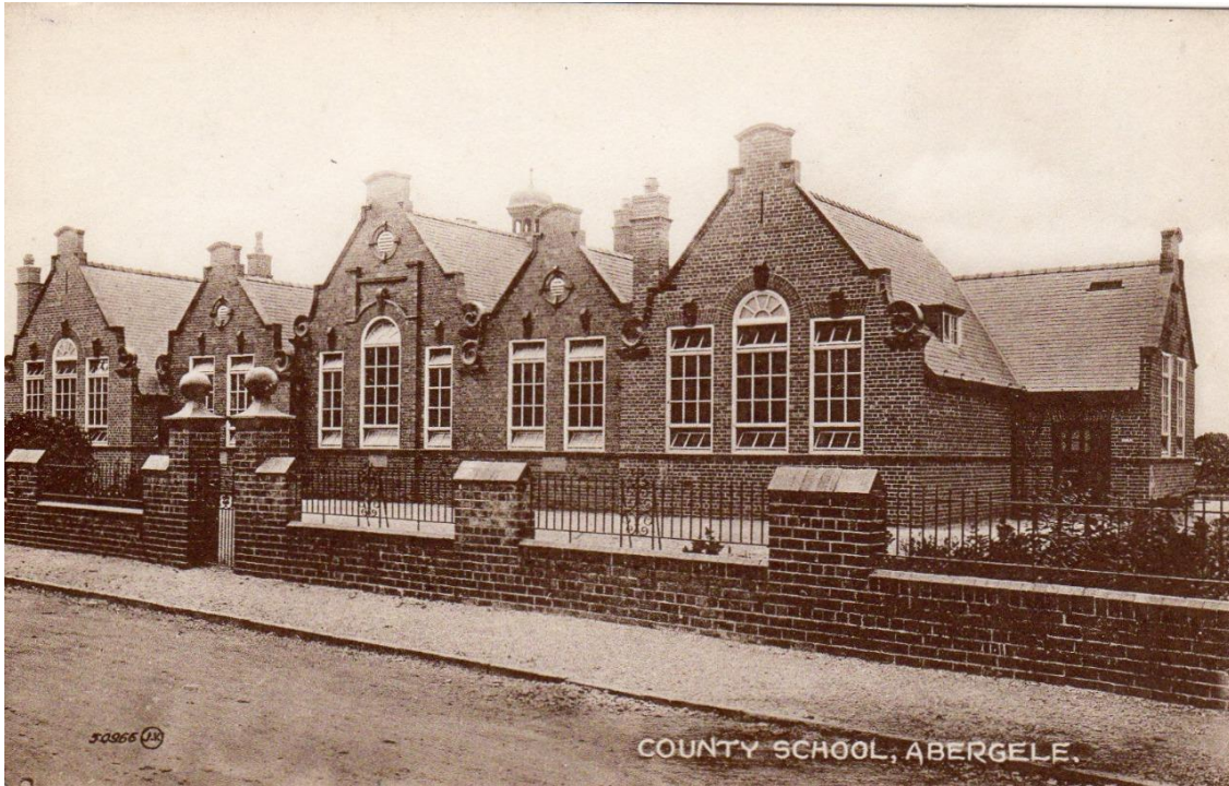
Figure 8 - Abergele Schools (Ysgol Emrys ap Iwan) built 1899
