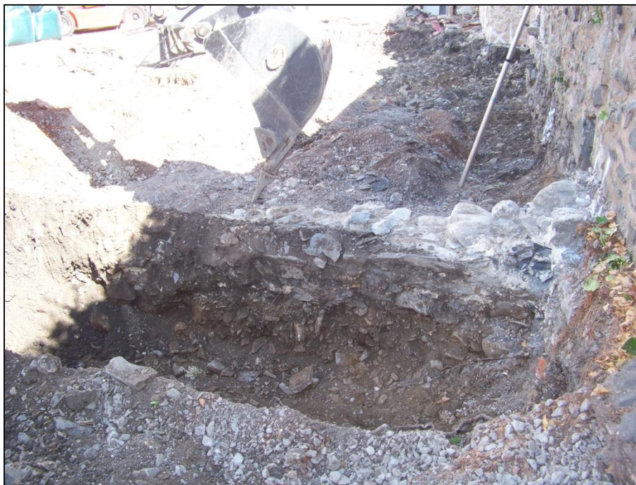
Plate 8: Exposing demolished wall foundations. 16.08.18
