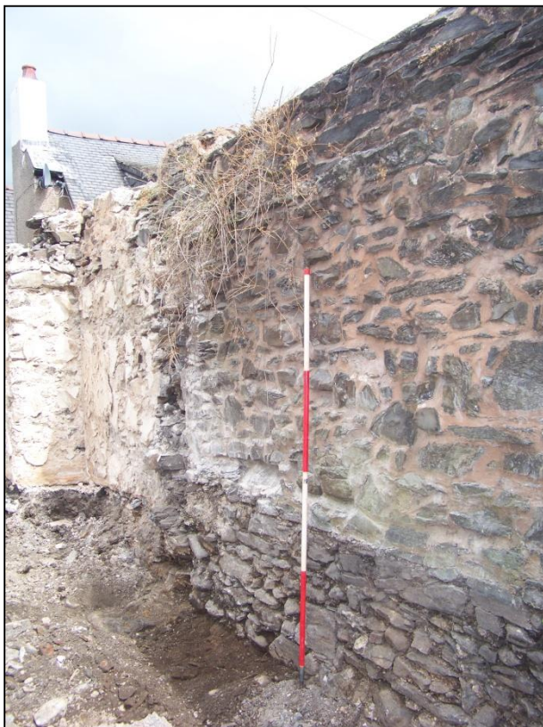
Plate 10: Looking NNE showing wall foundations resting on natural silt. 2m scale bar 17.08.18
