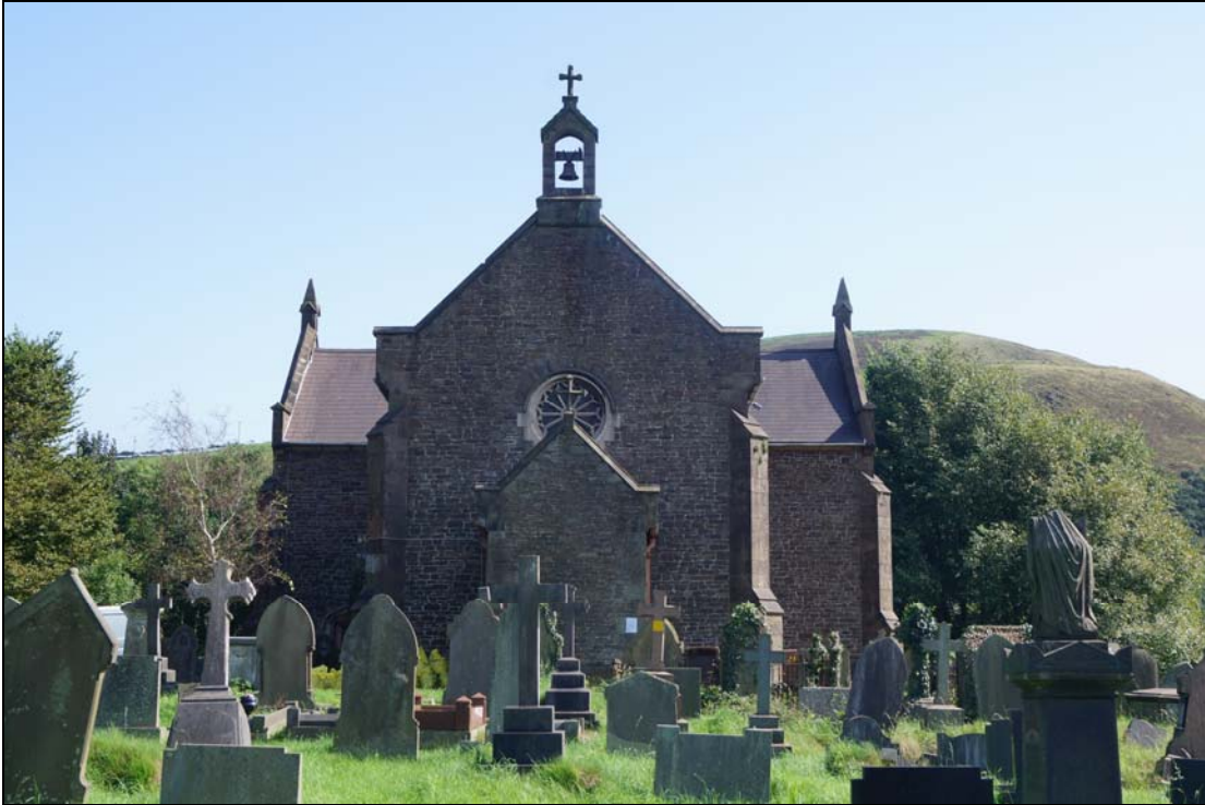
Plate 1: HCT2016_001, External view of western end of church, looking east-southeast.
