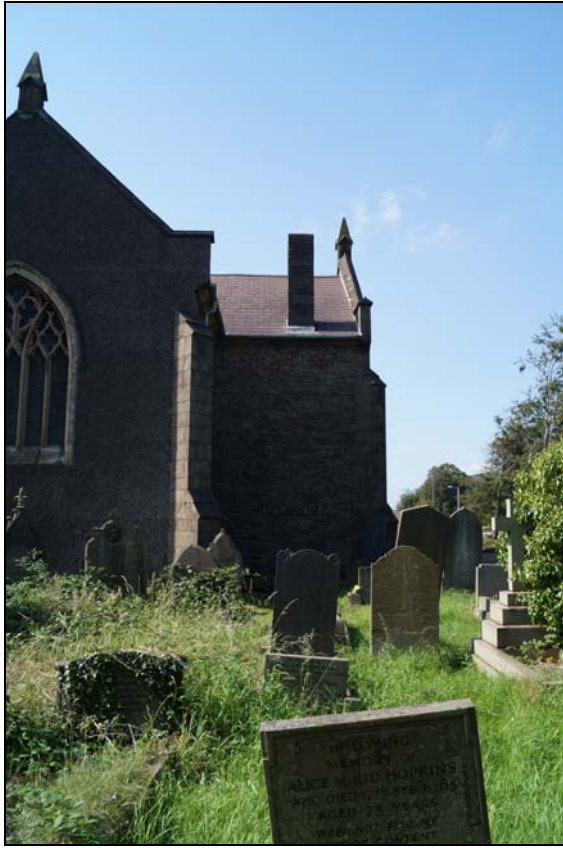
Plate 15: HCT2016_015, External view of east wall of the north transept, looking west-northwest.
