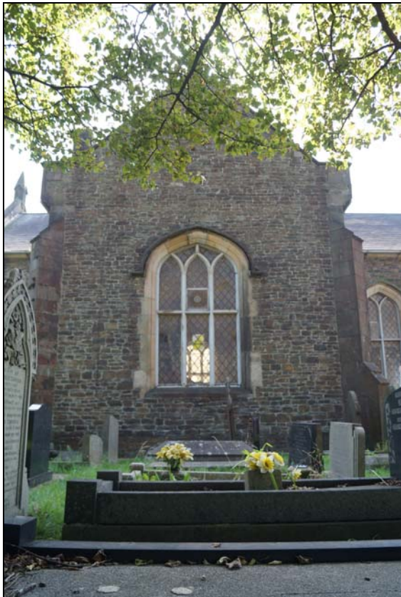
Plate 16: HCT2016_016, External view of north
