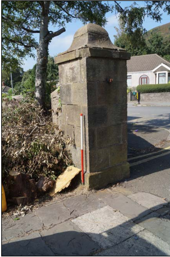
Plate 27: HCT2016_027, View of the intact western gate pillar at the entrance to the churchyard, looking north-northwest.
