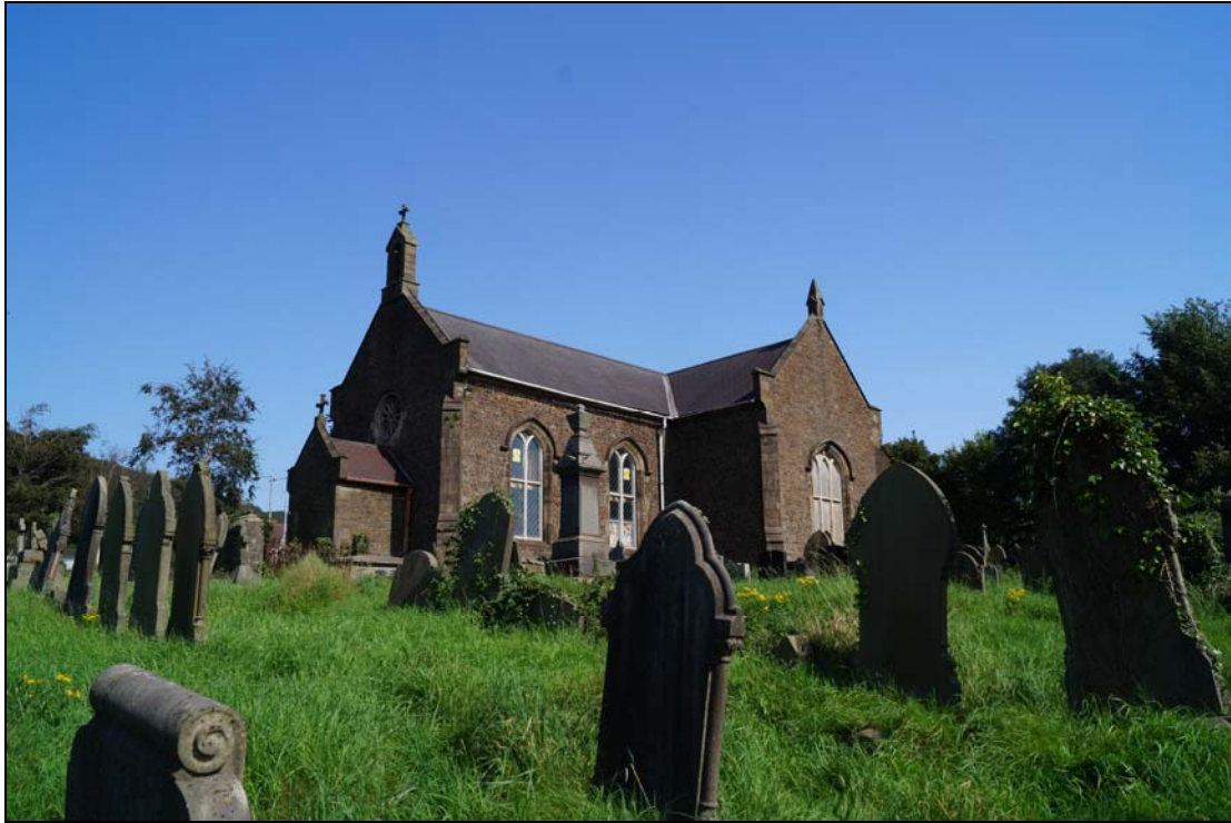
Plate 5: HCT2016_005, External view of church, looking east-northeast.
