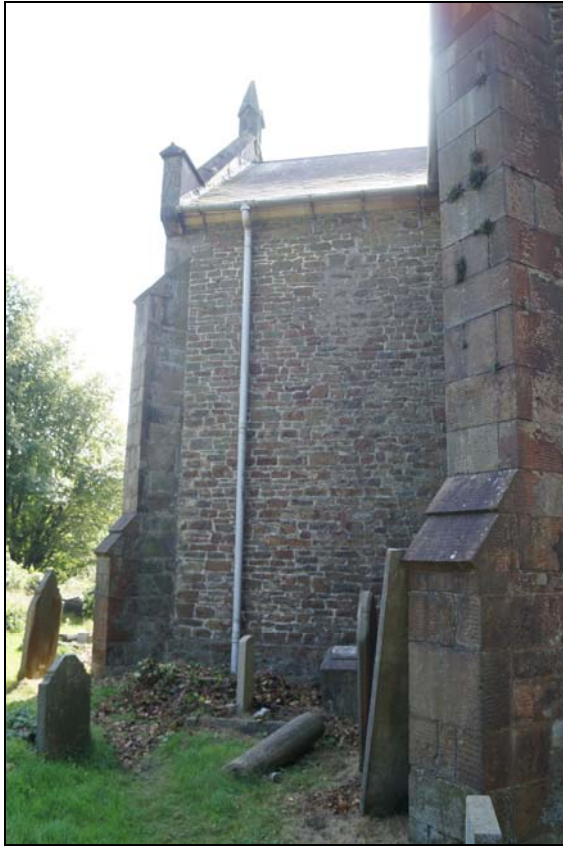
Plate 17: HCT2016_017, External view of northern chancel wall, looking south.
