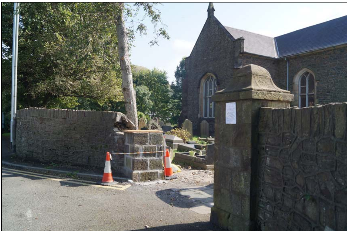
Plate 26: HCT2016_026, View of gate pillars at entrance to churchyard with the eastern pillar under reconstruction after the entrance has been widened, looking south-southeast.
