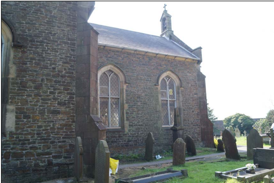
Plate 18: HCT2016_018, External view of northern side of the nave, looking west-southwest.
