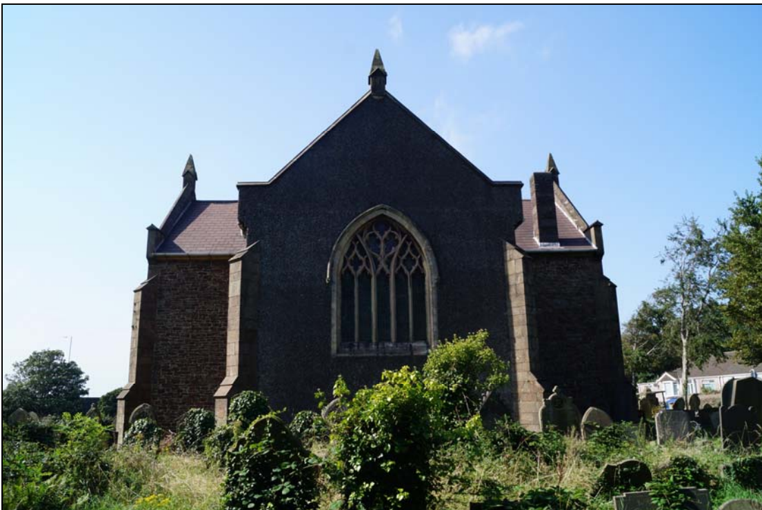
Plate 14: HCT2016_014, External view of east-southeast end of church, looking west-northwest.
