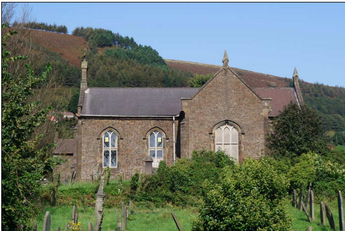
Plate 6: HCT2016_006, External view of southern side of church, looking north-northeast.
