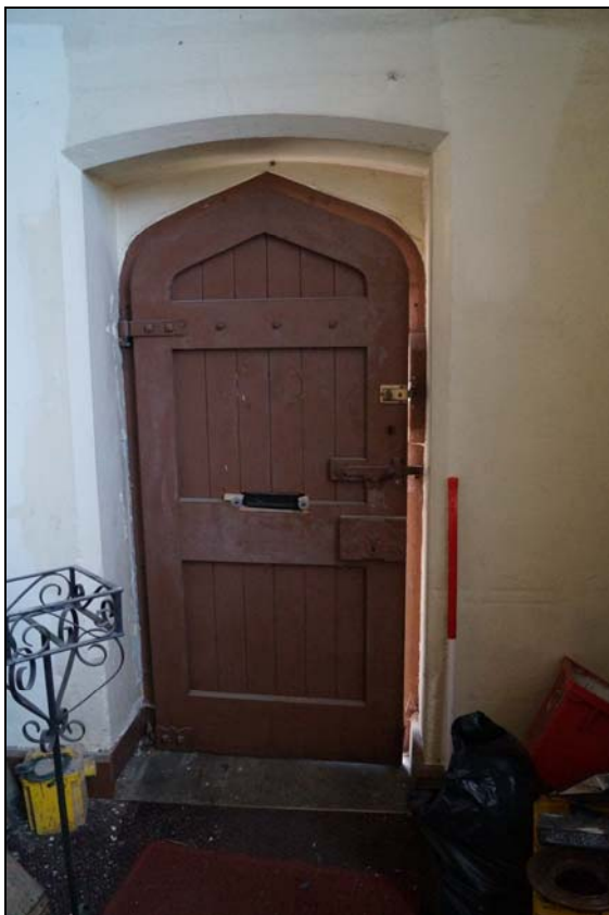
Plate 60: HCT2016_060, Internal view of vestry door in west wall of north transept, looking west-northwest.
