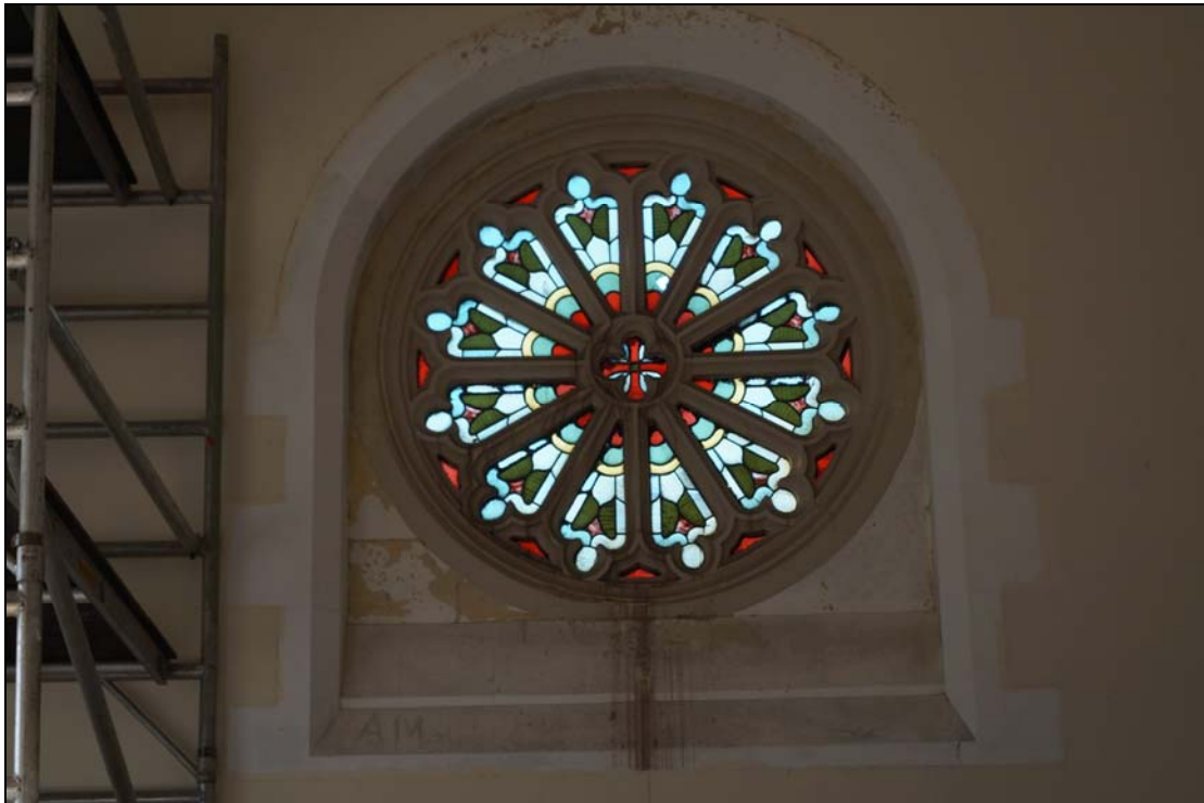
Plate 73: HCT2016_073, Internal close-up of the rose window in the west end of the nave, looking west-northwest. Taken from a stepladder.
