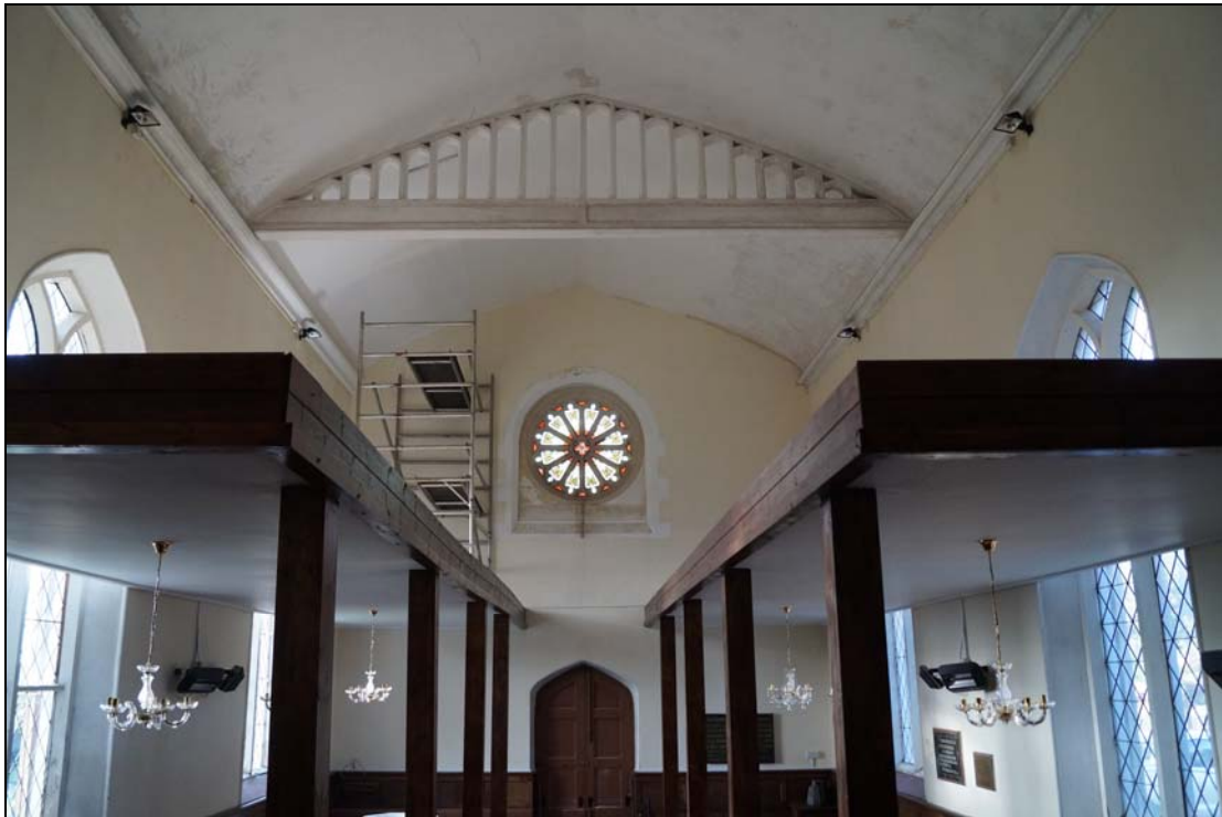
Plate 31: HCT2016_031, Internal view of the nave, showing the rose window above the main entrance, as well as the new "canopies" erected over the pews along either side of the nave. Also showing the western end of the church roof and a roof beam. Looking west-northwest. Taken from a stepladder.
