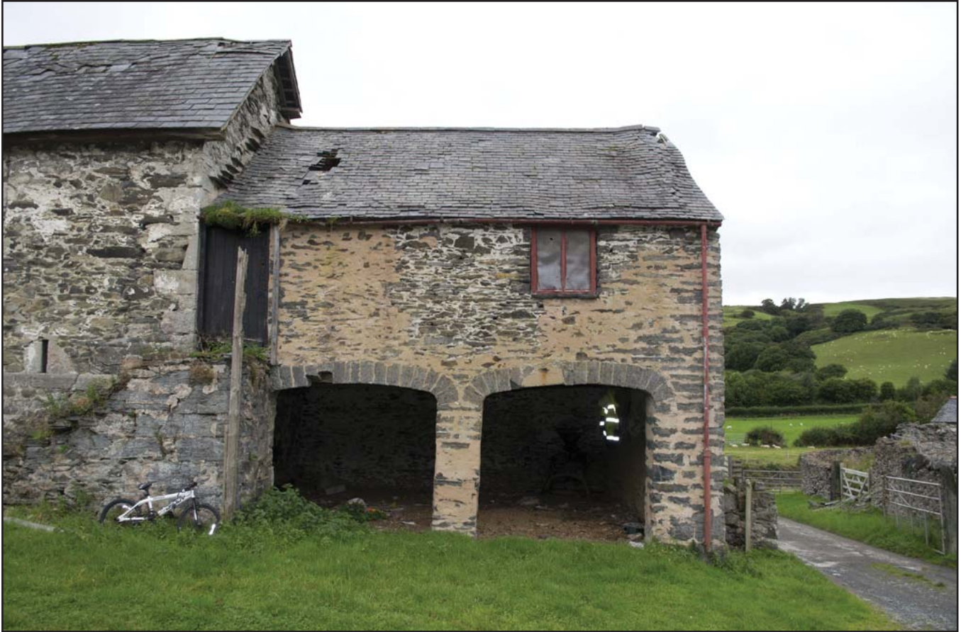
Plate 33: SE elevation of Cart Shed G04 (external) (archive reference: G2479_002).
