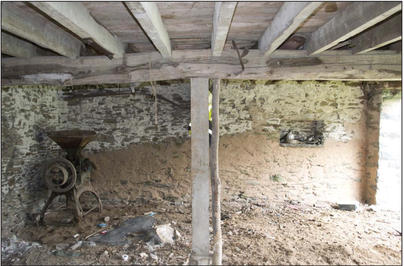
Plate 37: NE elevation Cart Shed G04 (internal) (archive reference: G2479_007).
