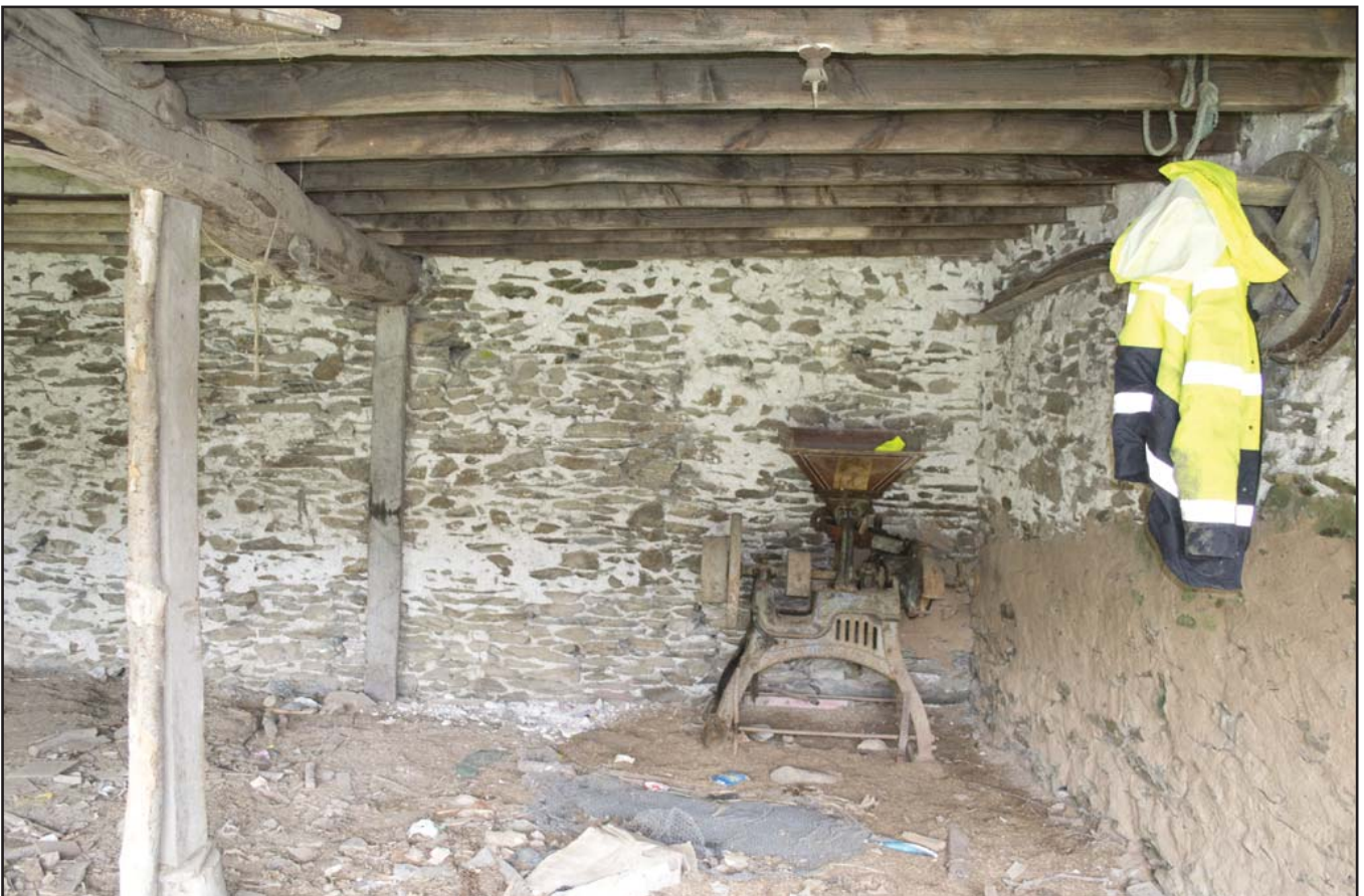
Plate 36: NW elevation of Cart Shed G04 (internal) (archive reference: G2479_008).
