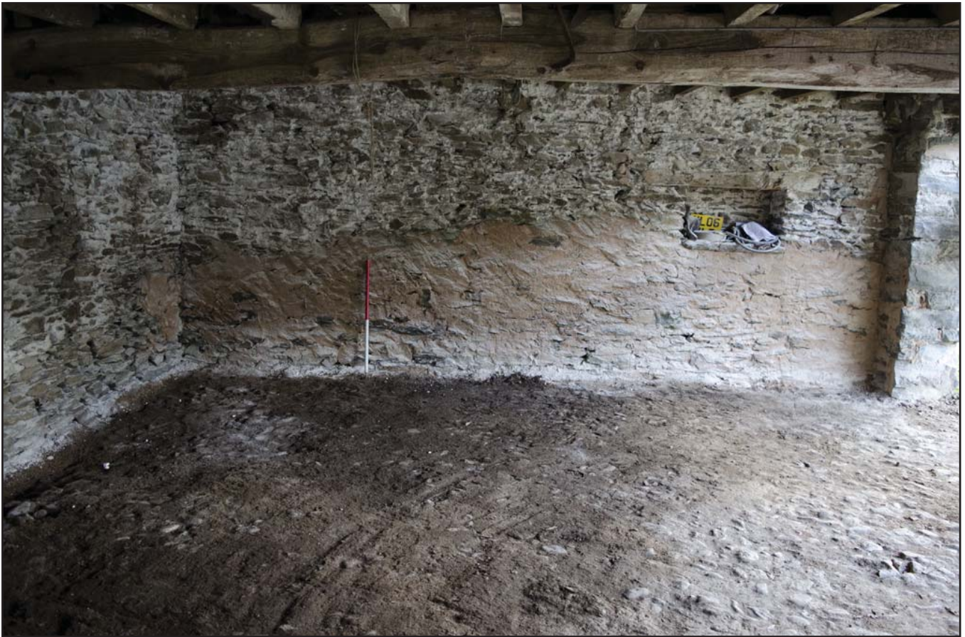
Plate 63: N wall and cobbled floor in Cart Shed G04; scale: 1x1 m (archive reference: G2479_100).
