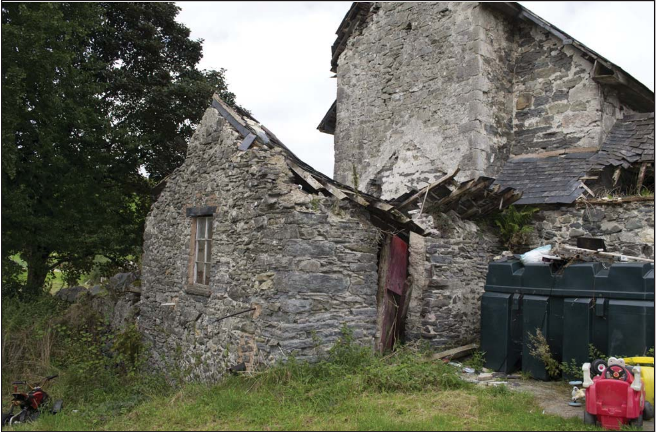
Plate 3: SW/SE elevation of Outbuilding G03 (archive reference: G2479_026).
