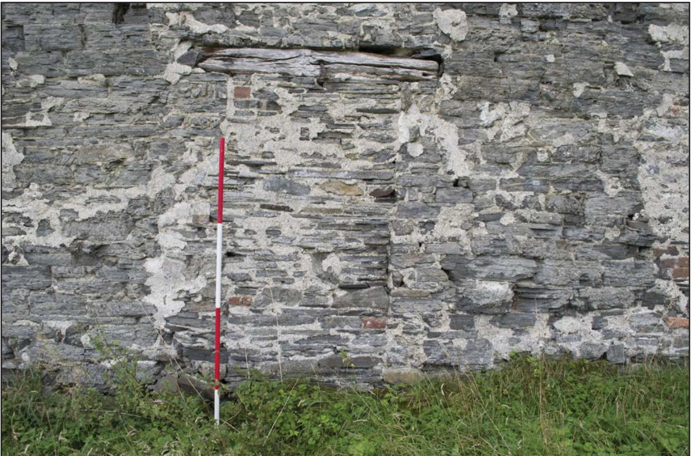
Plate 16: Blocked doorway in NW elevation of G01/F01 with butt joint either side; scale: 1x2m (archive reference: G2479_048).
