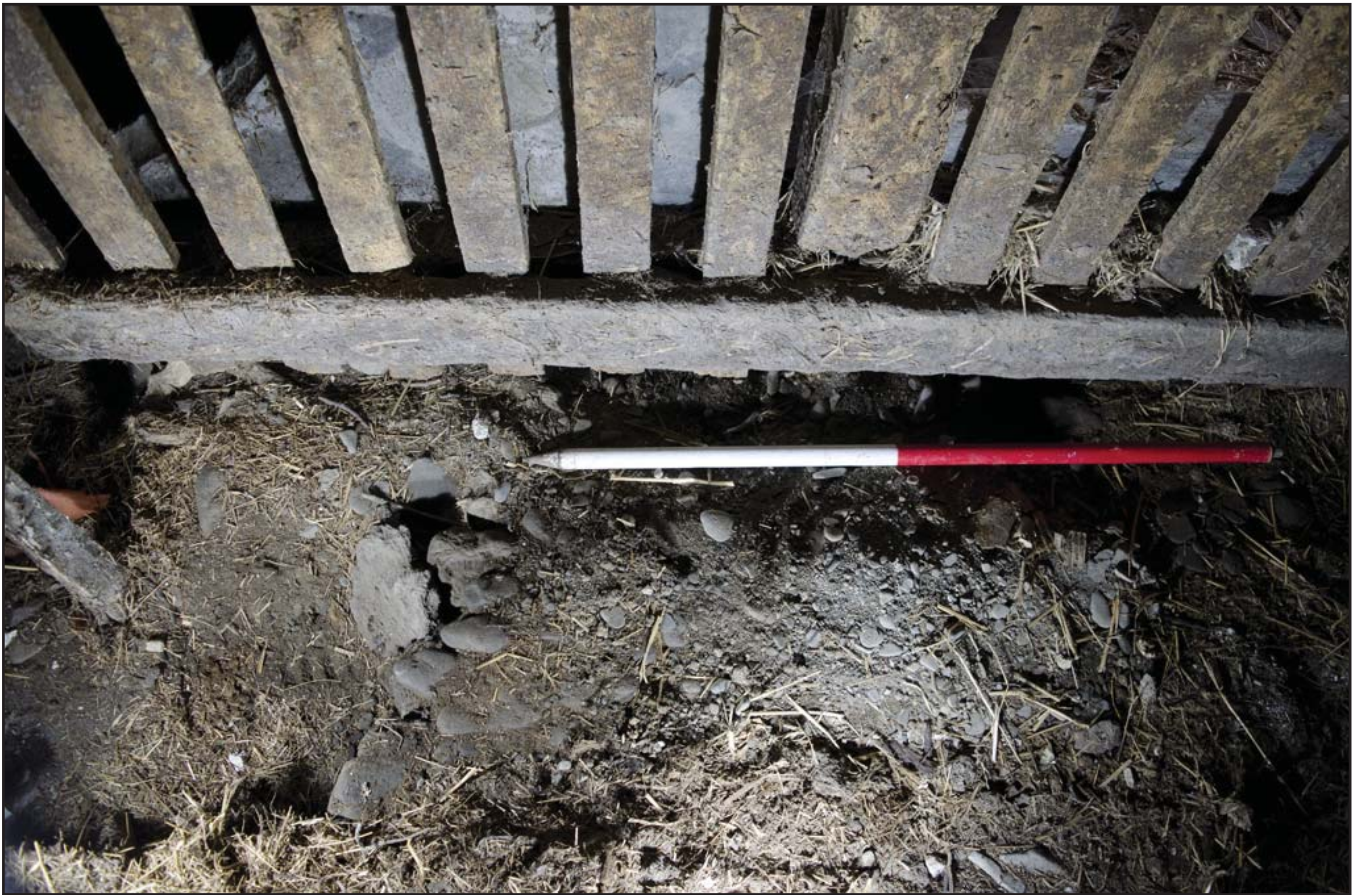
Plate 29: Cobbled floor remains in Loose box in G01 Stables; scale: 1x1m (archive reference: G2479_141).
