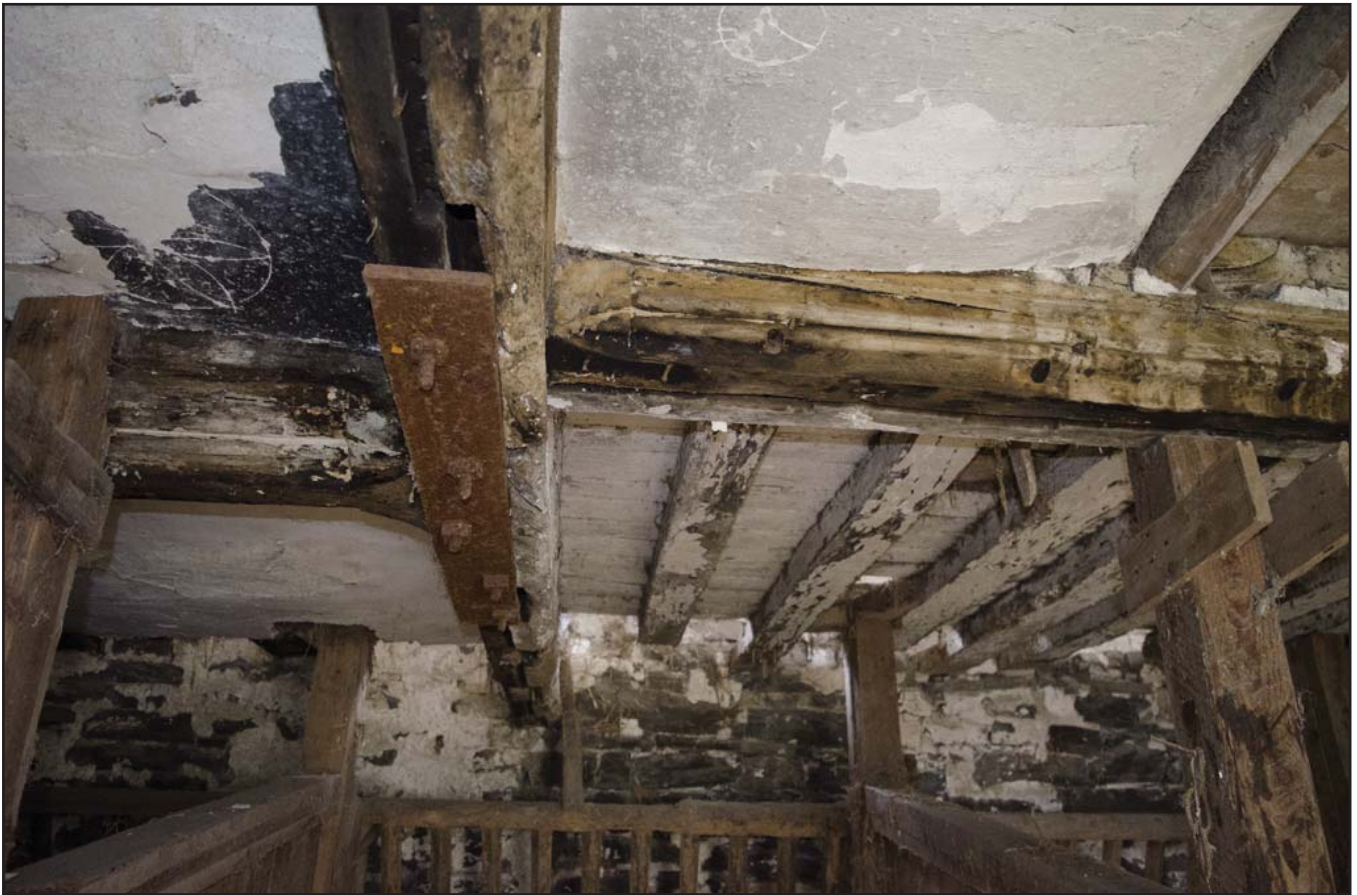
Plate 27: Roof; scale: (archive reference: G2479_177).
