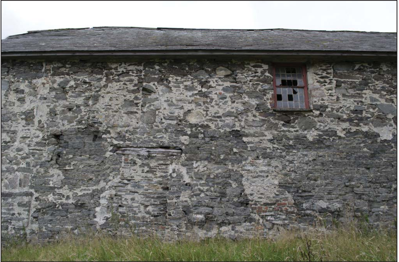
Plate 15: NW wall of G01/F01 showing complex phasing (archive reference: G2479_041).
