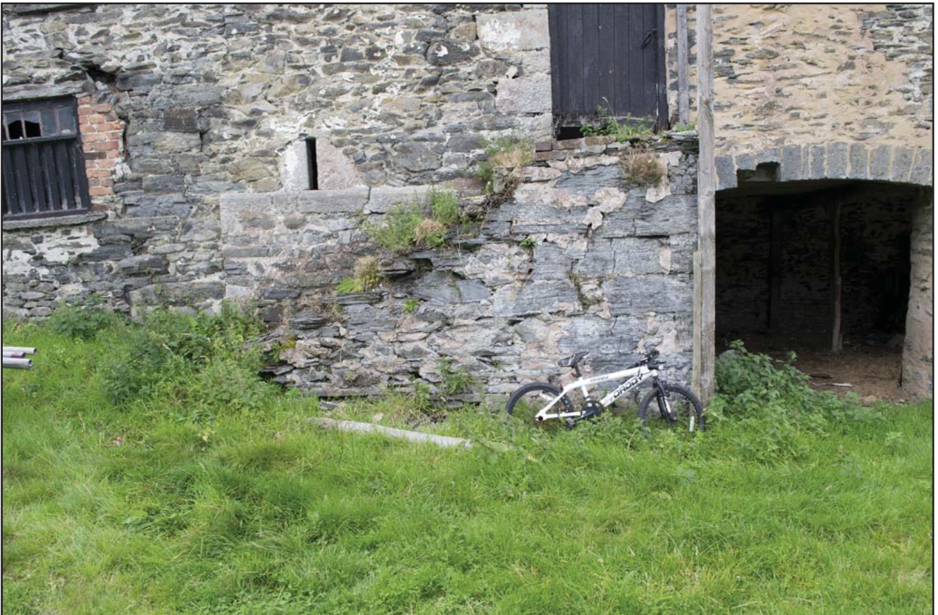
Plate 54: External staircase to Grain Store F04 (archive reference: G2479_028).
