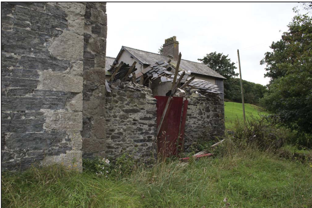
Plate 32: North elevation of Outbuilding G03 (archive reference: G2479_027).
