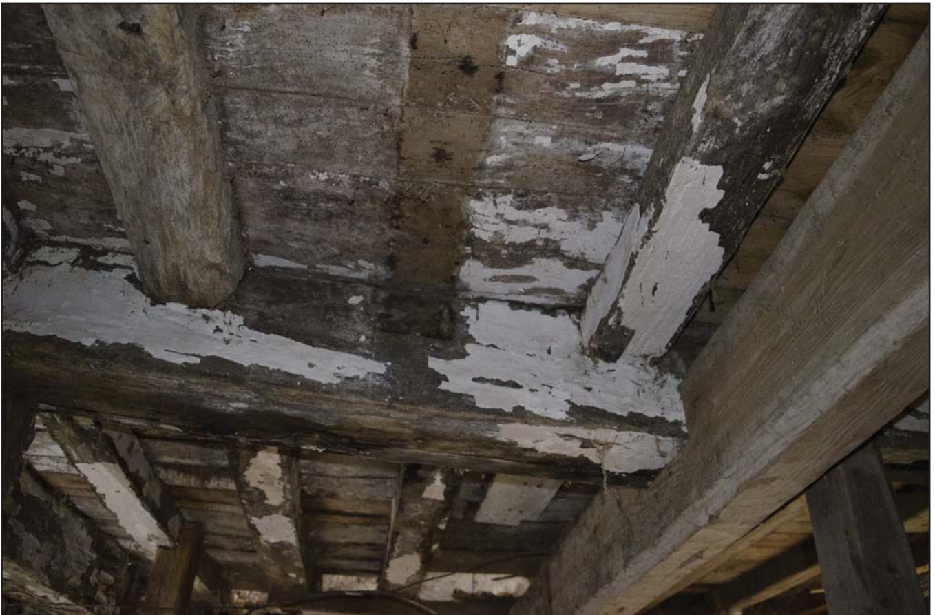
Plate 26: Roof; scale: (archive reference: G2479_180).
