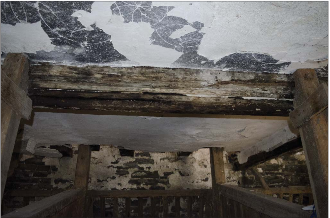
Plate 25: Roof; scale: (archive reference: G2479_176).
