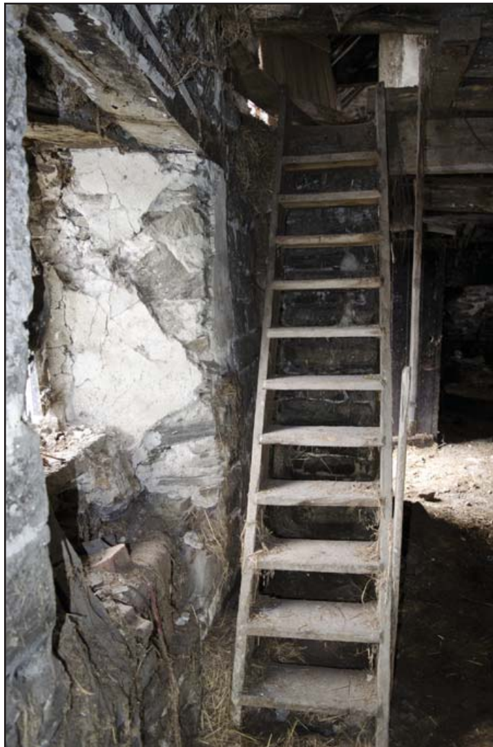
Plate 24: Stairs up to Hayloft F01 from Stables G01 (archive reference: G2479_191).
