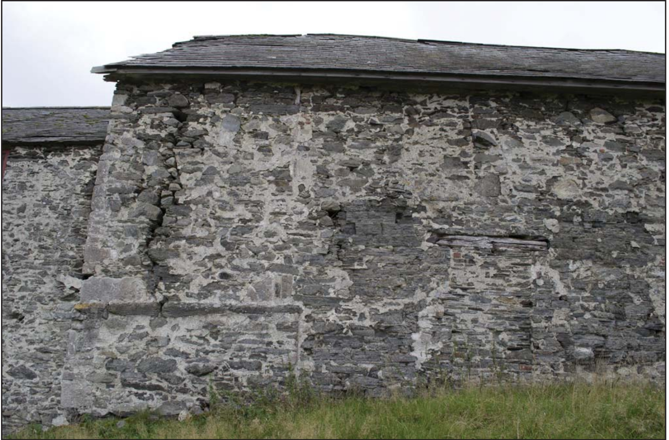
Plate 17: NW wall of G01/F01 showing complex phasing (archive reference: G2479_040).
