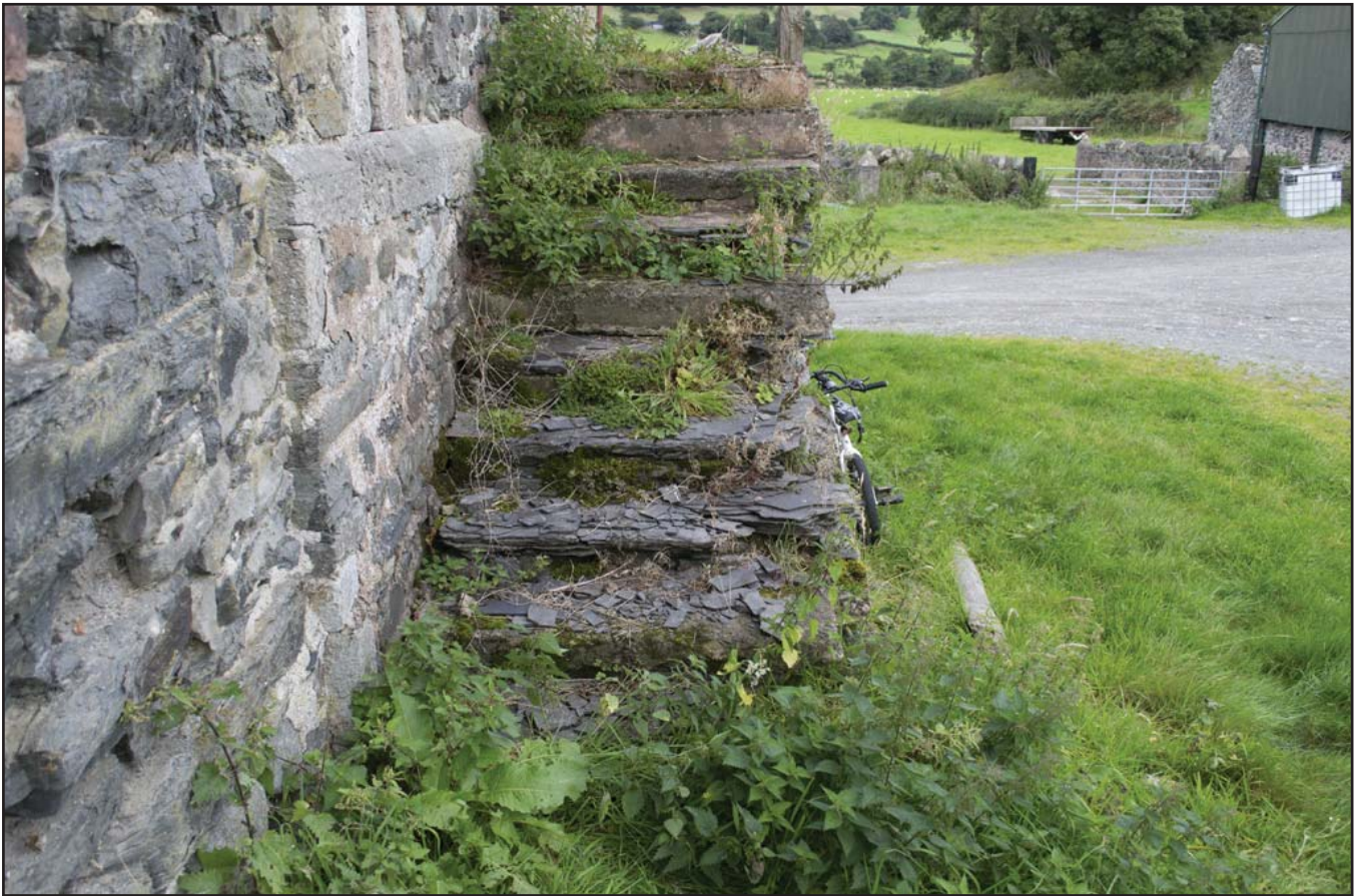
Plate 13: External staircase to Grain Store F04 (archive reference: G2479_029).
