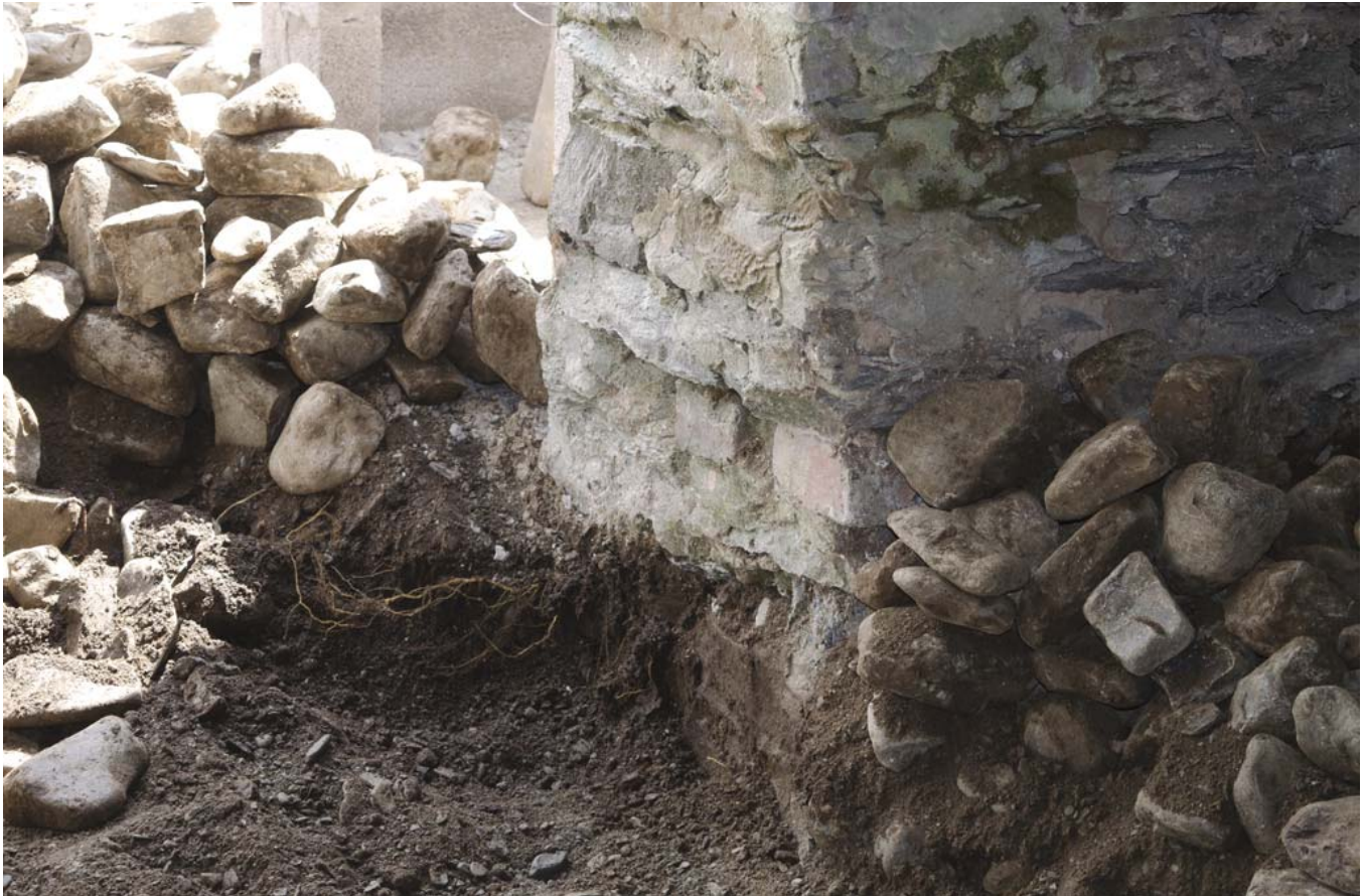
Plate 71: Cobbles lifted on S side of G04 Cart Shed showing base of wall of G04 Cart Shed (archive reference: G2479_217).
