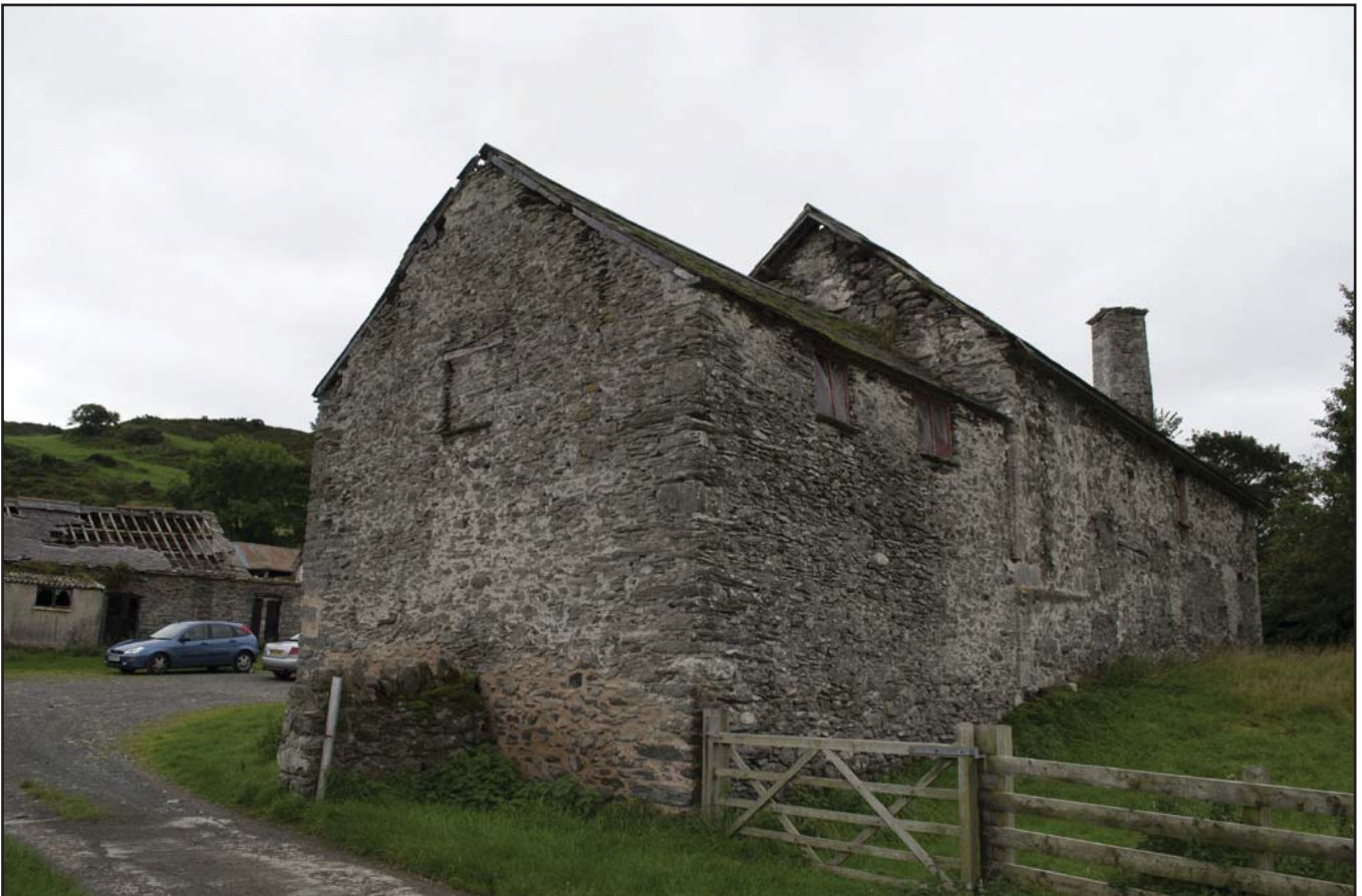
Plate 14: NE elevation Cart Shed G04 (external) (archive reference: G2479_005).
