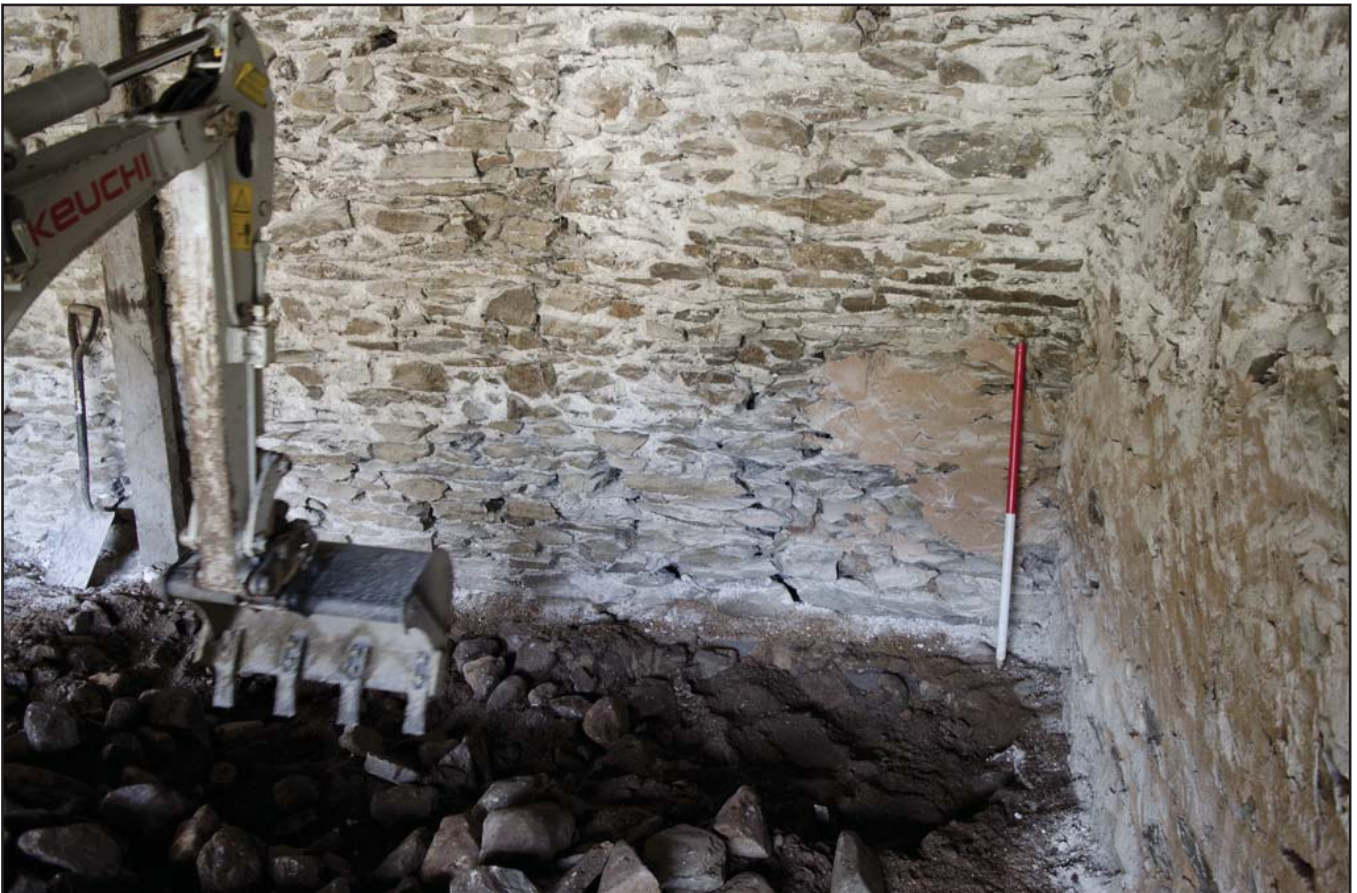
Plate 66: Lifting of Cobbles in NW corner of G04 Cart Shed; scale: 1x1m (archive reference: G2479_196).
