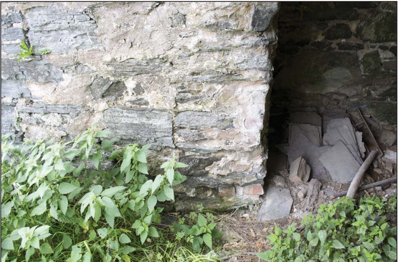
Plate 38: Butt joint between Cart Shed G04 and external access stairs, bricks visible at base of wall (archive reference: G2479_011).
