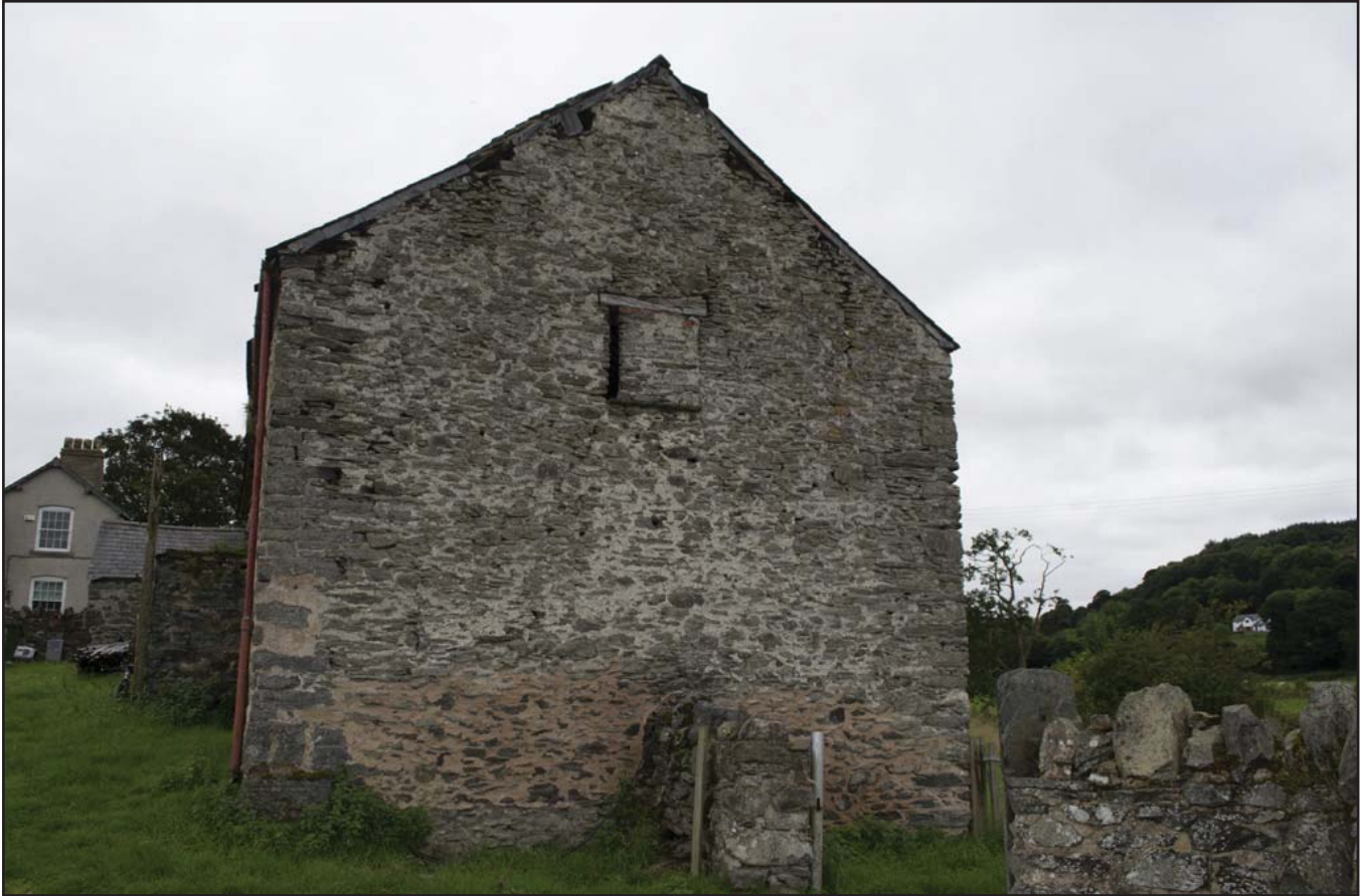
Plate 1: NE elevation Cart Shed G04 (external) (archive reference: G2479_004).
