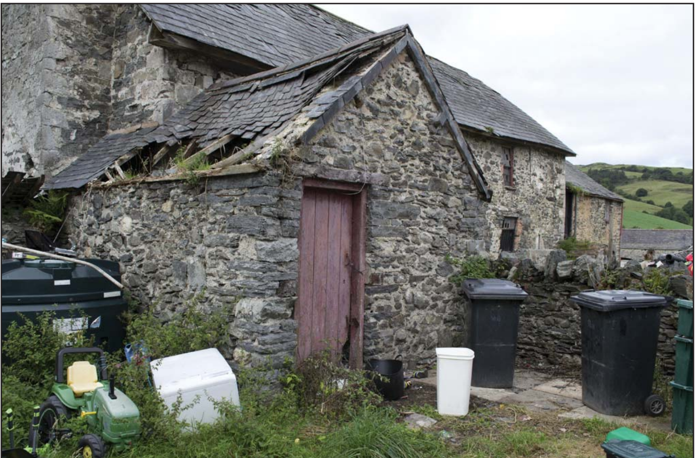
Plate 30: SW/SE elevation of Outbuilding G02 (archive reference: G2479_025).
