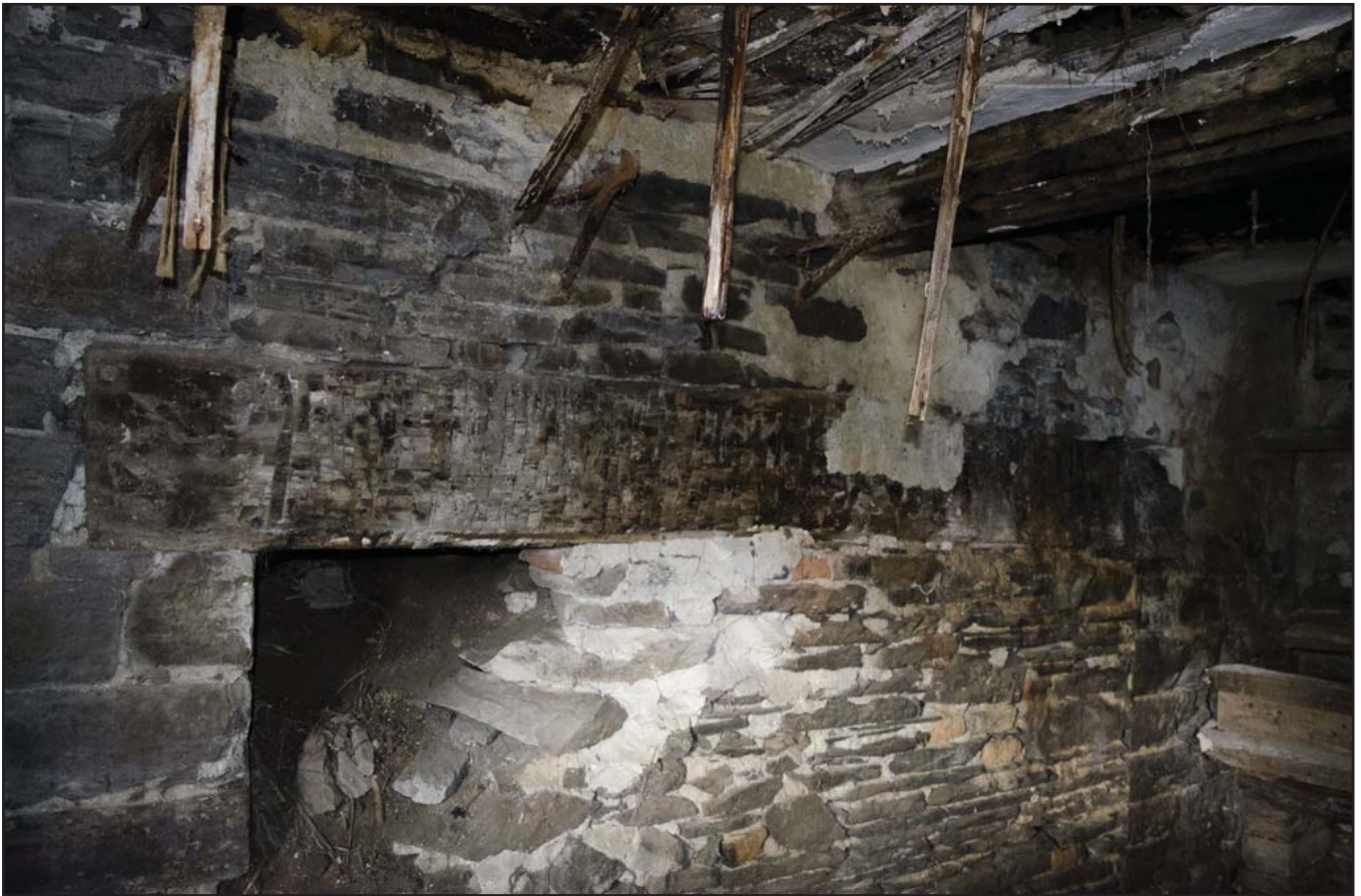
Plate 19: Fireplace Lintel; scale: (archive reference: G2479_189).
