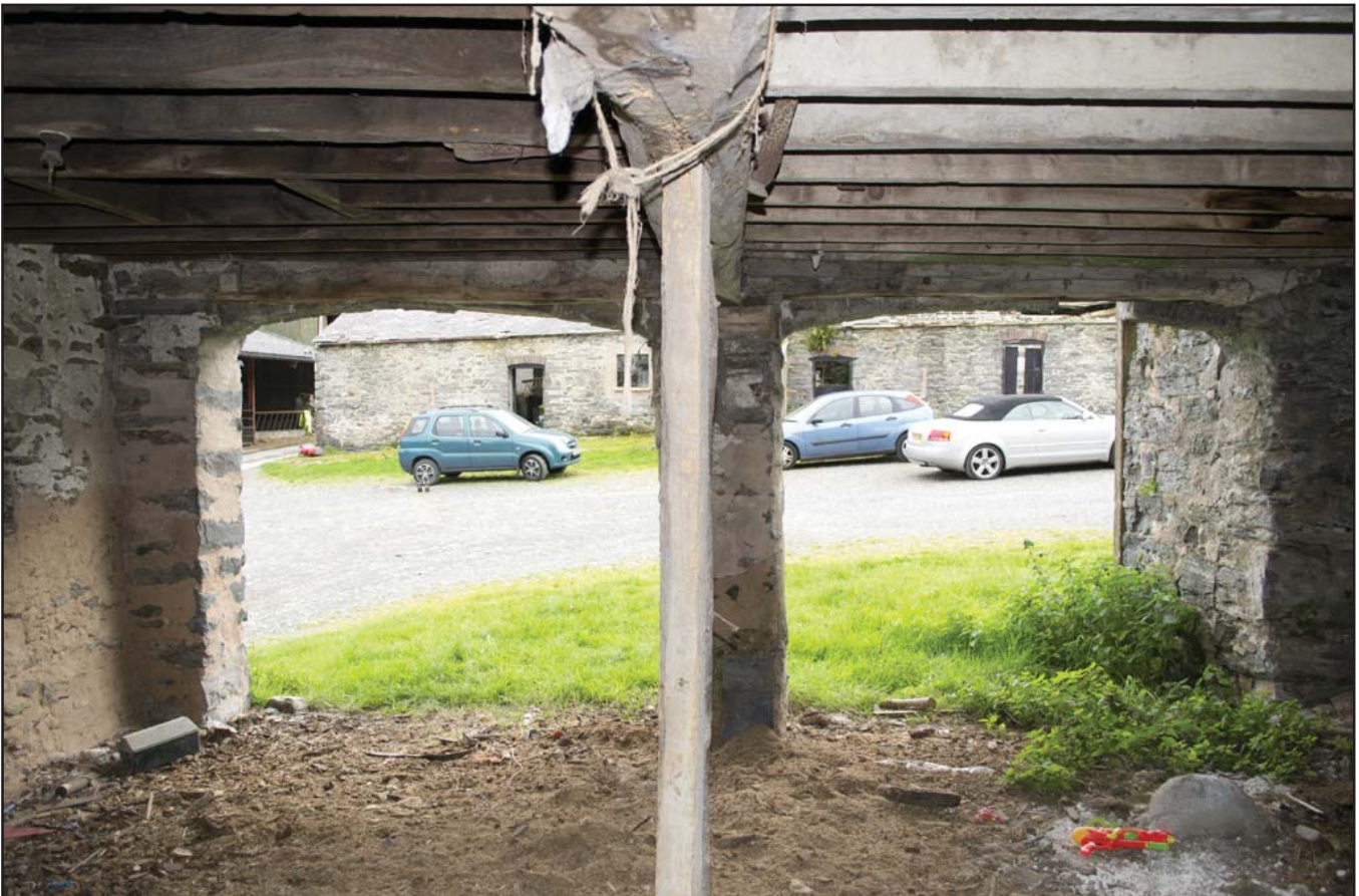
Plate 34: SE elevation of Cart Shed G04 (internal) (archive reference: G2479_013).
