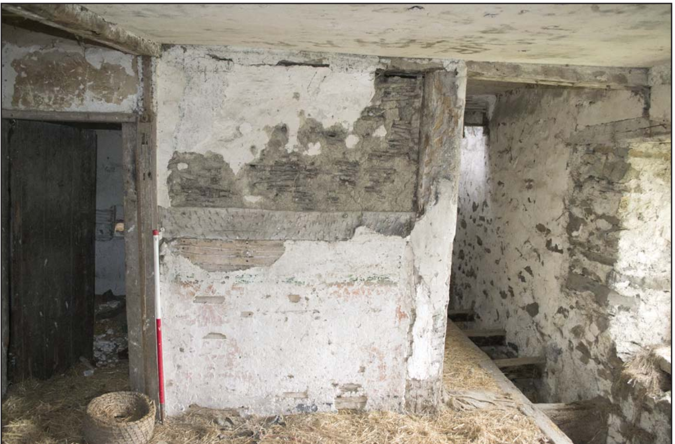
Plate 44: Decorative plasterwork - upper and lower panels - F01 Hayloft / F03 Store; scale: 1x1m (archive reference: G2479_081).
