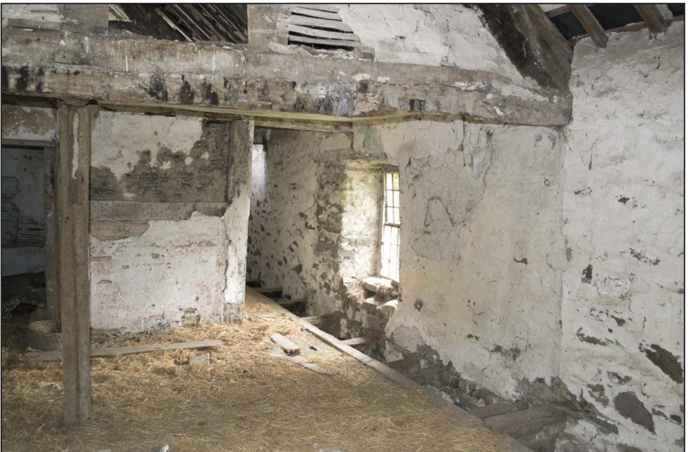
Plate 42: Partition with plasterwork, S corner F01 Hayloft (archive reference: G2479_076).
