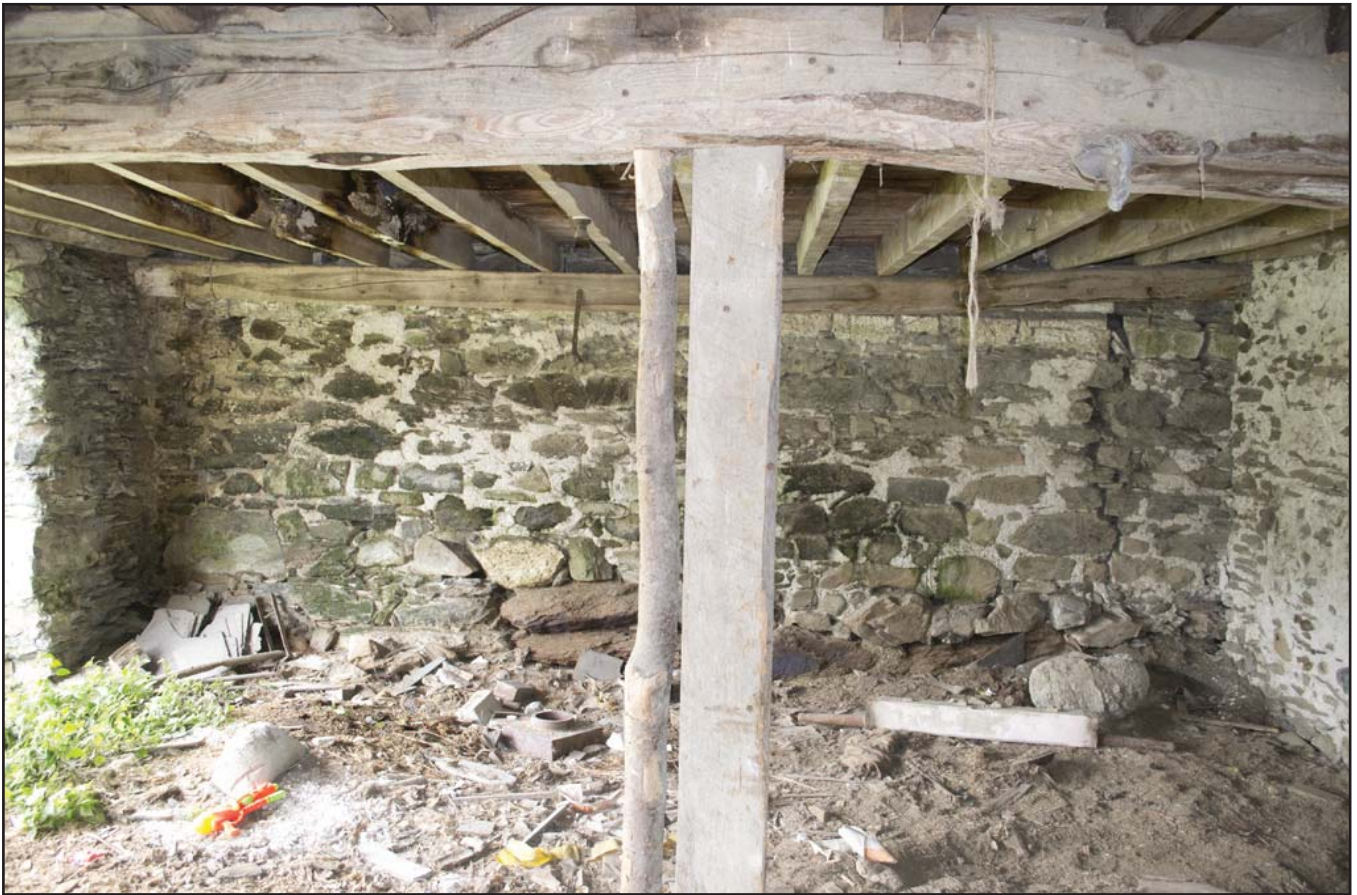
Plate 35: SW elevation of Cart Shed G04 (internal) (archive reference: G2479_010).
