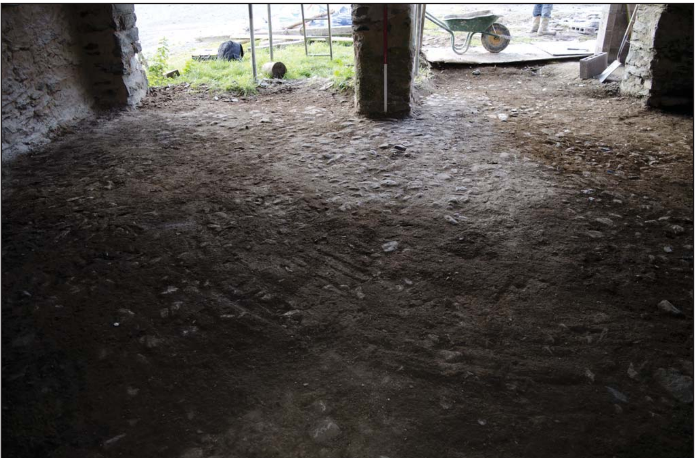
Plate 64: E opening and cobbled floor in Cart Shed G04; scale: 1x1 m (archive reference: G2479_101).
