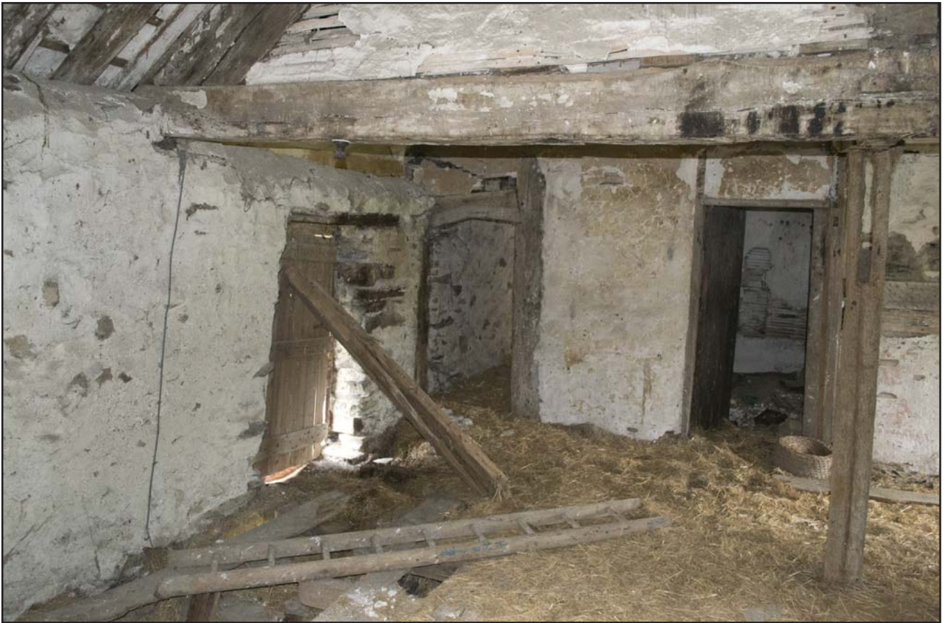
Plate 41: Partition with plater work, N corner F01 Hayloft (archive reference: G2479_075).
