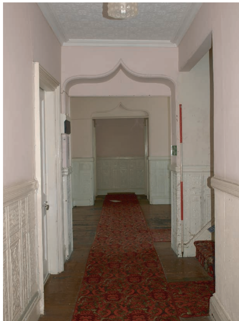
Plate No. 176: Derwen Fawr (Internal) - First floor. Series of two depressed 'ogee' arches on first floor corridor. Looking south.
