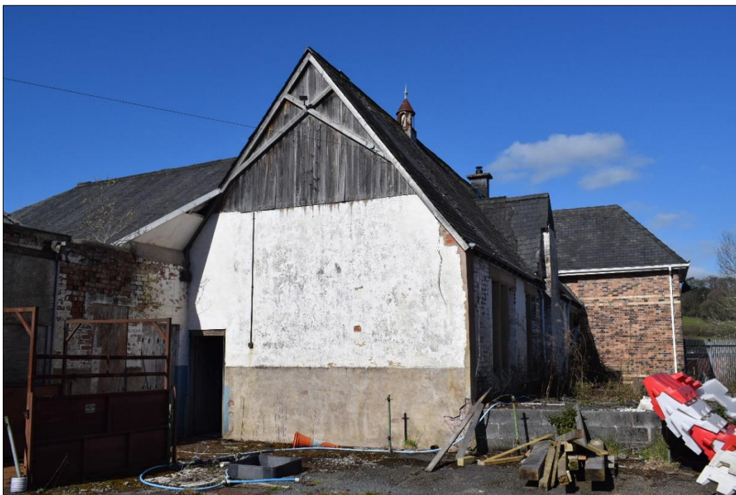
Fig. 4 The east elevation of the original building. Photo CPAT 4634-0003
