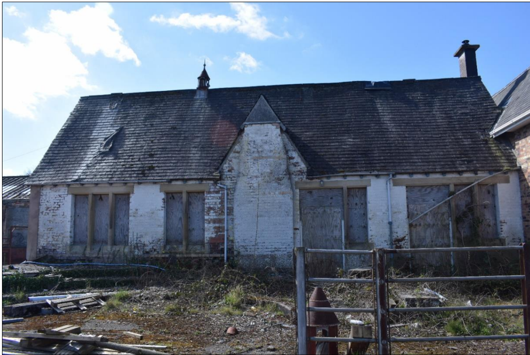
Fig. 3 The north elevation of the original building. Photo CPAT 4634-0023
