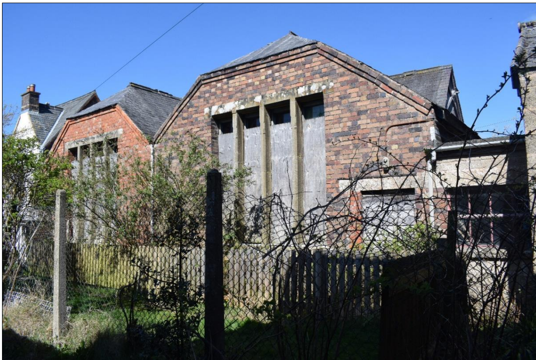
Fig. 8 The south elevation of the later classrooms. Photo CPAT 4634-0027
