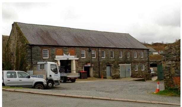
Fig 39 The two-storey Glandinorwig writing-slate mill, a grade II\* listed building under its modern name Felin Sarn. The upper storey is faced in rock-faced stone, above the random rubble of the lower storey.
