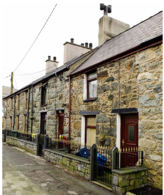
Fig 18 Houses in Tabernacle Street. The house on the right is built of random rubble stone, the later houses further left of quarried stone roughly shaped into blocks. All openings are under lintels of slate blocks. The snecked-stone garden walls are later. Originally the houses opened directly on to the street.
