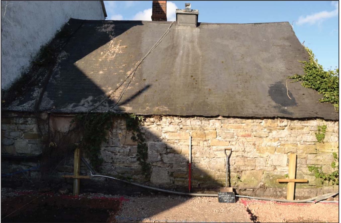
Plate 11: East face of outbuilding with tar pitched roof; scale: 1x1m (archive reference: G2602_017).
