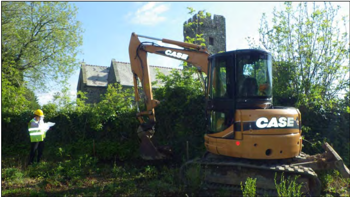
Plate 11: RWH2013_111 Beginning excavation of the trench, looking southeast.
