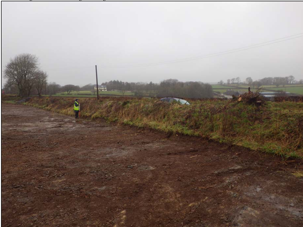
Plate 6: TNB2015_106: Eastern side of the development area, boundary bank to be breached for access, looking north northeast
