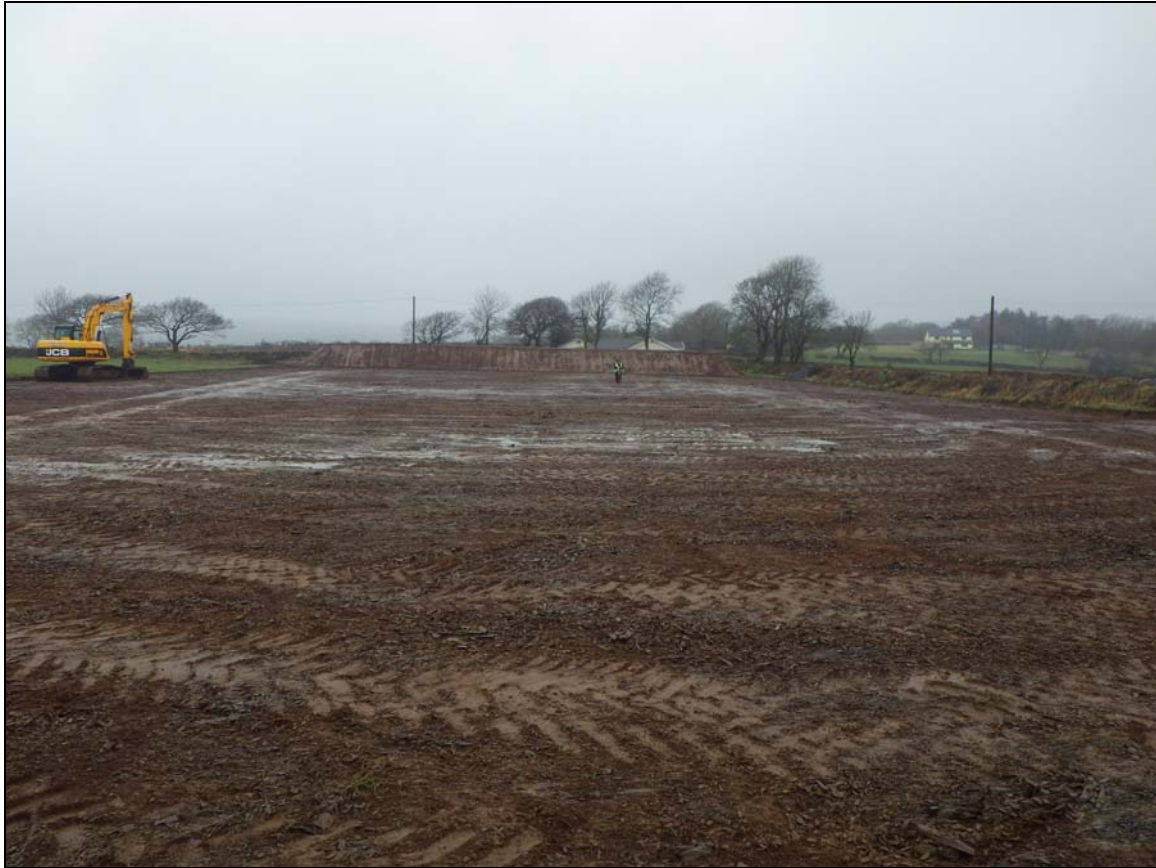
Plate 7: TNB2015_107: Development area fully stripped, looking north northwest.
