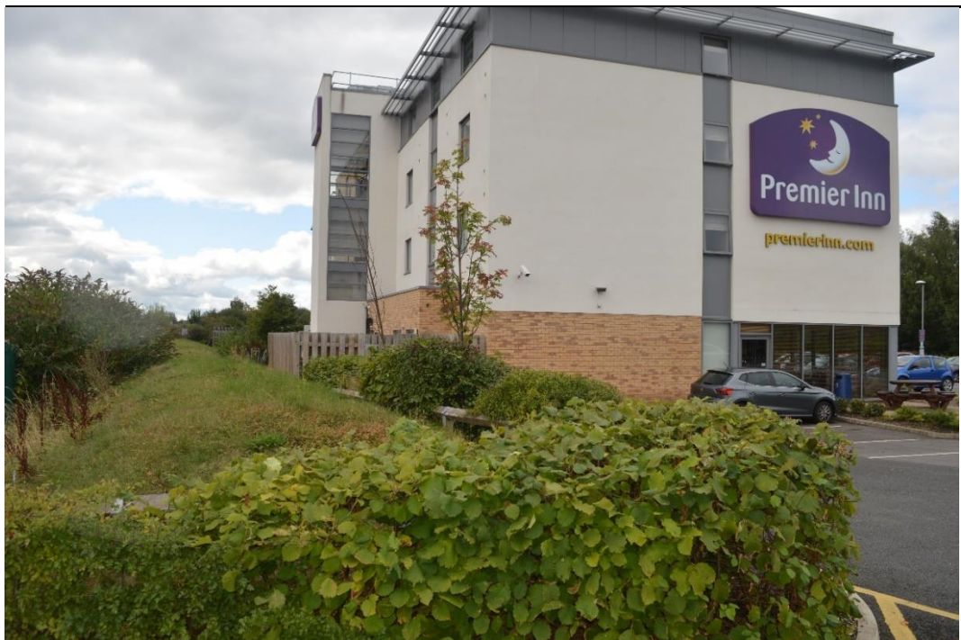
Fig. 8: The reconstructed section of the bank along the eastern side the Premier Inn, viewed from the north.
