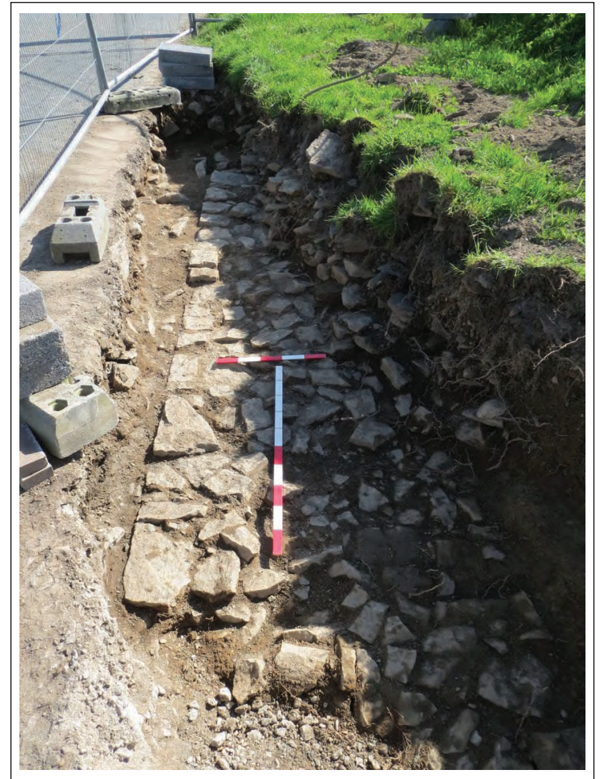
Plate 12. Post-excitation shot of stone foundations (25) at the north-east corner of the site. Scales: 1 x 0.5m & 1 x 1m. Looking South.
