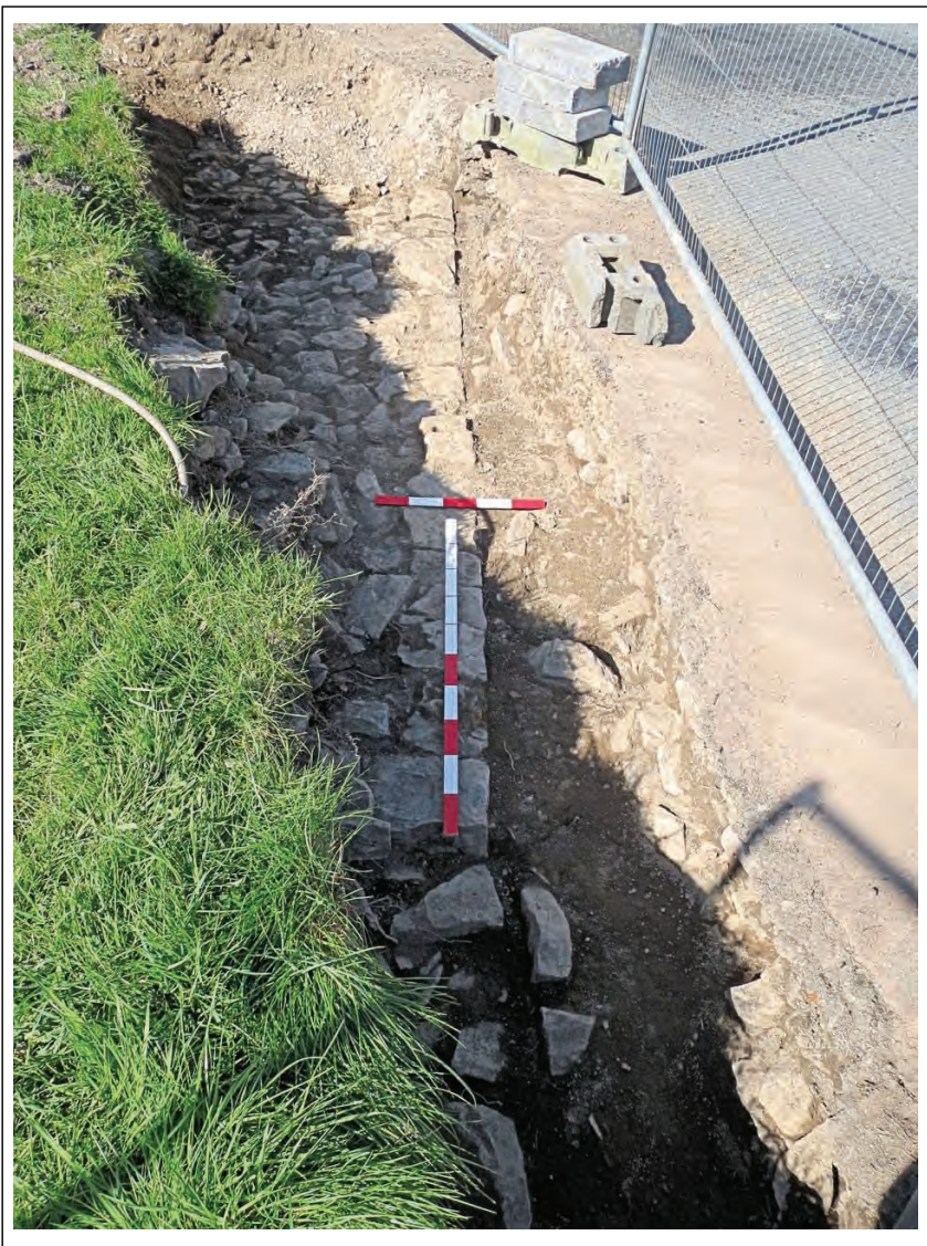
Plate 13. Post-excitation shot of stone foundations (25) at the north-east corner of the site. Scales: 1 x 0.5m & 1 x 1m. Looking North.
