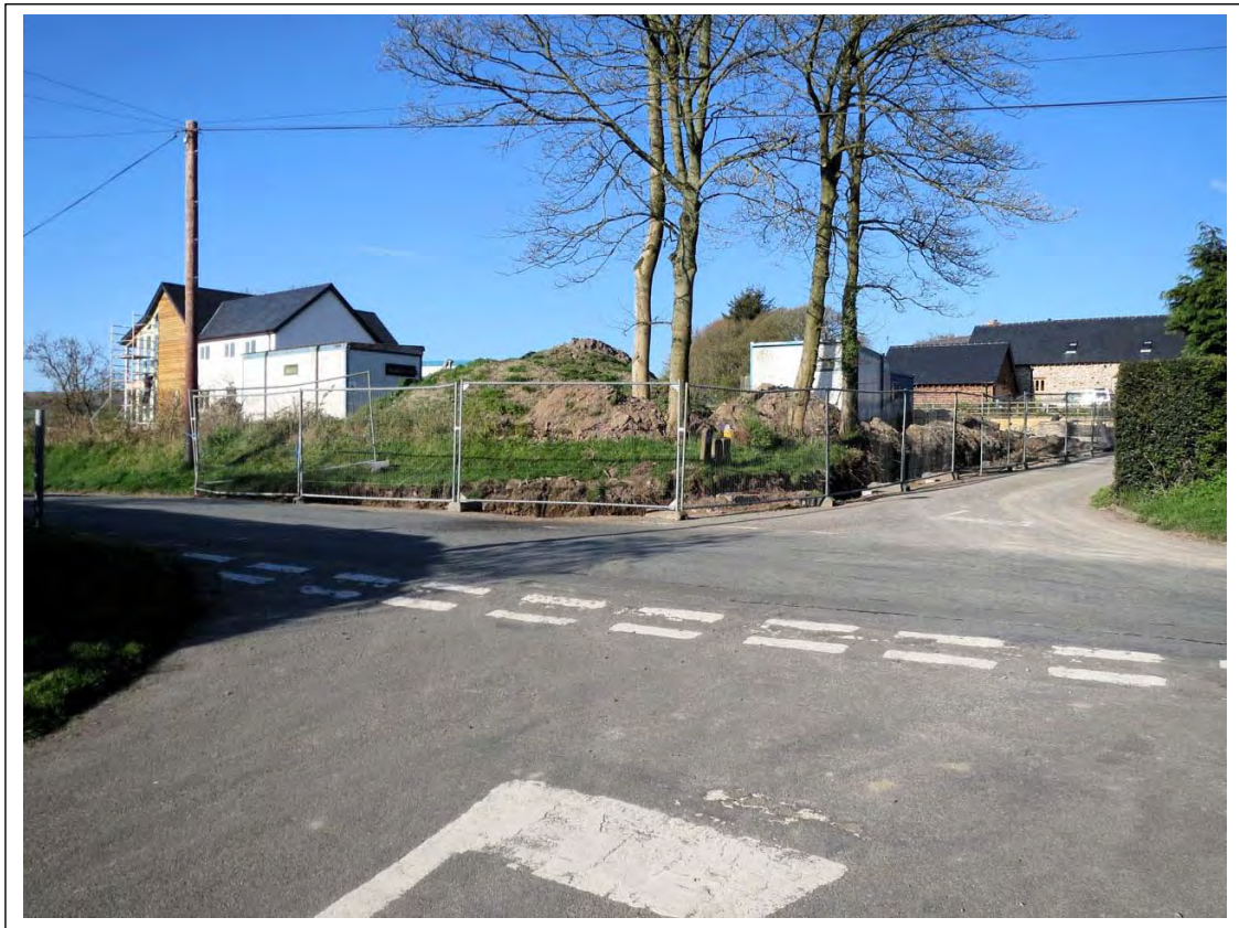
Plate 6. General view of the excavation area. Looking South-West.
