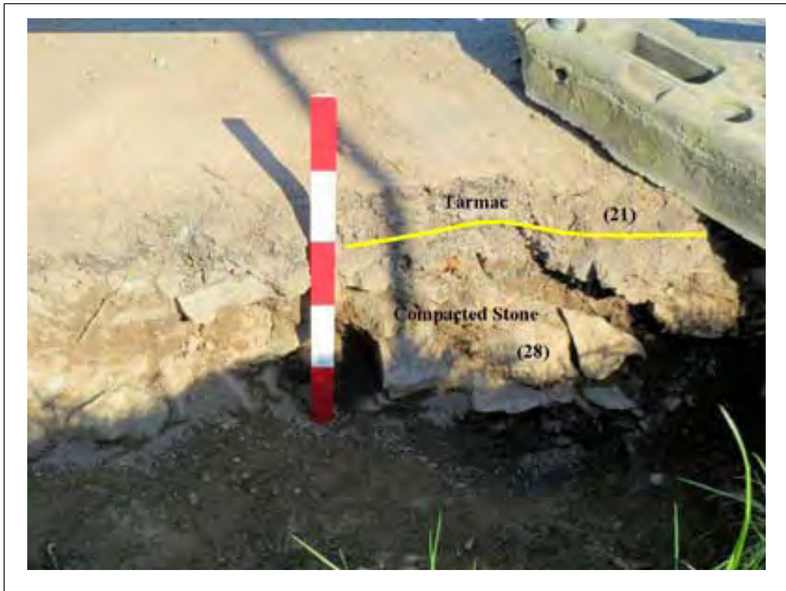
Plate 19. Sample Section 4 (facing west). Partly annotated photograph showing 5cm of tarmac (21) overlying 27-32cm of compacted stone (28). Scales: 1 x 0.5m. Looking East.
