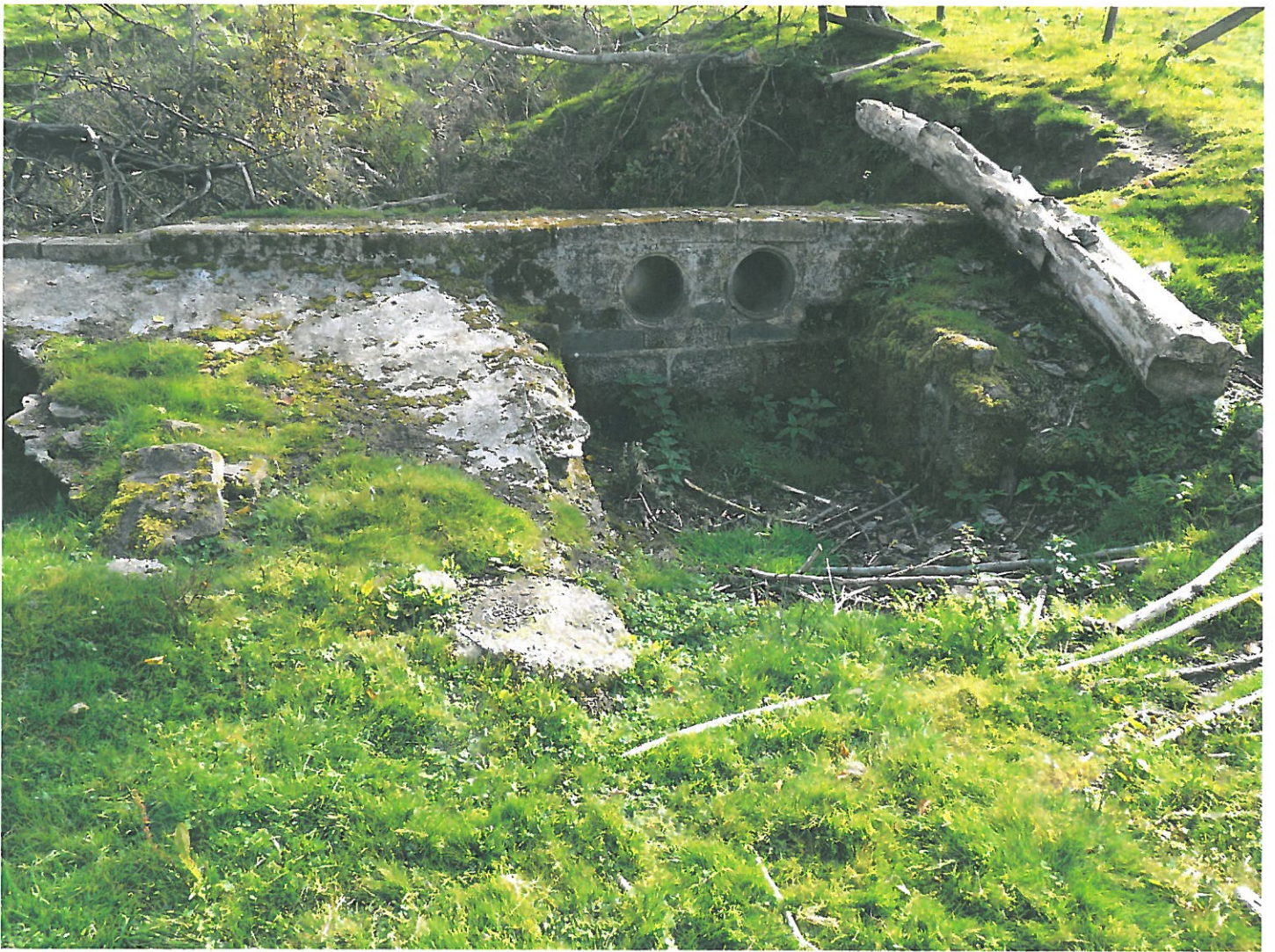
4530 Stanage Park Lake – Lake Overflow
