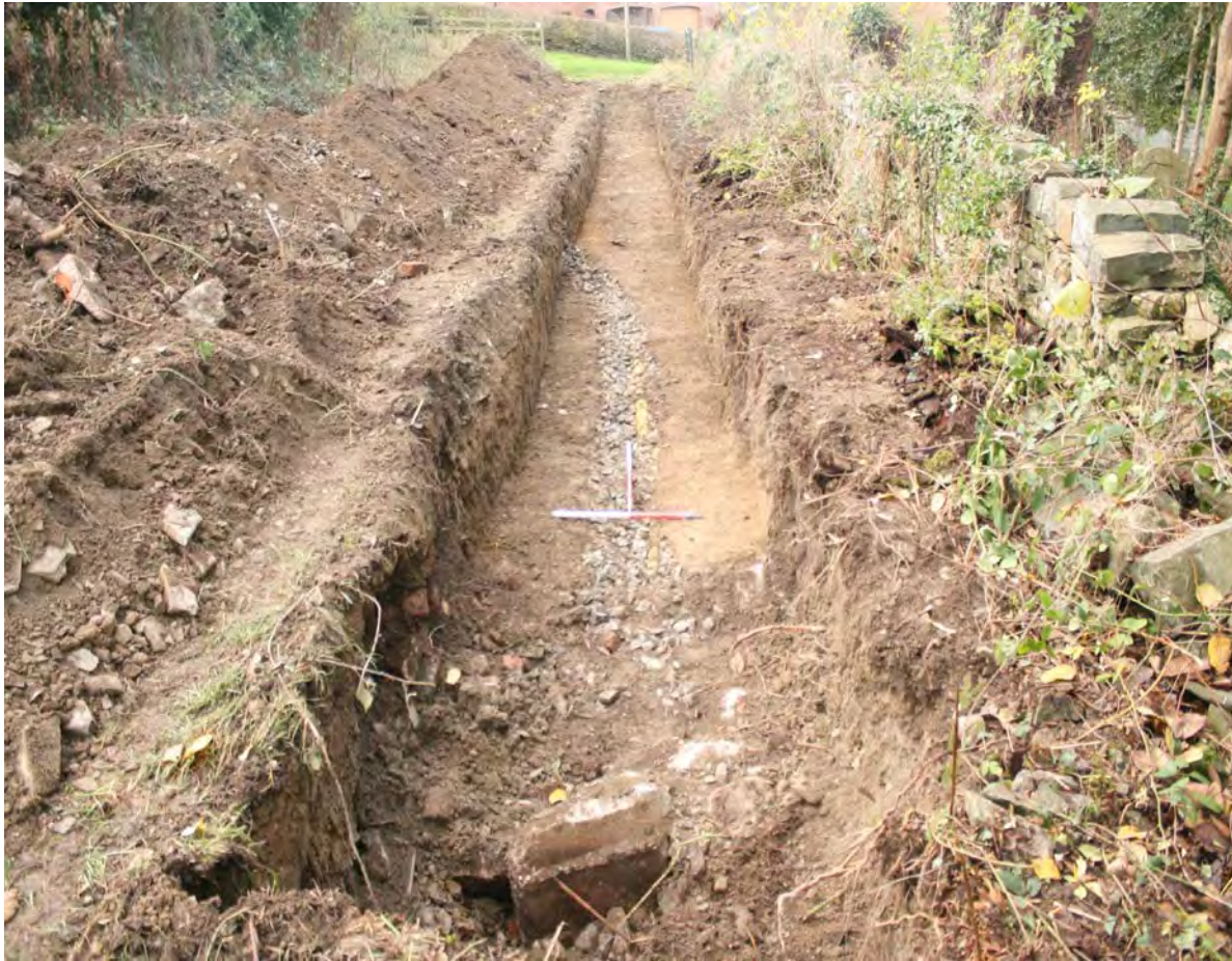
Trench 1: looking south-southwest and showing gravel filled pipe gully at north-eastern end
