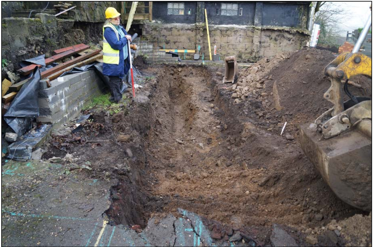
Plate 7: PBL2016_107: Excavation of southern foundation trench, through context 001 and into natural subsoil 005, looking west northwest.
