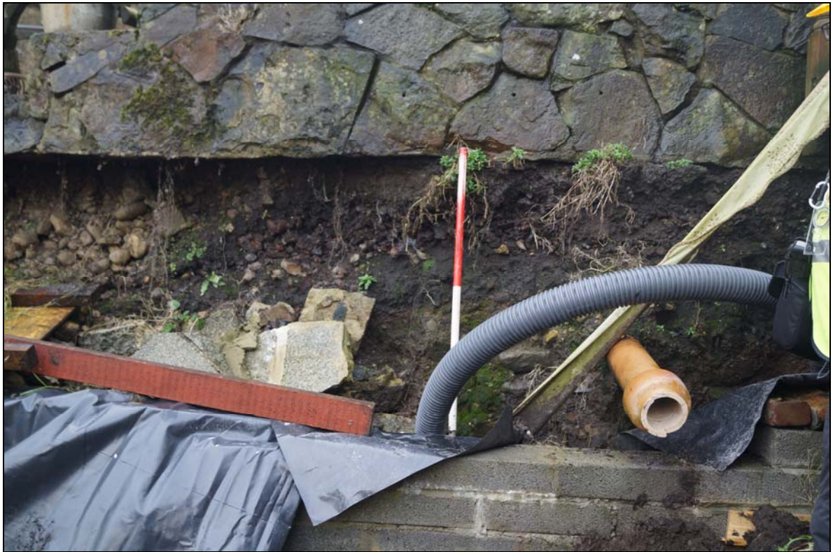
Plate 9: PBL2016_109: Section below steps showing the stone and concrete of the steps, 002, the cobble make up 003 below on the left of the photo and the former topsoil, 003 below that , looking south southwest.
