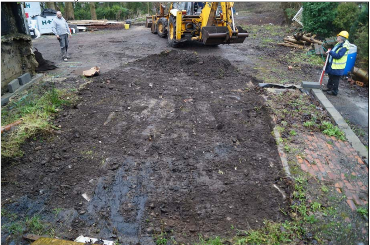
Plate 2: PBL2016_102: Surface vegetation and debris scraped off context 001, looking north northeast.
