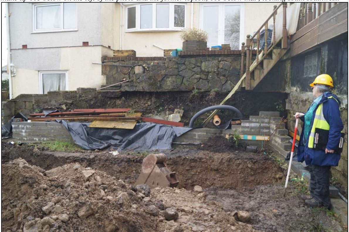
Plate10: PBL2016_110: The section below steps 002 showing 003 and 004, looking south southwest.
