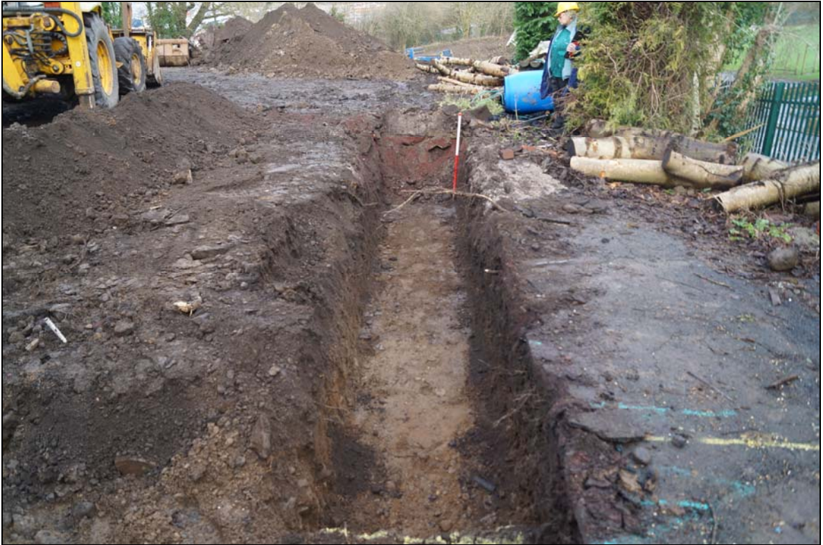
Plate 11: PBL2016_111: Eastern foundation trench, looking north northeast.
