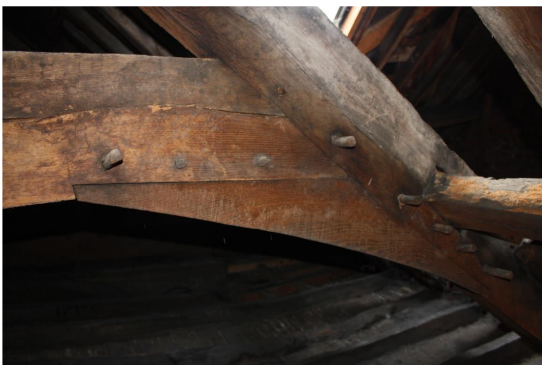
Fig.4. Cross-wing arched-brace. DS2013_386_023
