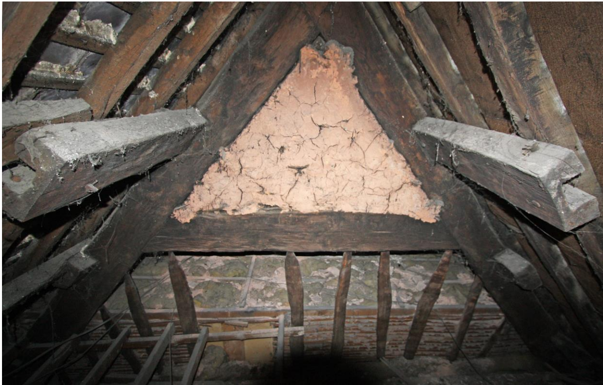
Fig. 9. Hall closed truss against cross-wing.
