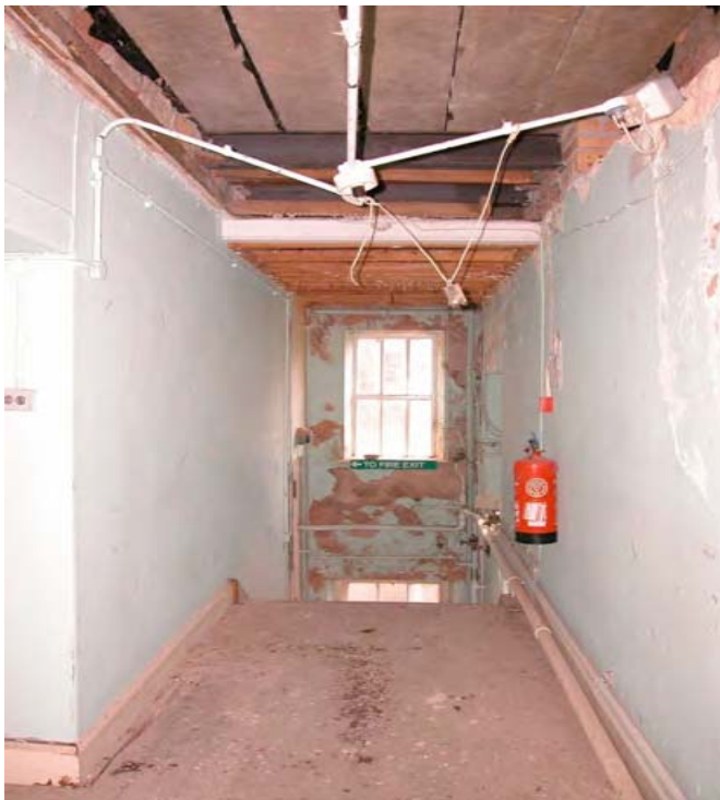
4.1.14 Second Floor Landing (S09)
