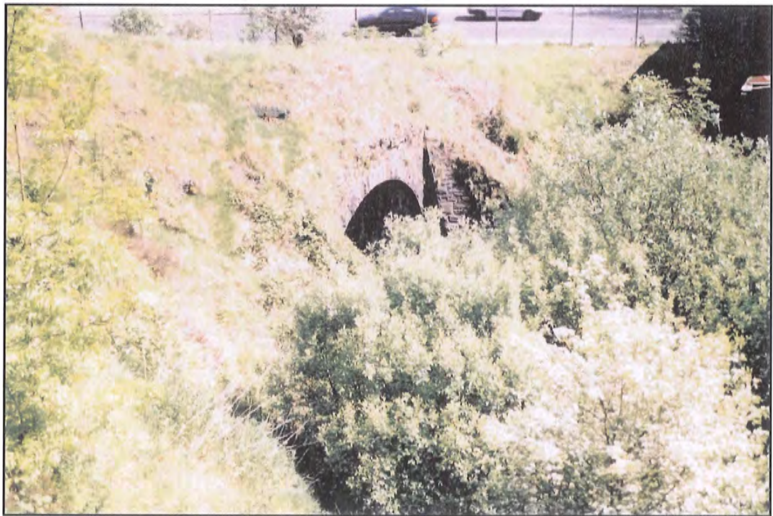
Plate 8 Southern end of Llynfi River culvert
