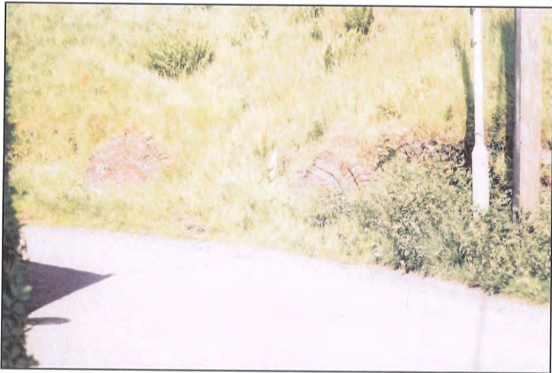
Plate 10 Brick arched features at Llynfi Road
