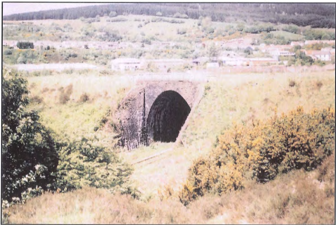
Plate 12 Bridge crossing Llynfi Valley Railway
