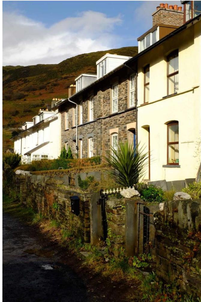
Fig 16 Numbers 13-24 Heol y Dwr / Water Street, showing the front garden walls with slate-slab gate piers and slate fences. Numbers 19-24 also have a sill band and pilaster strips.
