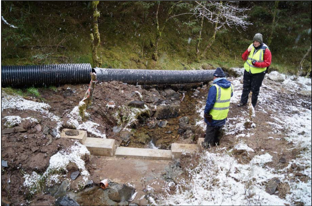
Plate 5: CNE2016_105, Hydro intake, looking northwest.
