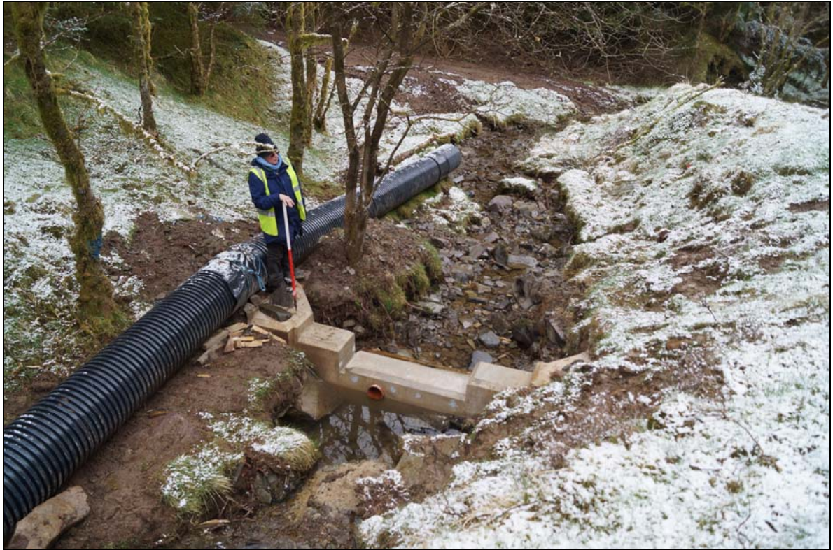
Plate 3: CNE2016_103, Hydro intake, looking northwest.
