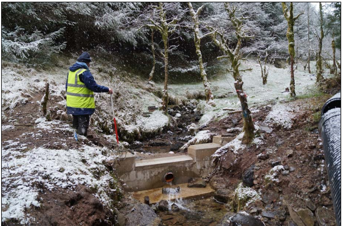
Plate 4: CNE2016_104, Hydro intake, looking south southeast.
