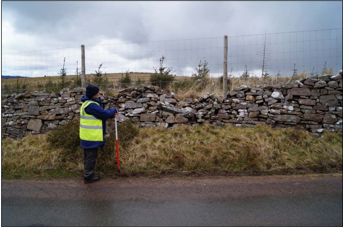
Plate 7: CNE2016_107, Boundary wall, looking north northwest.
