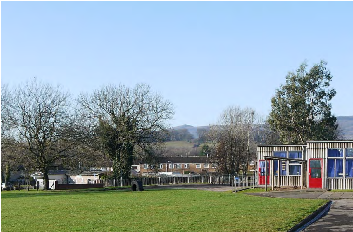
Photo 11: View from east side of building looking south west
