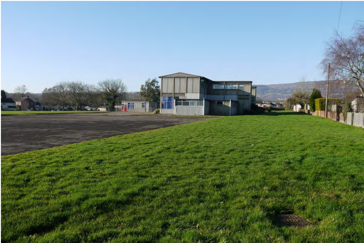
Photo 8: View from north east corner looking west
