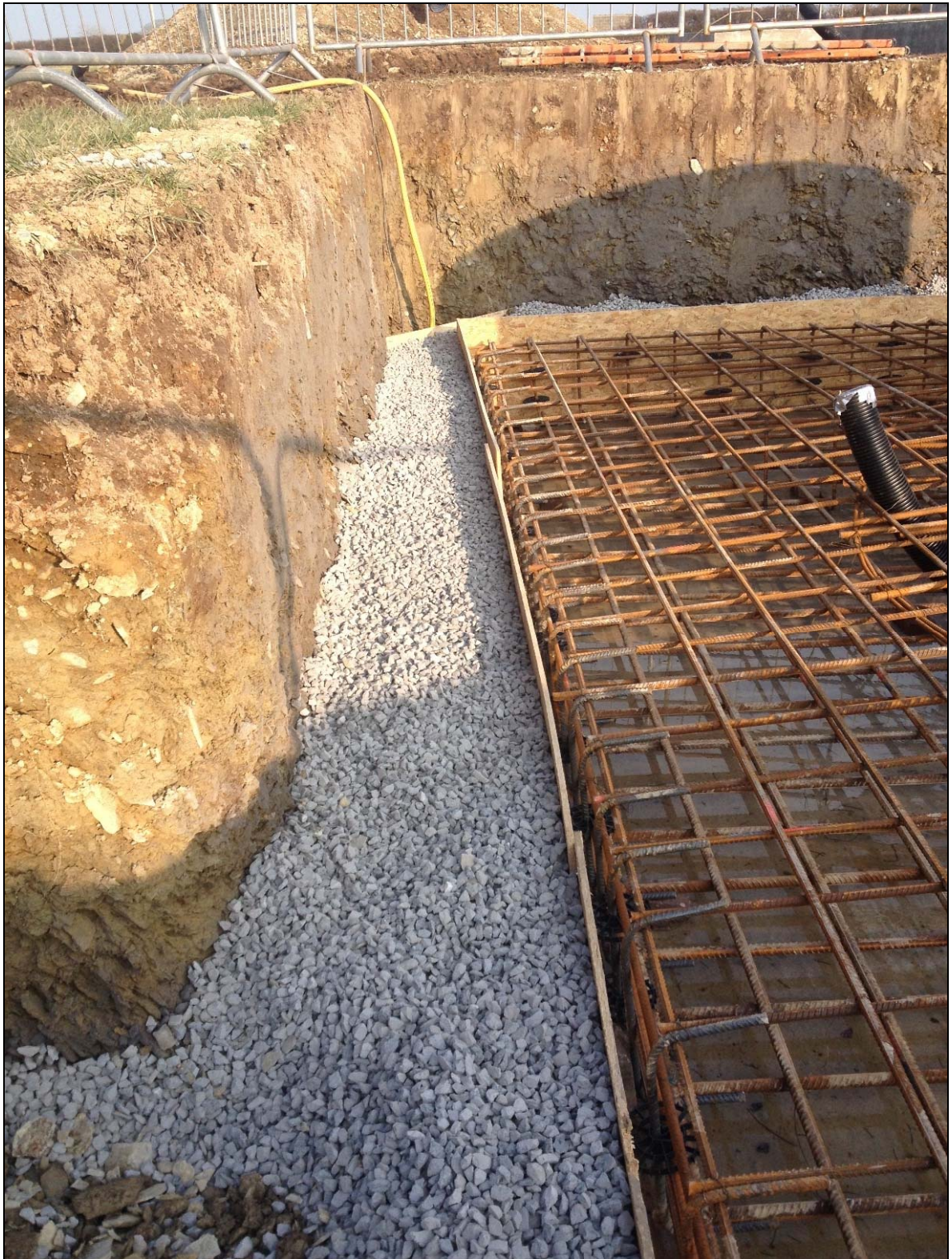
Plate 2: SAR2015_102, foundation hole, looking east.
