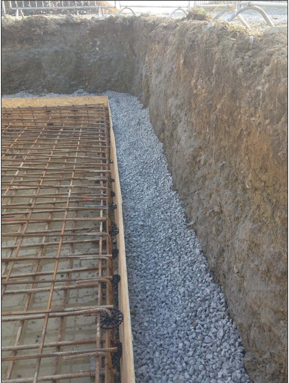
Plate 3: SAR2015_103, foundation hole, looking south.
