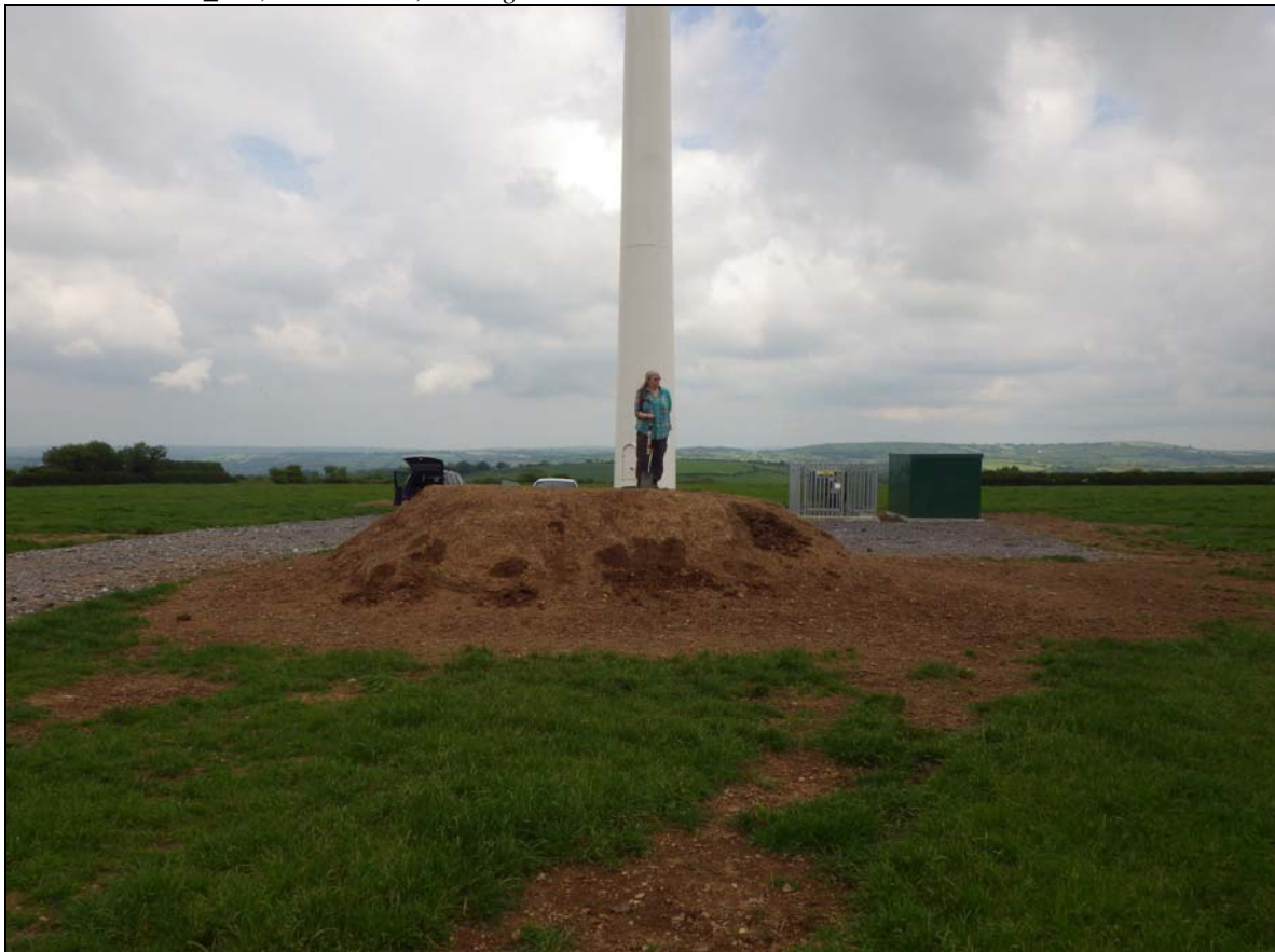
Plate 5: SAR2015_105, spoil heap, hardstanding, substation and turbine tower, looking north northwest.
