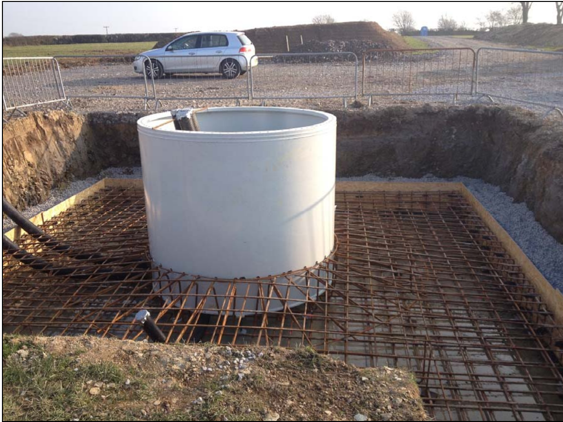
Plate 1: SAR2015_101, foundation hole, looking south.
