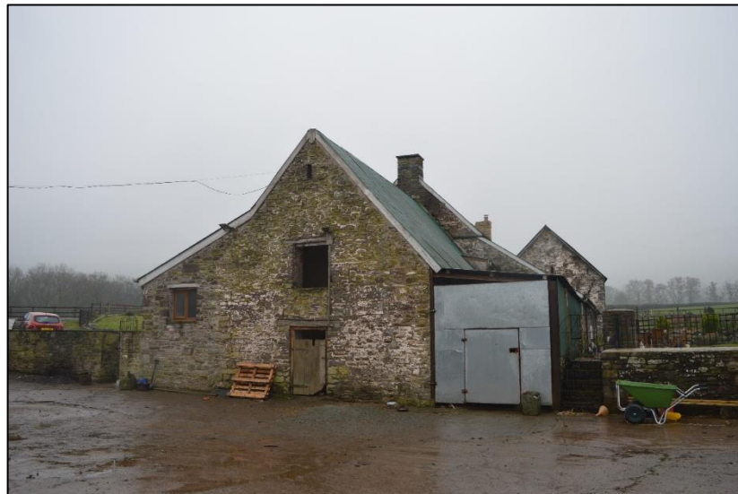
Fig. 10 View from the north showing the relative difference in roof pitch between the byre (in the foreground) and house behind it. Photo CPAT 4635-0026
