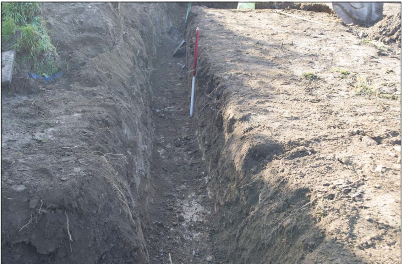
Plate 04: Electricity cable trench; scale: 1x1m (archive reference: G2629_014).
