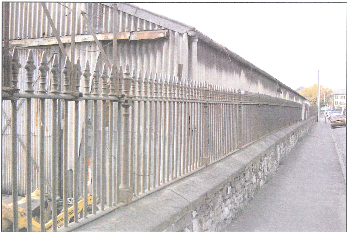
Plate 4 The cast-iron railings between the Cattle Market and Ruperra Street
