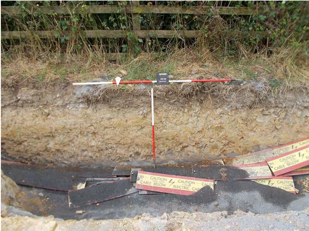
Photo 3: Looking south at a section of cable trench showing deposits 109 and 110 (Section 1). 2m & 1m scale.
