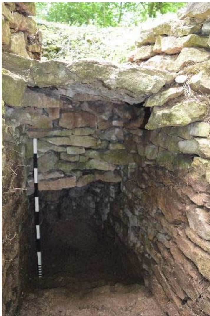
Fig 9. The channel after excavation, with a paving slab in place above.
