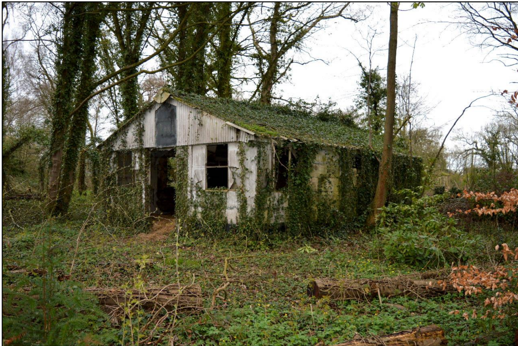
Fig. 13 The intact ward (Building 4), from the north-east. Photo CPAT 4486-0052
