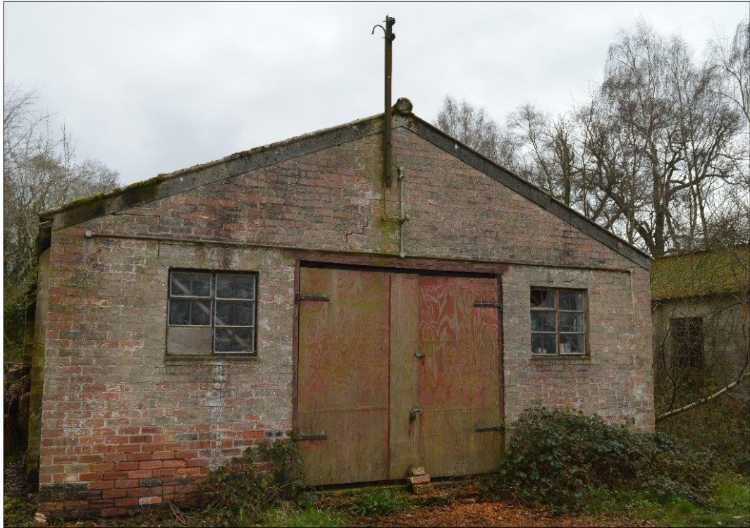
Fig. 7 West elevation of Building 1. Photo CPAT 4486-0085
