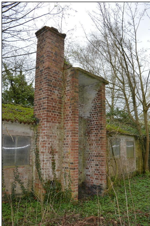
Fig. 12 The chimney stack and water tank support, viewed from the south. Photo CPAT 4486-0066
