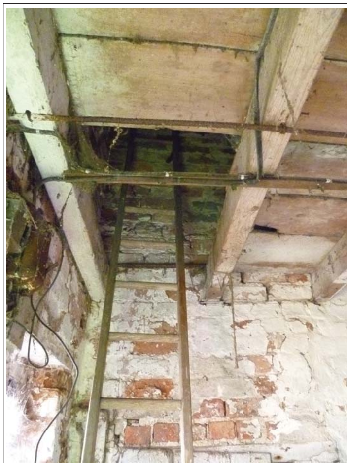
Plate 12. Hatch to barn loft.
