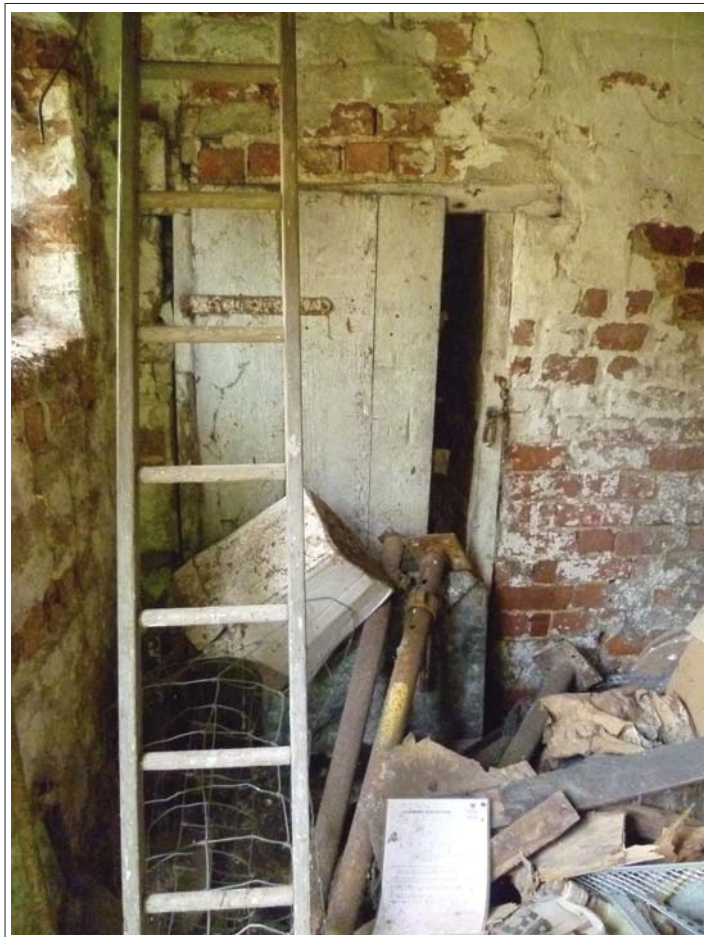
Plate 11. Interior of adjacent barn.
