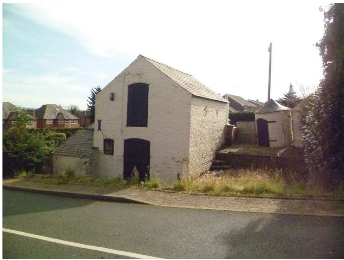
Plate 5. The Privies viewed from the north-west, 1m scale.
