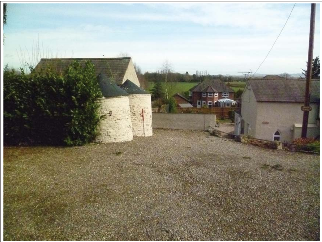
Plate 14. The Privies, view east, 1m scale.
