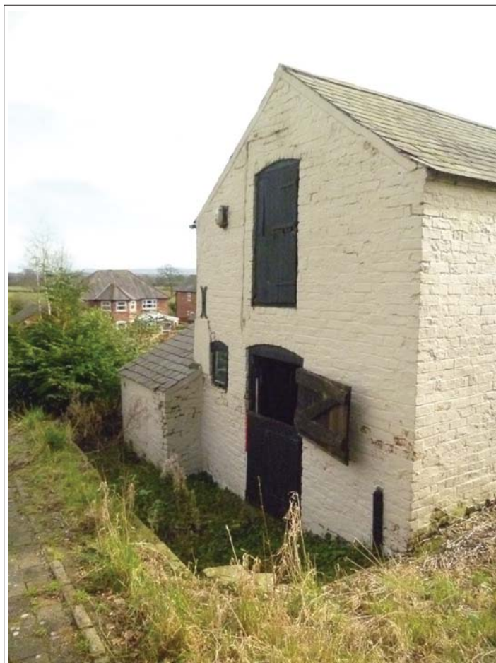
Plate 8. Detail of adjacent barn, view south-east.
