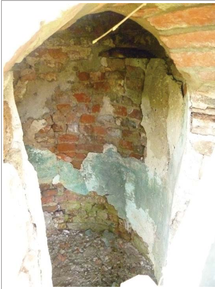
Plate 3. Interior view of the western most Privie, access limited.
