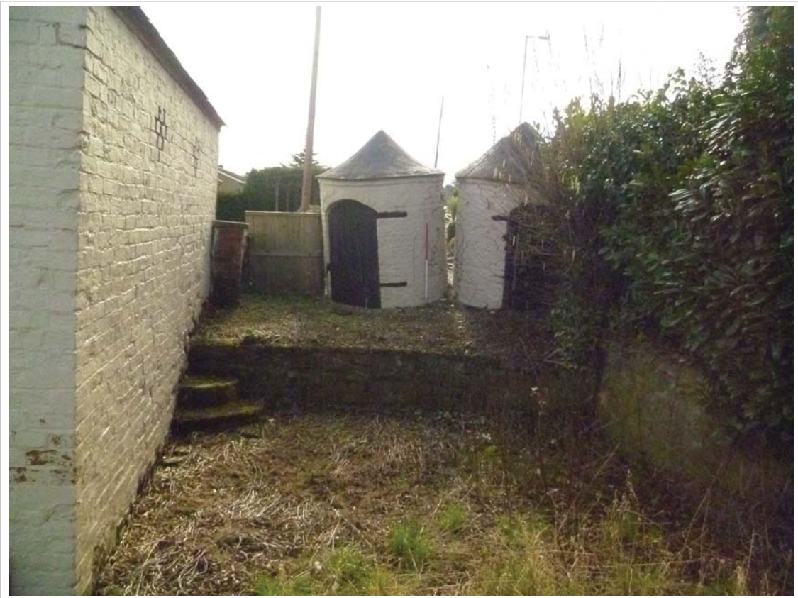
Plate 1. The Privies, view south. 1m scale.
