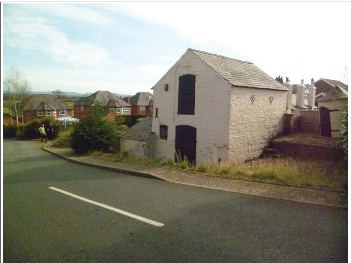
Plate 6. The Privies' setting viewed from the north-west.
