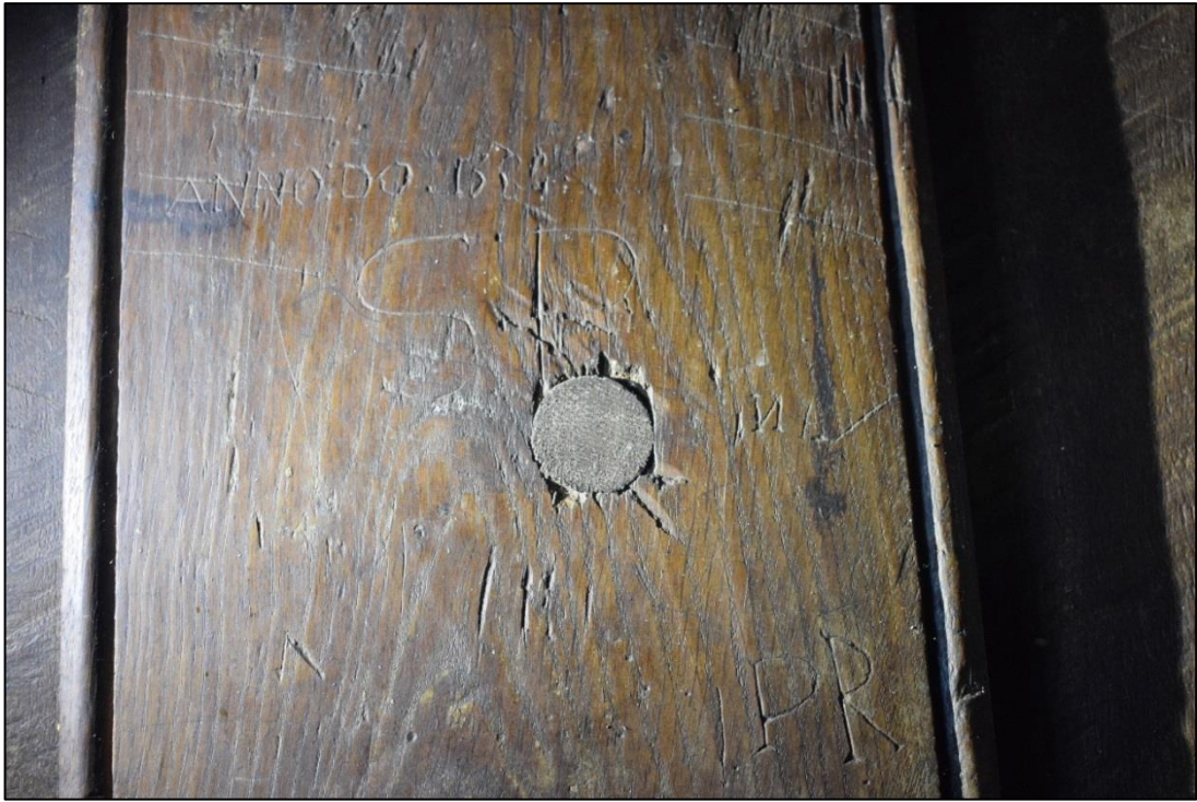
Fig. 9: The incised date of 1586 on one of the posts in the partition, also showing the three sets of initials, the decorative grooves on the vertical edges of the post and the assembly marks. CPAT 4599-0039
