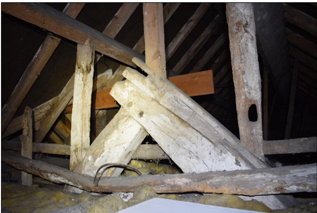
Fig. 11: The apex of the roof truss in the loft space. CPAT 4599-0028
