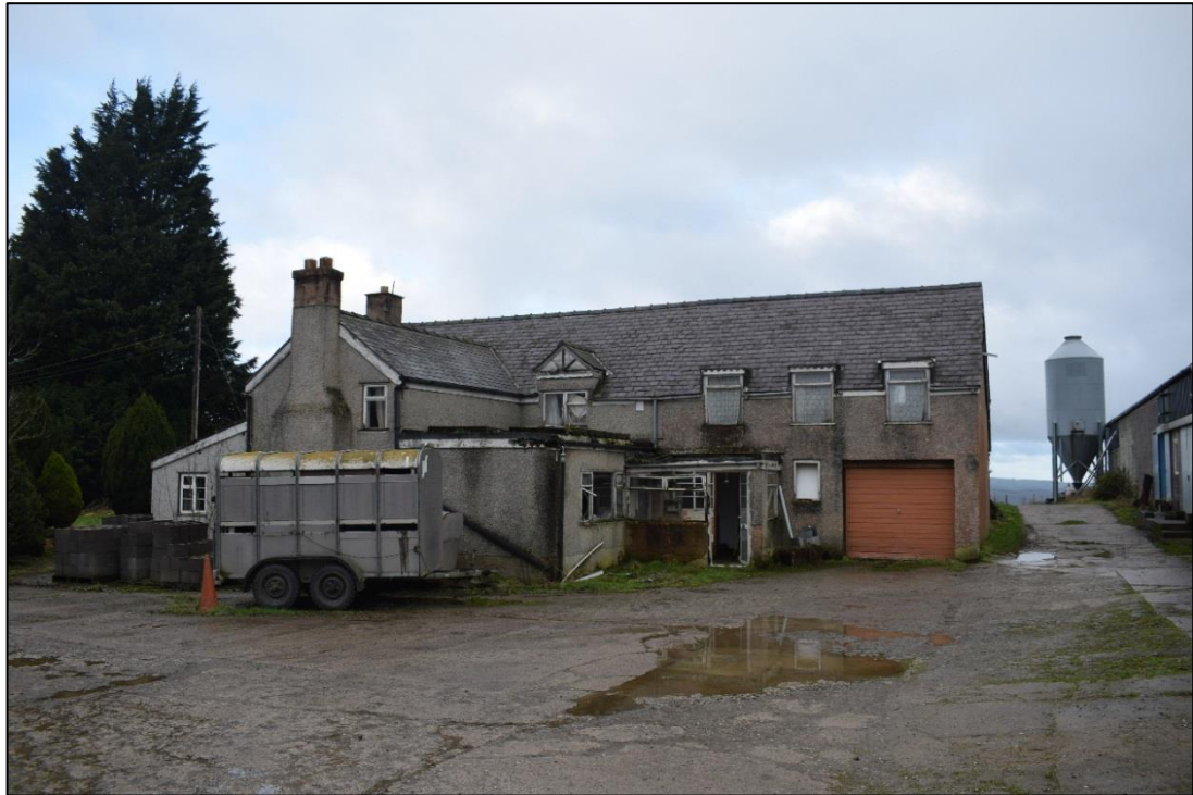
Fig. 5: General view of Llidiart Fawr from east, showing the pebble-dash covering and later piecemeal additions. The north-east end of the original house is identified by a gutter downpipe to the left of the three modern dormer-type windows. CPAT 4599-0008
