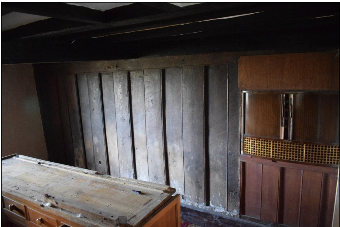
Fig. 7: The post-and-panel partition on the ground floor. CPAT 4599-0030
