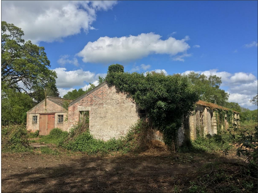
Fig. 8 Buildings 1 and 2, viewed from the south-west. Photo K. Barker.
