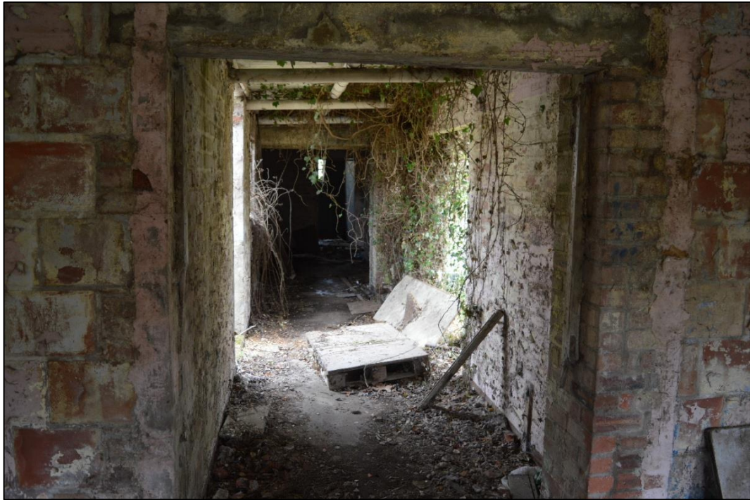
Fig. 10 The covered access way between Buildings 1 and 2, from the south. Photo CPAT 4486-0097
