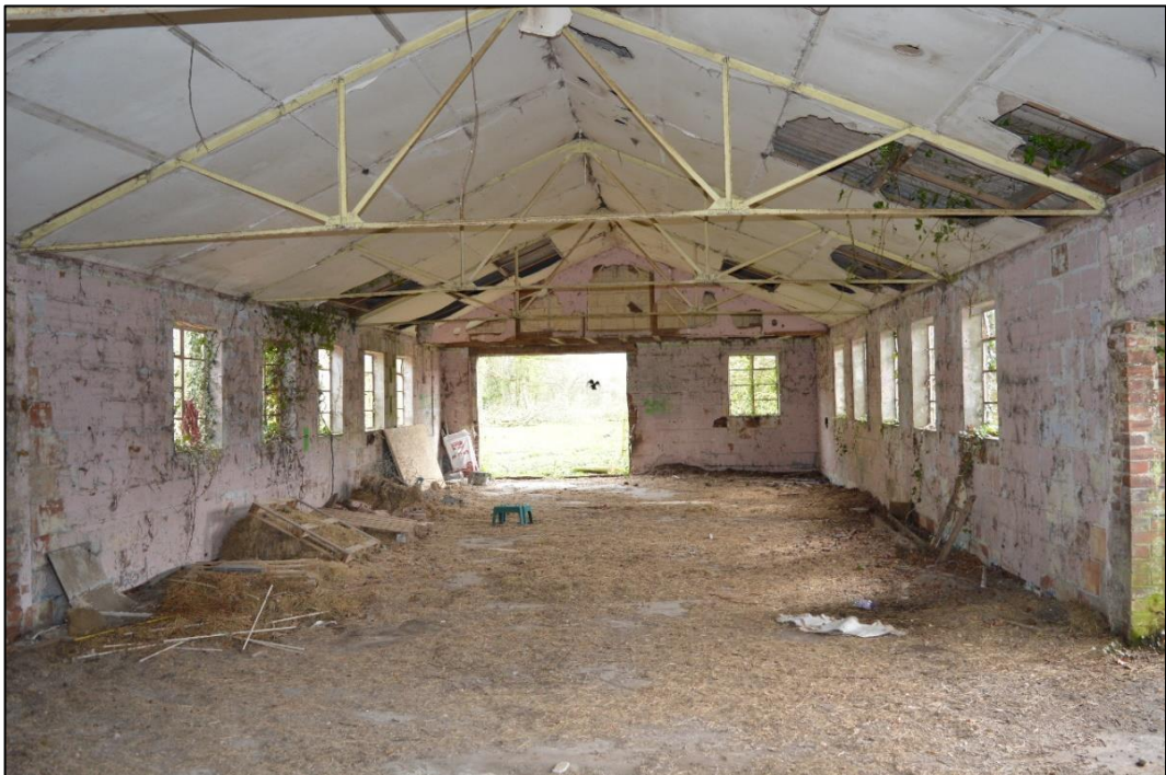
Fig. 9 The interior of Building 2, viewed from the west. Photo CPAT 4486-0095
