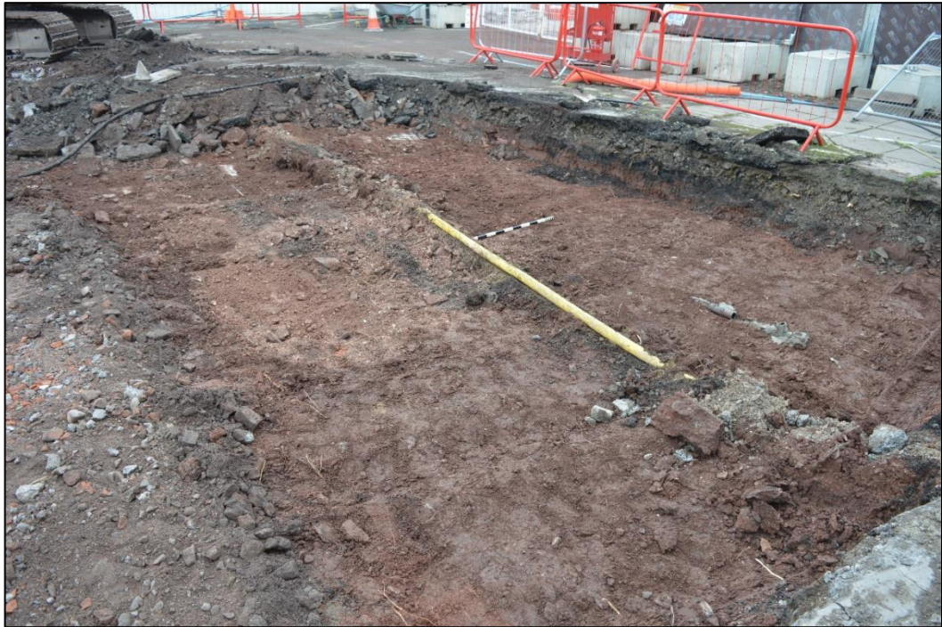
Fig. 7 View from the south-east of Area 2. Photo CPAT 4323-0011
