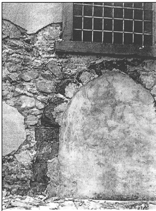
Fig. 2 Blocked doorway, west wall of the north nave, revealed during restoration in 2007. Photo G. Holland.
