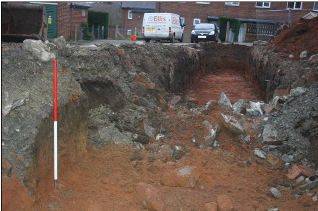
Fig. 2 The service trench (viewed from the street frontage), showing modern footings in the foreground. Photo CPAT 3747-0006
