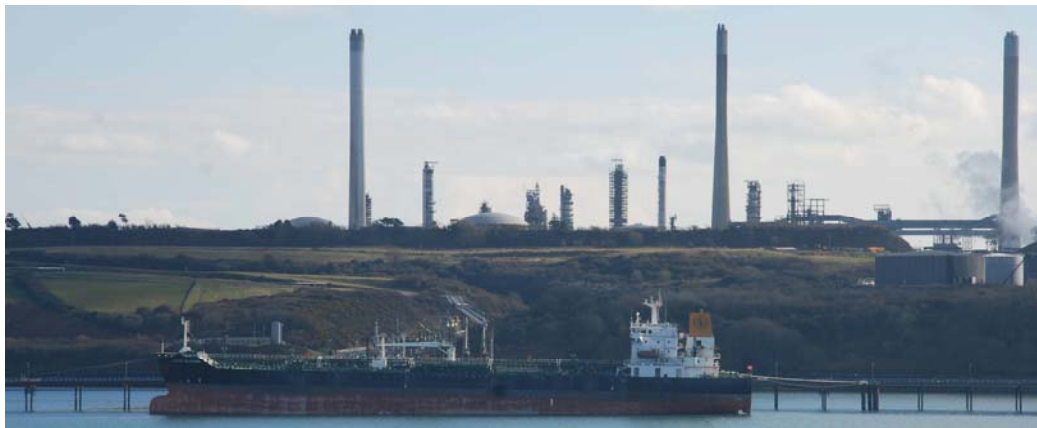
Milford Haven- refinery
