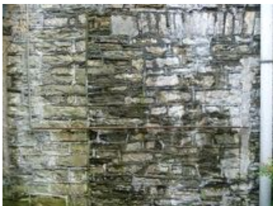
Figure 47 (left) and Figure 48 (right) above: old openings to north east wall at lower ground level – source Pembroke Design Ltd
