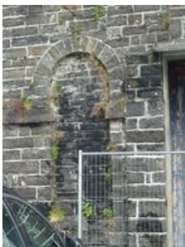
Figure 41 (left) and Figure 42 (right) above: Example of retained smaller blind panels and larger panels with windows inserted
