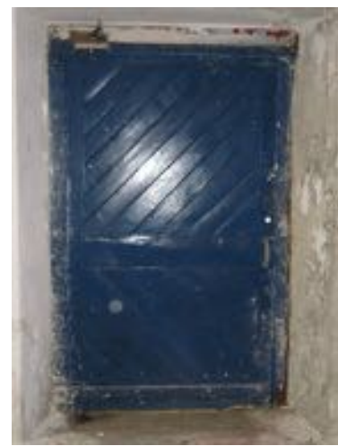
Figure 32 above: Door to north west elevation of market viewed internally with diagonal boarding
