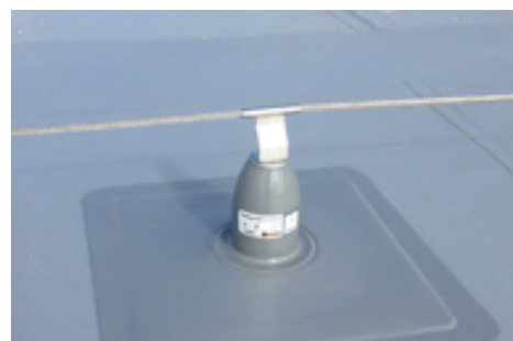
Figure 100 above: example of anchor point and cable within single ply roof finish
