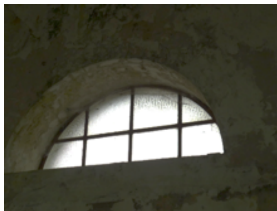
Figure 39 (left) and Figure 40 (right) above: typical arched metal window inserted into north west and south west elevations
