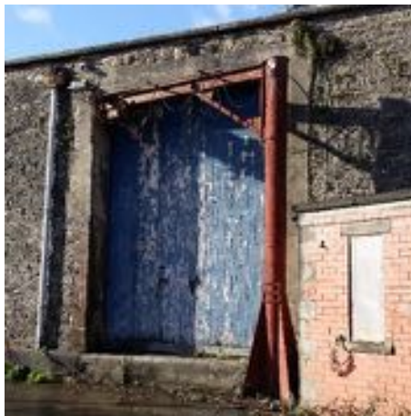
Figure 37 above: Hoist from iron foundry - – source Pembroke Design Ltd
